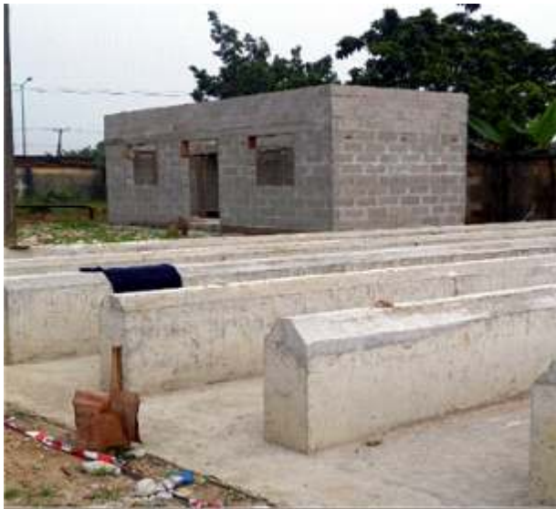
Ongoing construction of pump house and Ground Tank Foundation at Bori
