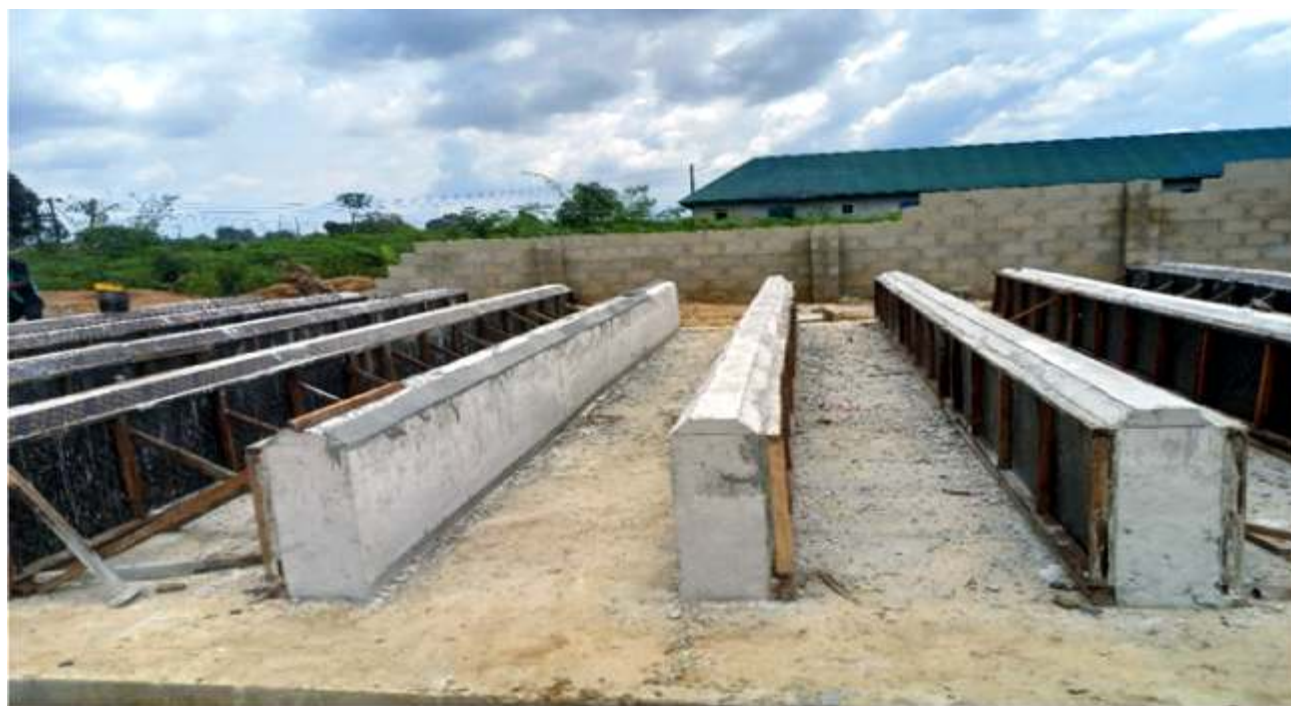
GRAND TANK FOUNDATION AT B- DERE
