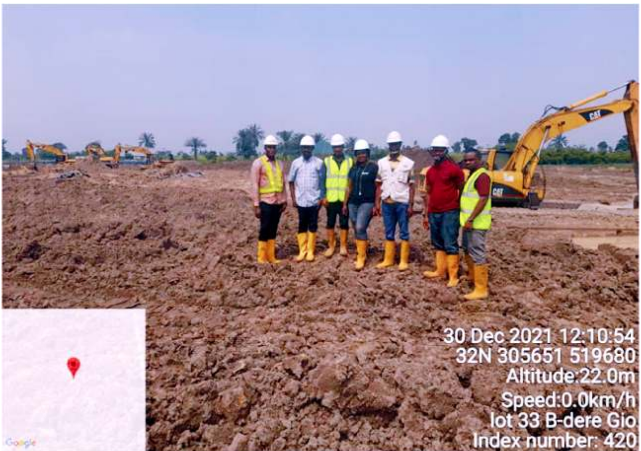
Plate 1.4: Backfilling of excavated pits with treated soil nearing completion at Lot 033 B.Dere / Gio, Gokana / Tai L.G.A. Remediation Contractor - CHRISTOHOUSTON ENERGY LTD
