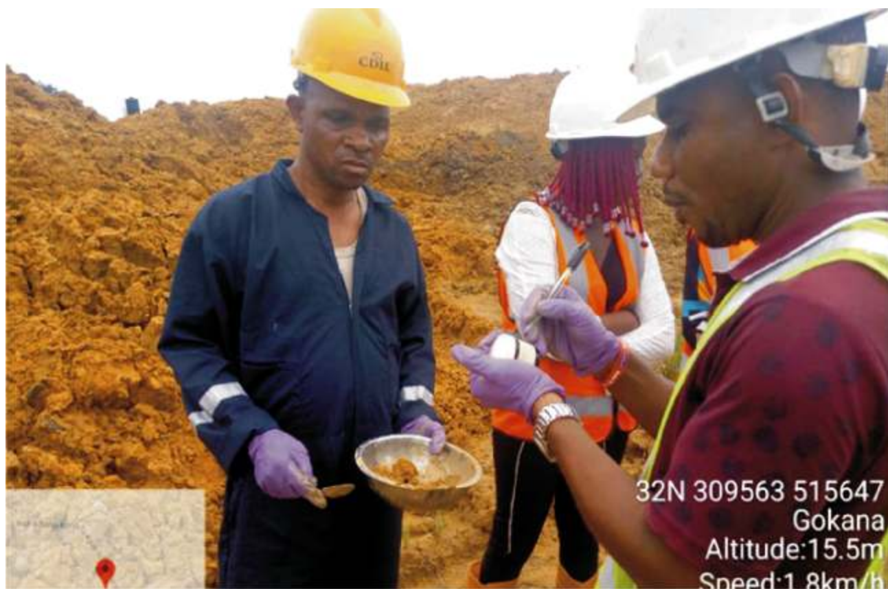
Plate 1.5: Quality Assurance / Quality Control (QA/QC) and Remediation Execution Officers from the Operations Unit of HYPREP collecting final lapse of QAQC Monitoring Samples from treated soil volumes with the Contractor representatives at Lot 013 Nweekol Zorbuke – K. Dere, Gokana L.G.A). Remediation Contractor -CENTENNIAL DEVELOPMENT & INVESTMENT LTD.
