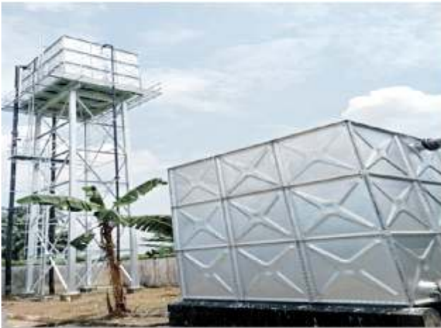
Rehabilitated surface and overhead Tanks at Agbonchia Booster Station
