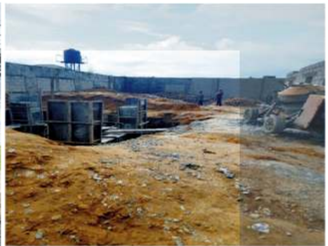
Overhead and Ground Tanks Foundation works at Biara
