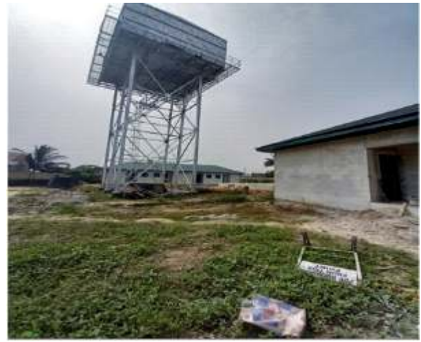
Rehabilitated Ogale Booster Station
