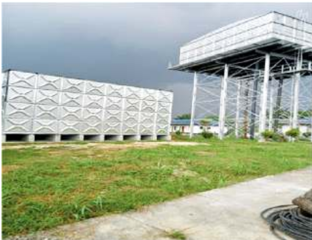
Completed Surface and Overhead Tanks at Terabo
