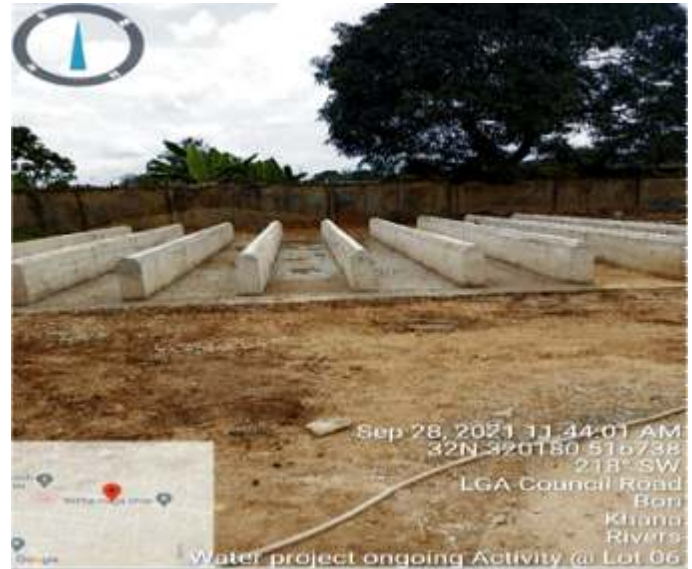
Ongoing construction of pump house and Ground Tank Foundation at Bori
