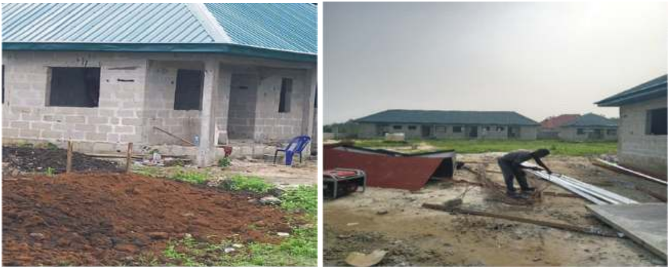
Staff Quarters construction works at Korokoro and Nonwa sites ongoing
