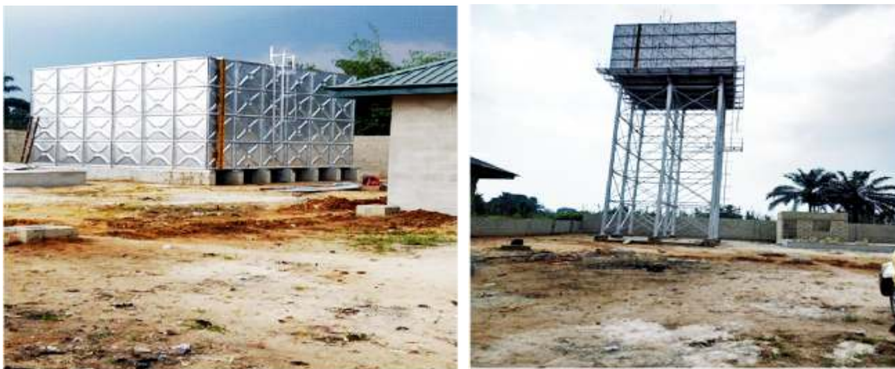
Constructed and installed Overhead and Ground Tanks at Barako
