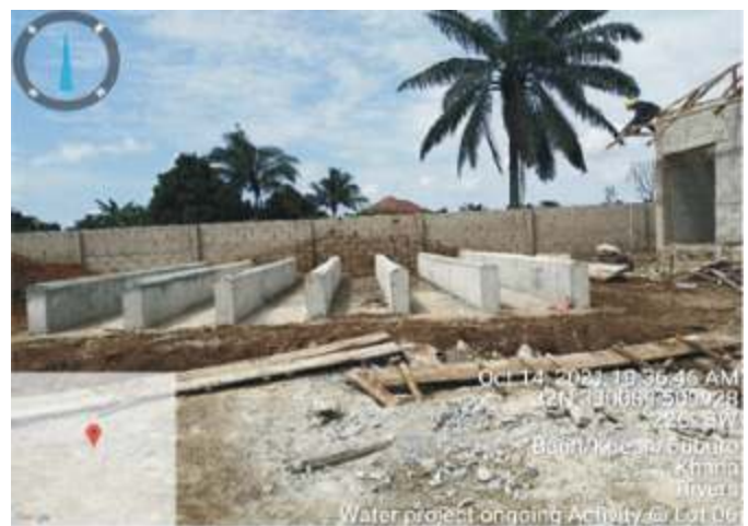
Construction of Treatment House and Ground water Tank at Kpean ongoing
