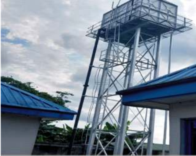
Constructed and installed Overhead tank at Ebubu
