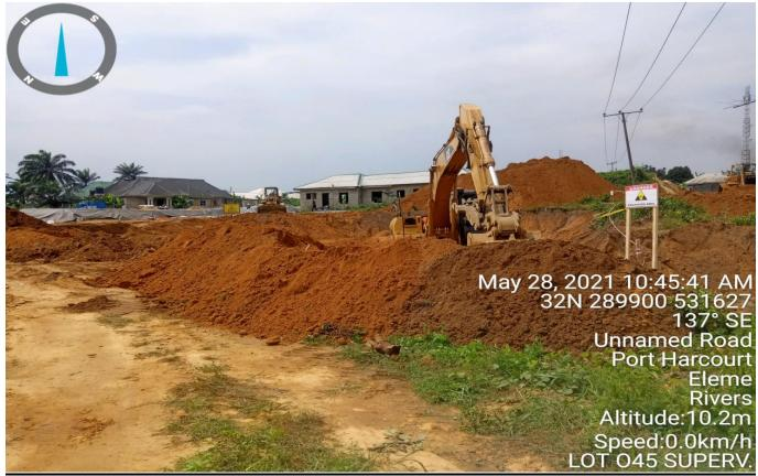
Plate 4: Commencement of excavation of impacted soil from delineated impacted area for treatment at Lot 045 (Aleto –Ngofa in Eleme L.G.A). (Remediation Contractor = Chavyn Nig. Ltd).
