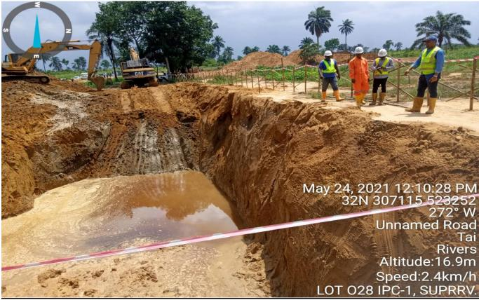
Plate 3: Commencement of excavation of impacted soil from delineated impacted area for treatment at Lot 028 (Bara Alue in Tai L.G.A). (Remediation Contractor = Emamed Nig. Ltd).
