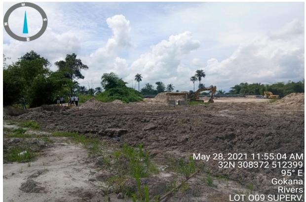
Plate 1: Final stage of backfilling of excavated pit with treated soil at Lot 009 (Saanako) in Mogho, Gokana L.G.A. (Contractor: Odun Environmental Ltd). The four (4) other Phase 1 Batch 1 Remediation Lots (Lot 011 and 012 at Debon-
