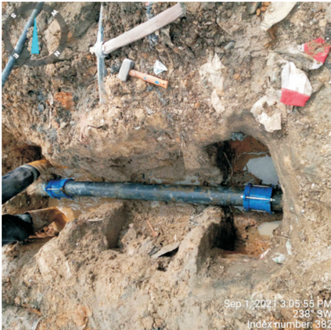
Laying of pipes at Ogale
