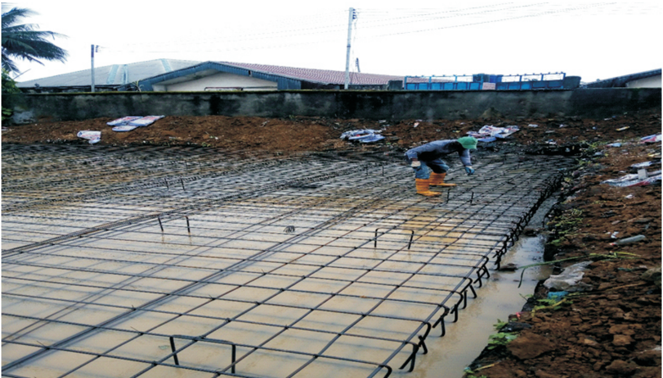
GROUND TANK FOUNDATION WORKS AT EBUBU
