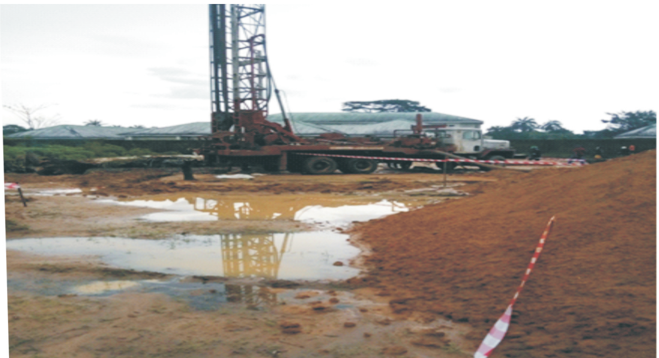
Construction of Foundation for Overhead Tank Drilling of borehole 2
