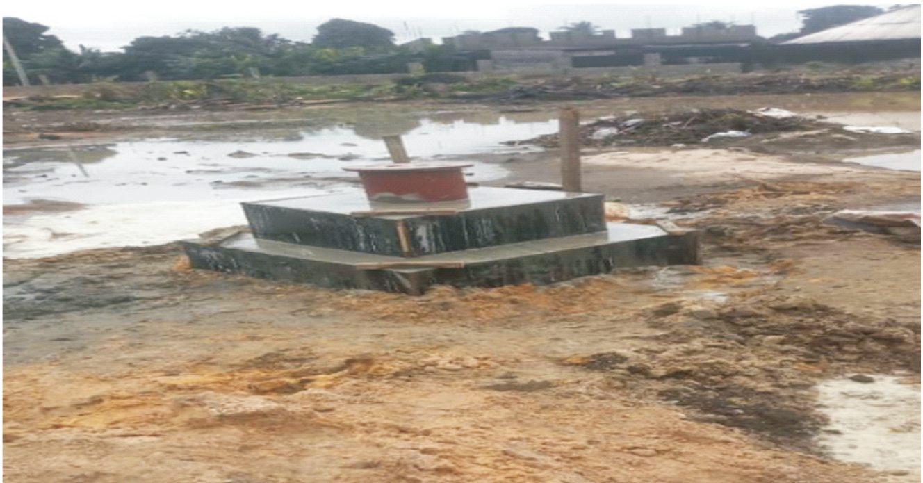
One of the Completed Borehole at Nonwa
