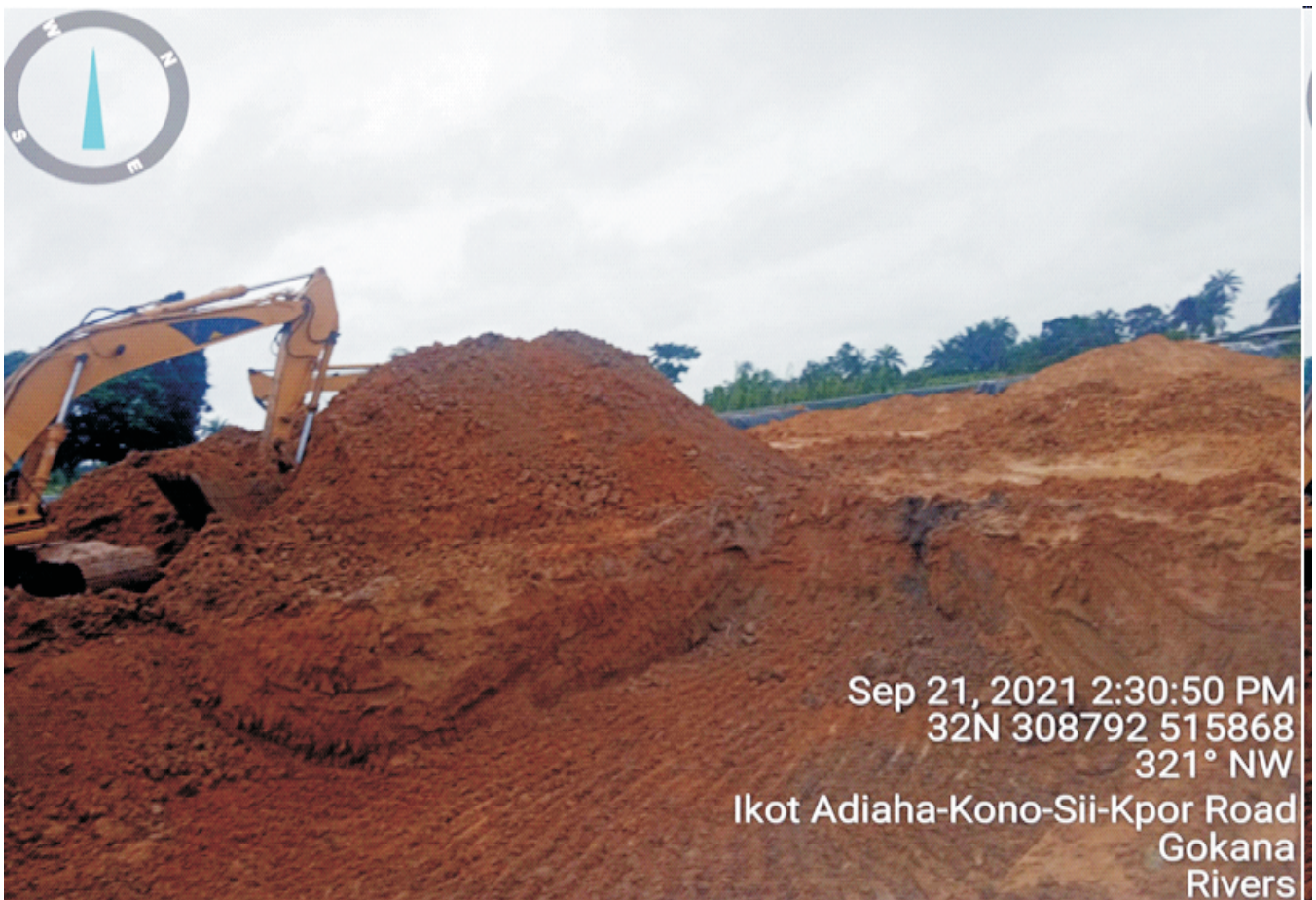
Plate 1.1: Concluding stage of excavation of impacted soil for treatment in progress at Lot 013 (Nweekol Zorbuke in K. Dere, Gokana L.G.A). (Remediation Contractor - CENTENNIAL DEVELOPMENT & INVESTMENT LTD).
