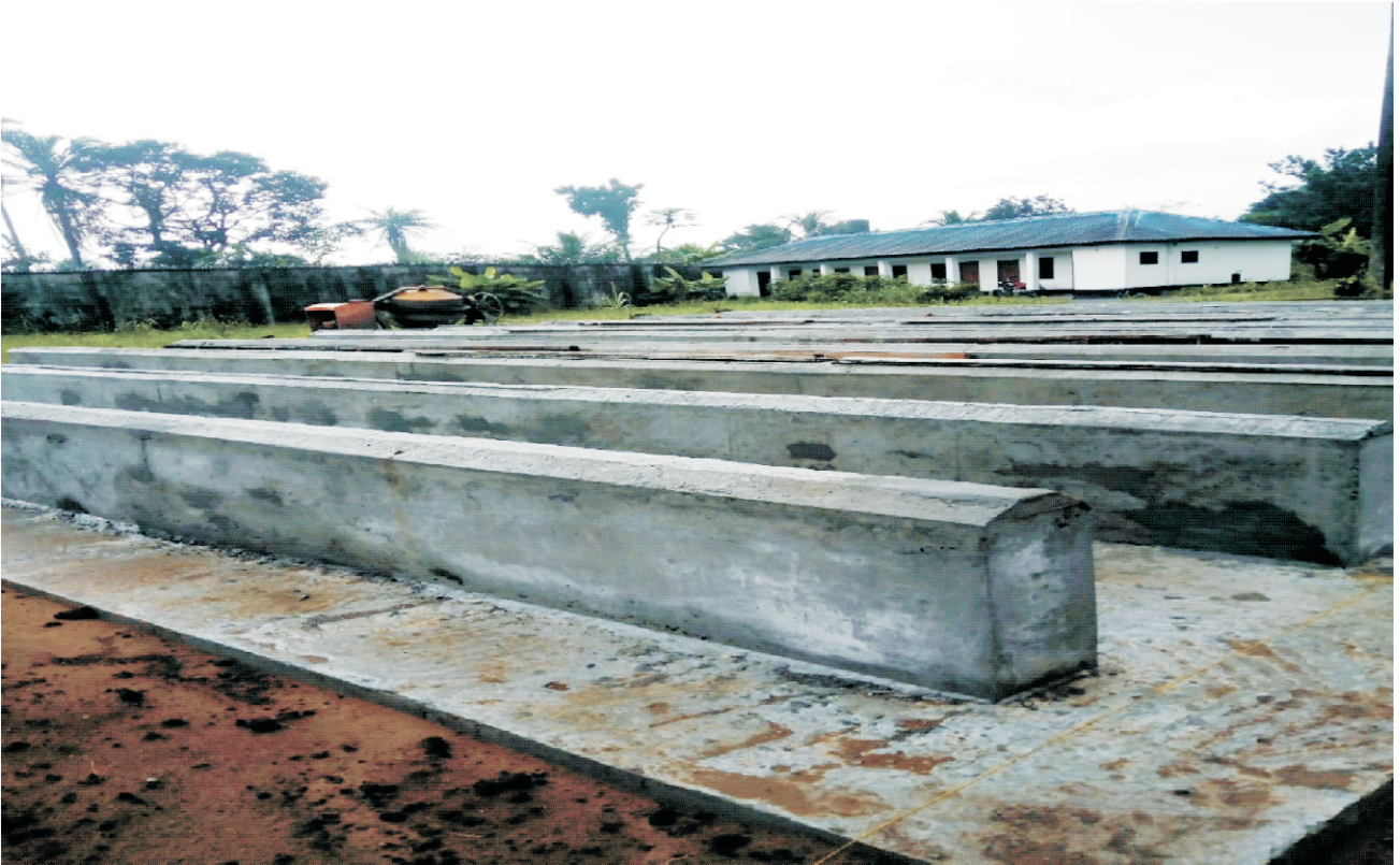
GROUNDTANK FOUNDATION AT TERRABO
