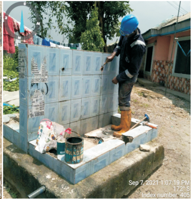
Servicing of water fetching point at Alode
