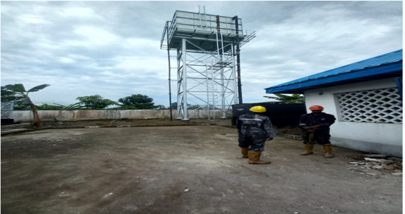
Replaced brazing of vandalized overhead tank at Alesa Booster station
