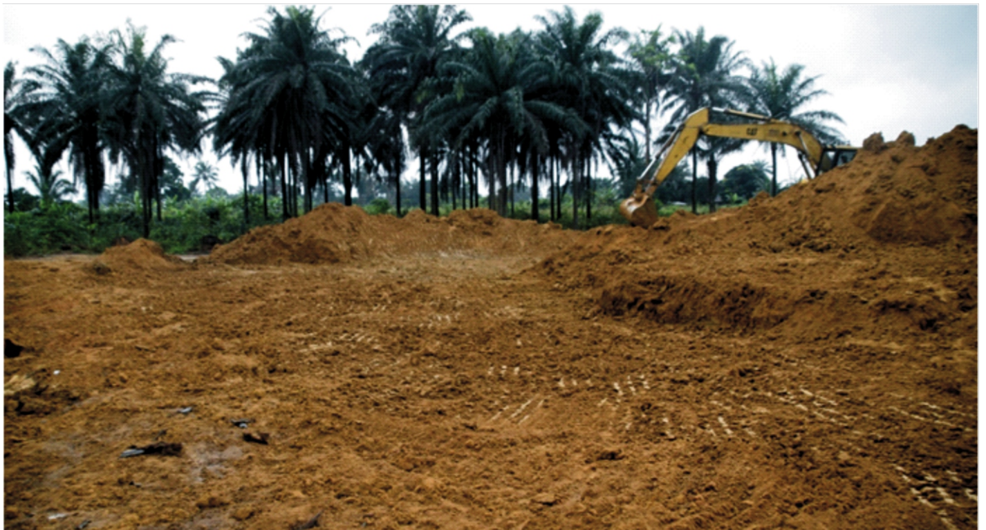
Plate 1.4: Final stage of backfilling, site leveling and landscaping in progress at Lot 029 (Bara Alue, Tai L.G.A) as at 3rd March, 2022. Remediation Contractor -WEAFRI WELLS SERVICES LTD.
