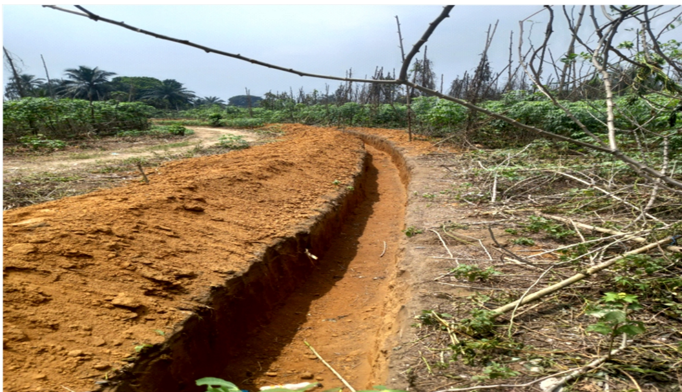
Excavations of trench for pipe laying at Barako.
