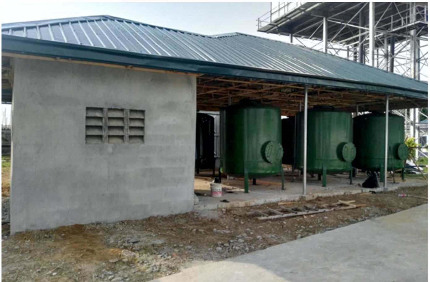
INSTALLATION OF PRESSURE FILTER AT TERABO.
