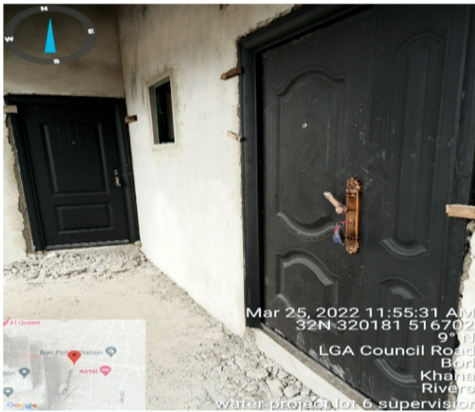
INSTALLATION OF DOORS ON BORI TREATMENT HOUSE.
