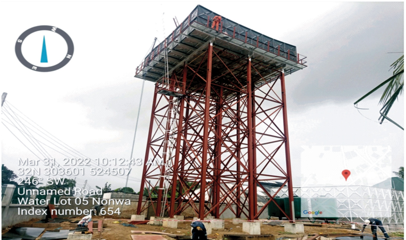
CONSTRUCTION OF OVERHEAD TANK AT NONWA.
