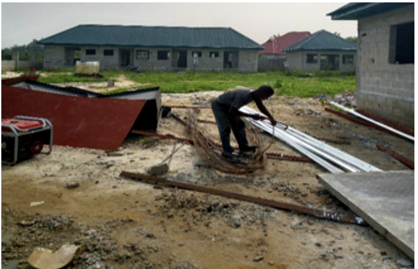
Staff Quarters/Treatment House at Korokoro.
