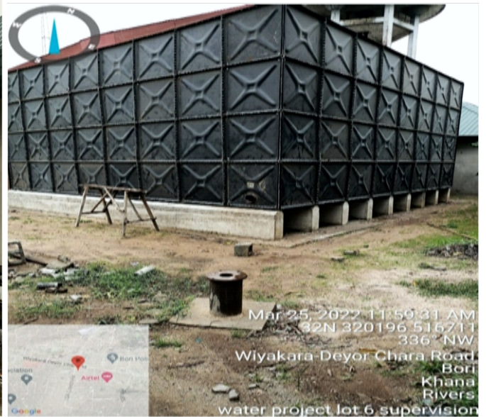
GROUND TANK FOUNDATION AT BORI
