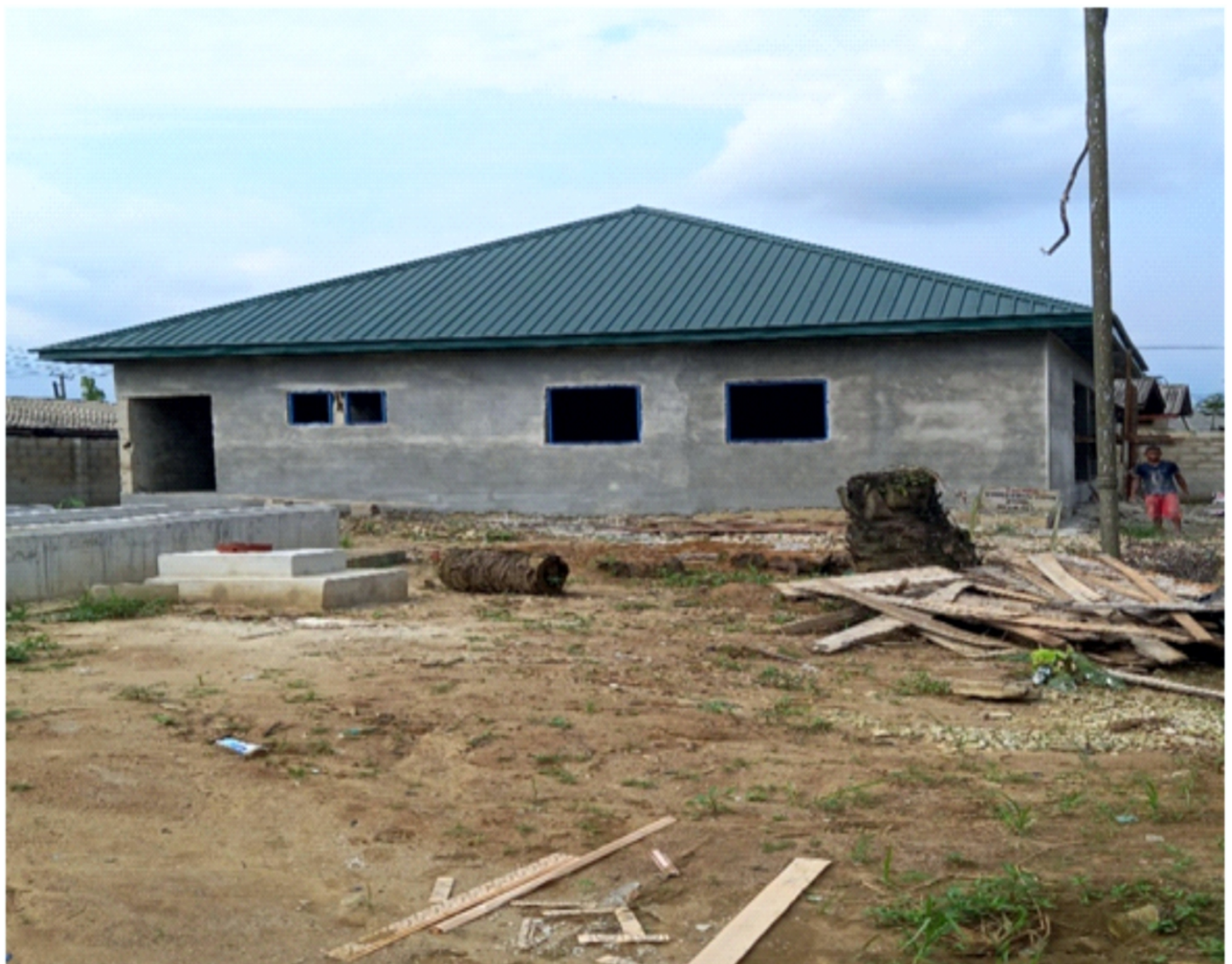
Treatment House at Ebu
