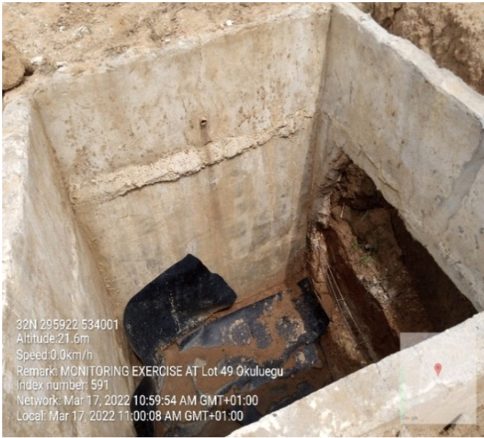
Collapsed sump of Lot 49
