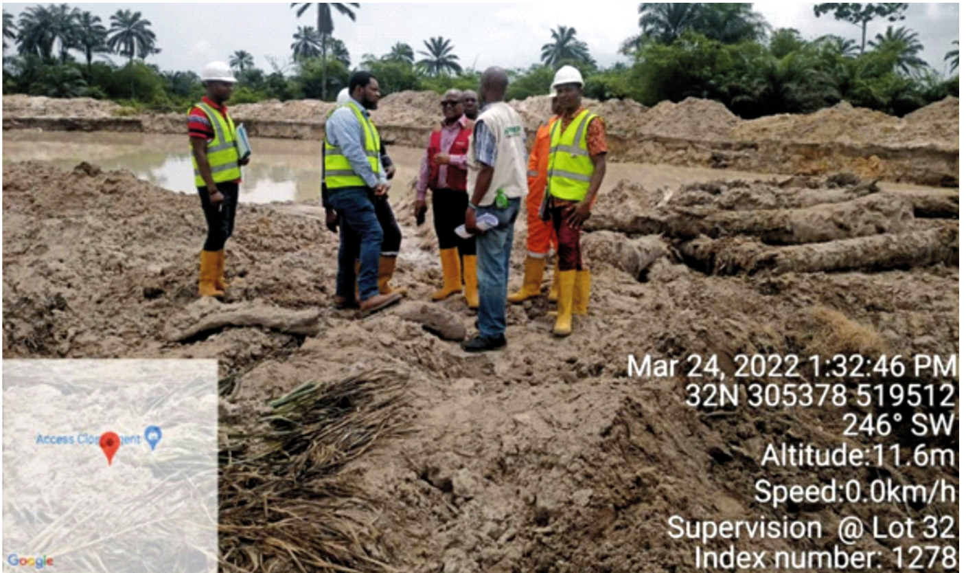
Plate 1.3: Excavation of impacted soil for treatment in progress at Lot 032 B-Dere/Gio, Gokana/Tai L.G.As. Remediation Contractor -MOSITO ENVIRONMENTAL LTD.
