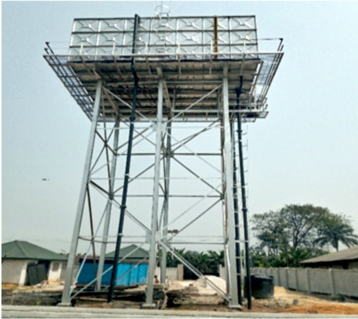
Overhead tank construction at Ebu
