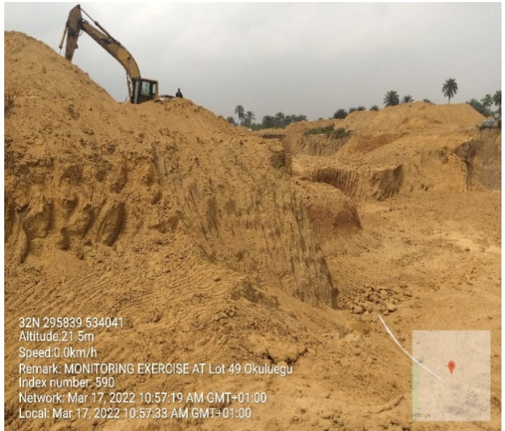
Excavation of contaminated soil at Lot 049
