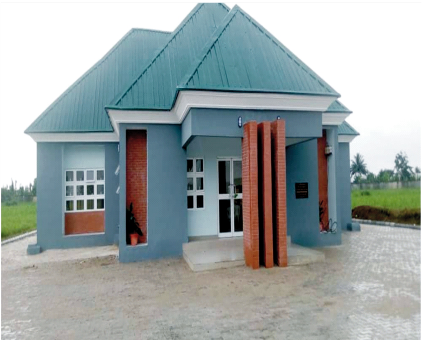
Picture of the External Building at Bori
