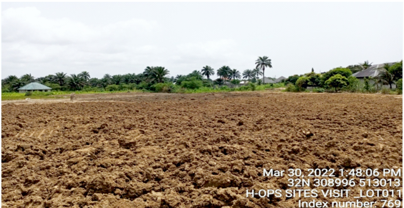
Plate 1.1: A panoramic view of Lot 011 at Debon, Bodo/Mogho, Gokana L.G.A. where final backfilling of excavated pits with the treated soil was recently concluded. (Contractor: MOSVINNY NIG. LTD).
