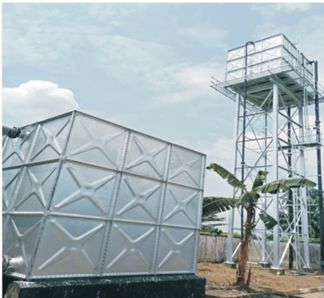
Replace brazing of vandalized overhead tank at Alesa Booster station
