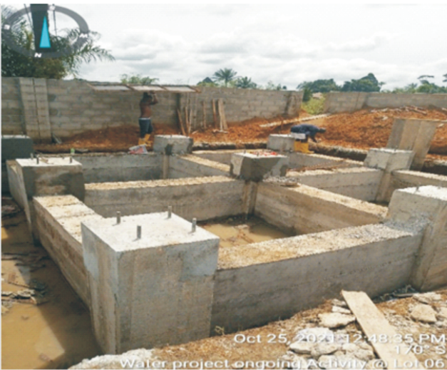
Treatment House and Ground tank foundation under construction at Kpean
