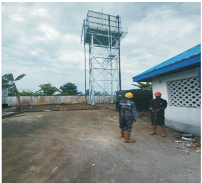
Rehabilitated Generator House and Pump House at Agbonchia
