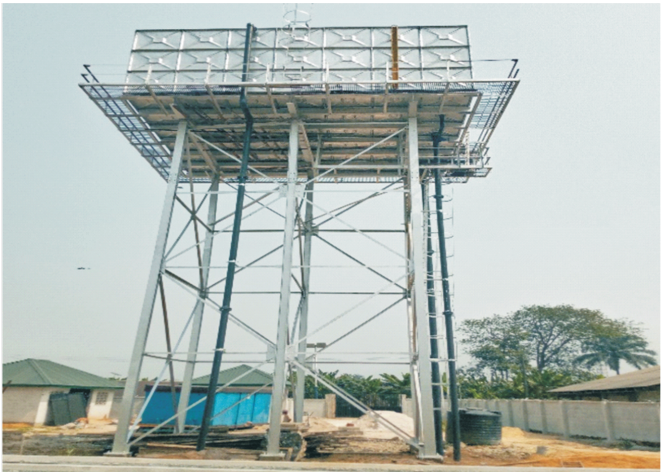
Completed Overhead Tank at Ebulu
