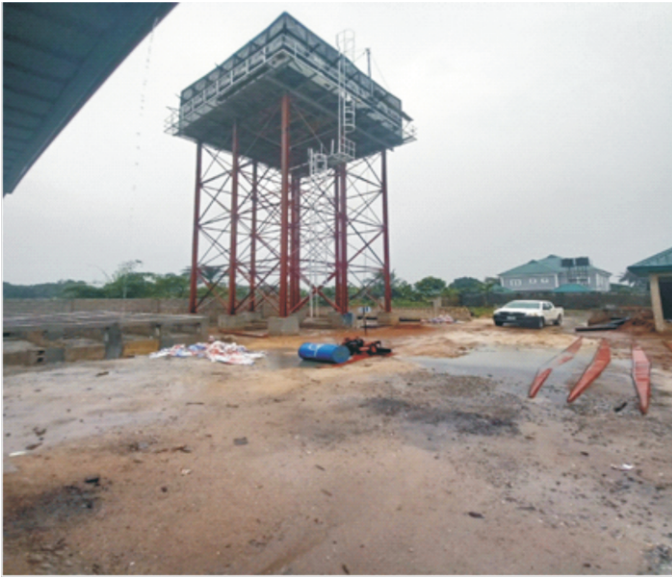
Constructed Overhead Tank at Korokoro
