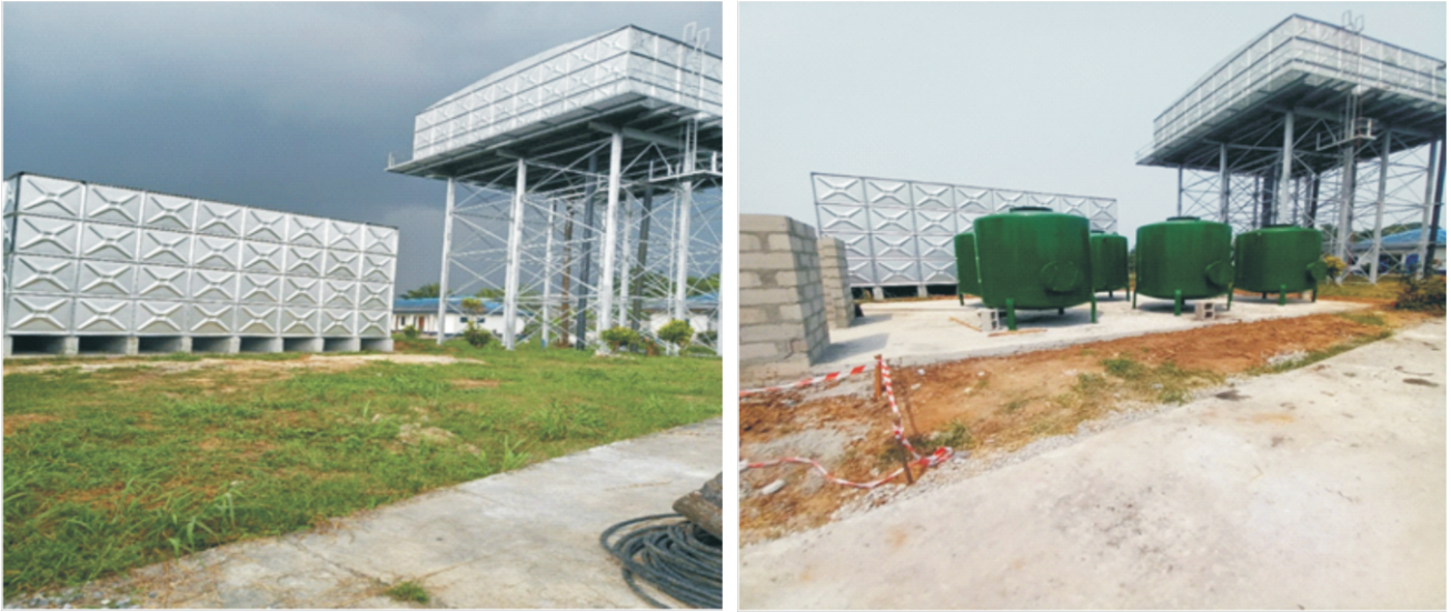
Completed and installed Ground/Elevated tanks and Pressure filter at Terabo
