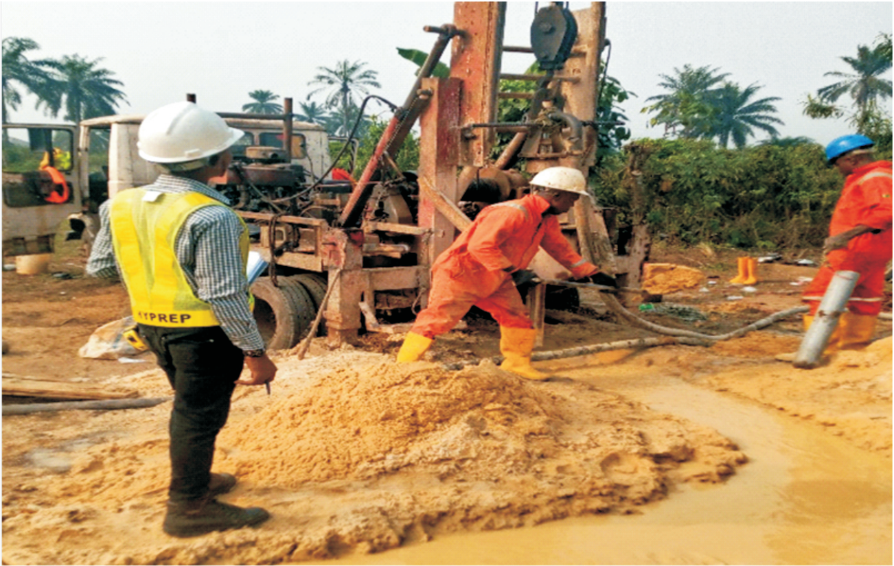
Drilling of Borehole at Ogale
