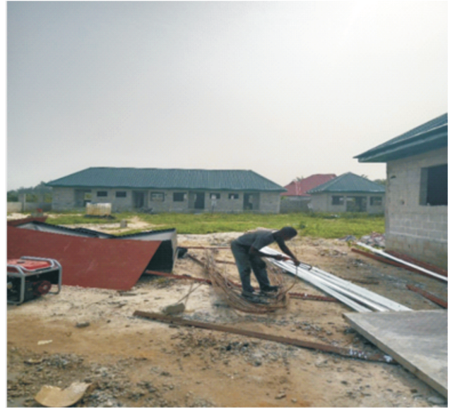
Ongoing Construction of Treatment house at korokoro
