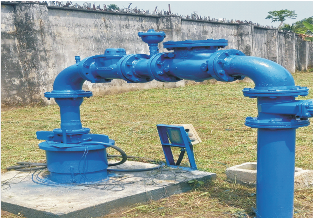
Completed and installed Borehole Head at Terabo
