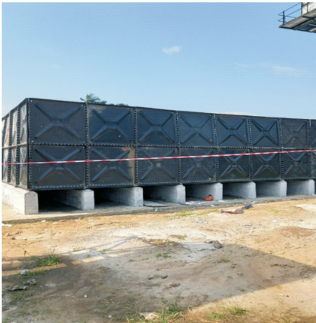
Installed Ground tank at Terrabo
