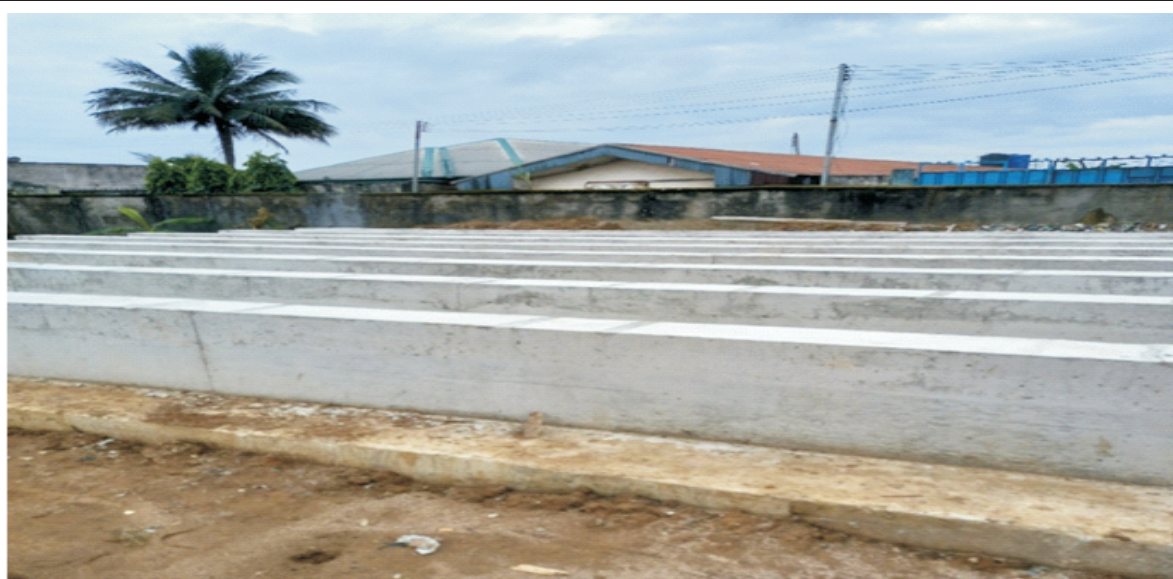
Construction of Foundation for Ground tank at Ebubu water station
