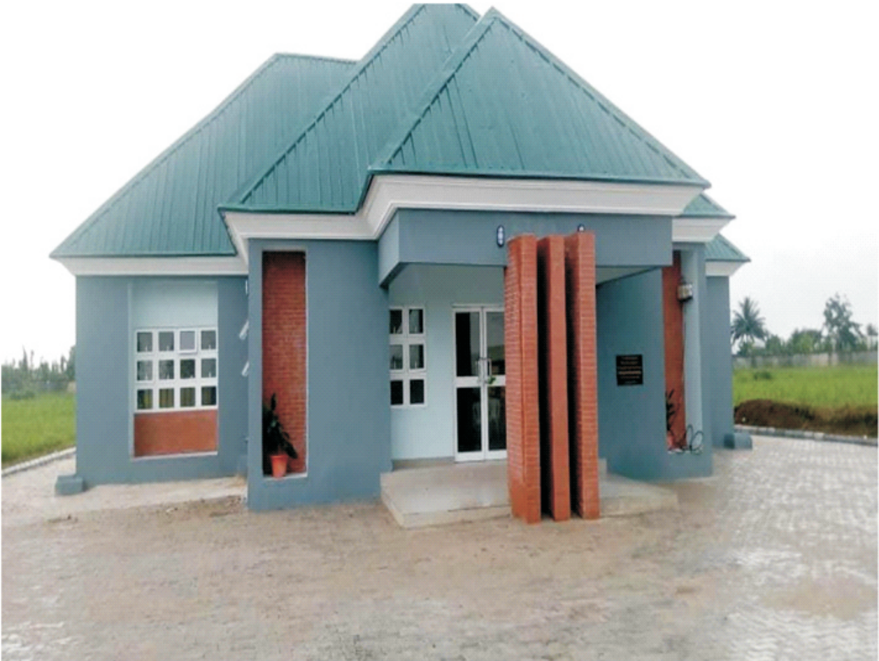
Completed and Commissioned Area Office at Bori, Khana LGA
