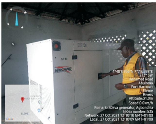
Pump House at Agbonchia
