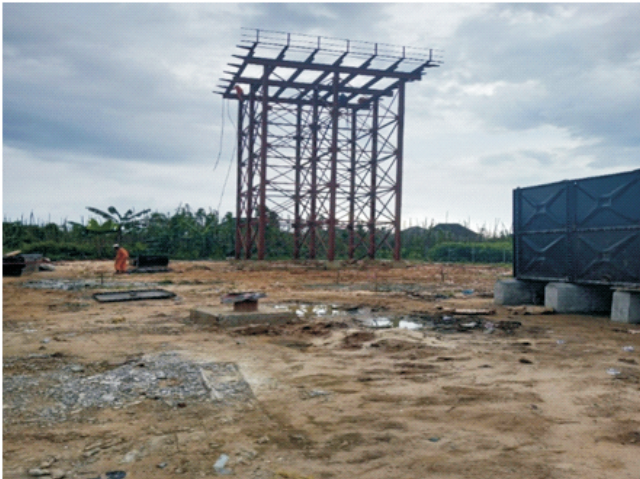
Stanchion installation at Barako
