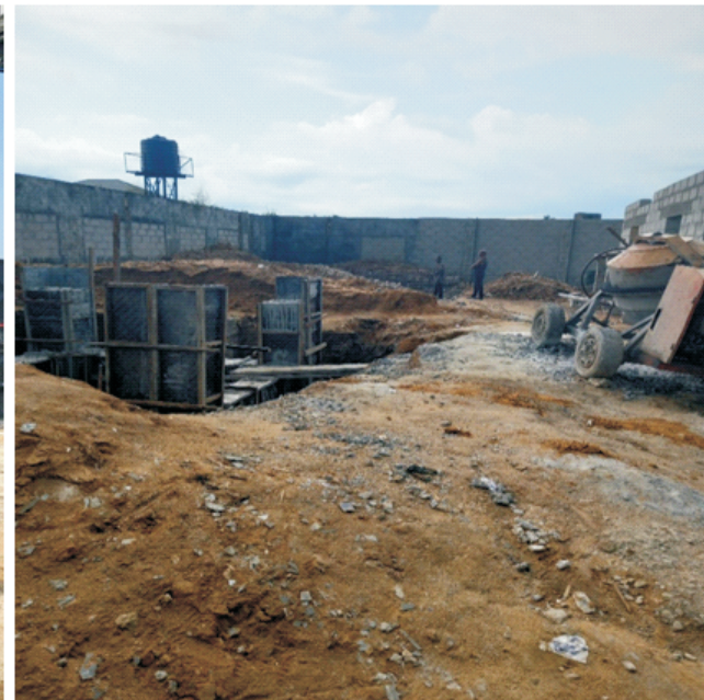
Overhead and Ground Tanks under construction at Biara
