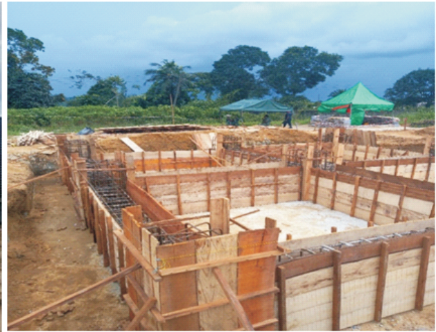
Overhead Tank foundation at B-Dere under
