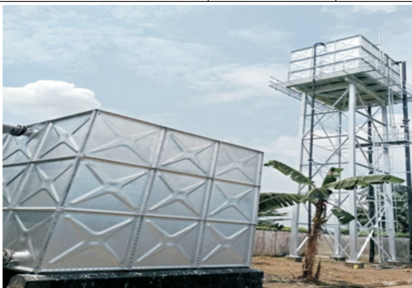
Rehabilitated surface and overhead tanks at Alesa water station
