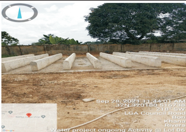
Ground Tank foundation at Bori
