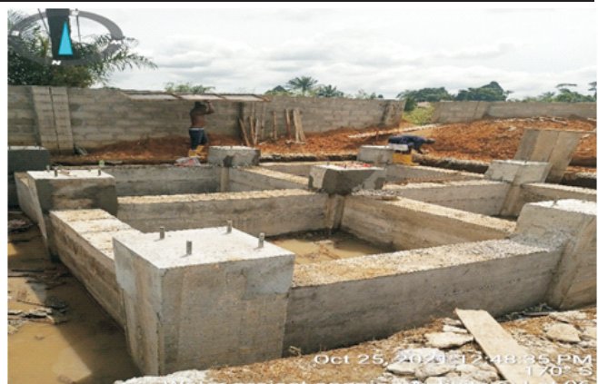
Overhead Tank foundation at Kpean
