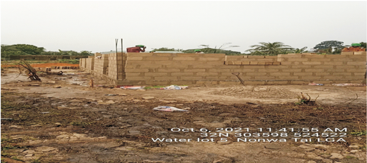
CT Construction of Treatment House in progress at Nonwa
