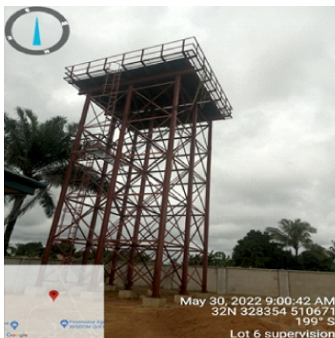
Installation of Elevated tank stanchion at Kpean facility
