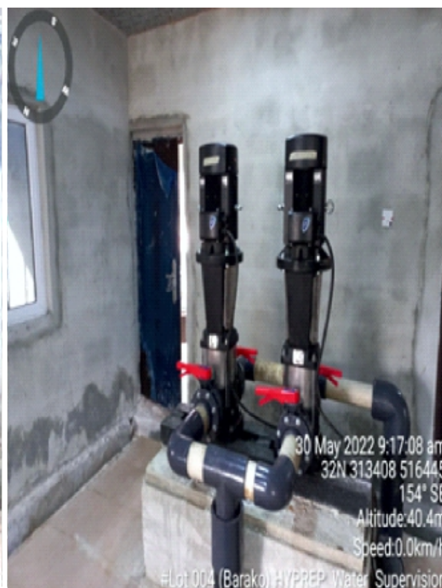
Newly installed high lift pumps
