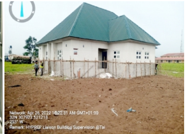
Figure showing external wall screeding and landscaping
