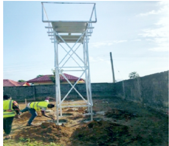
Picture showing erected stanchion
