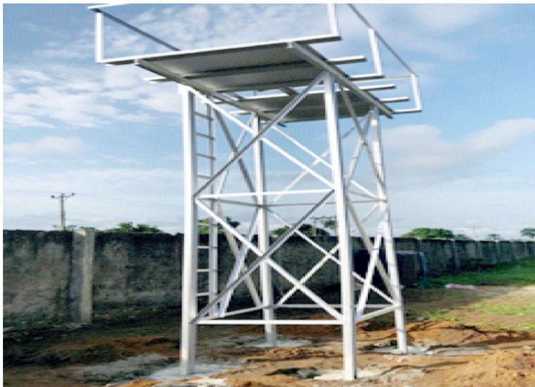
Picture showing erected stanchion
