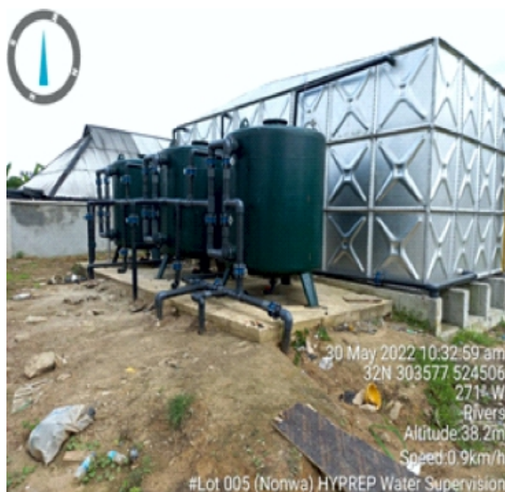
Connection of filters and storage tanks ongoing at Nonwa, Tai LGA
