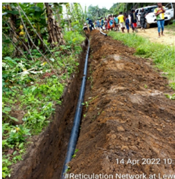
Reticulation (Pipe laying) at Lewe, Gokana
