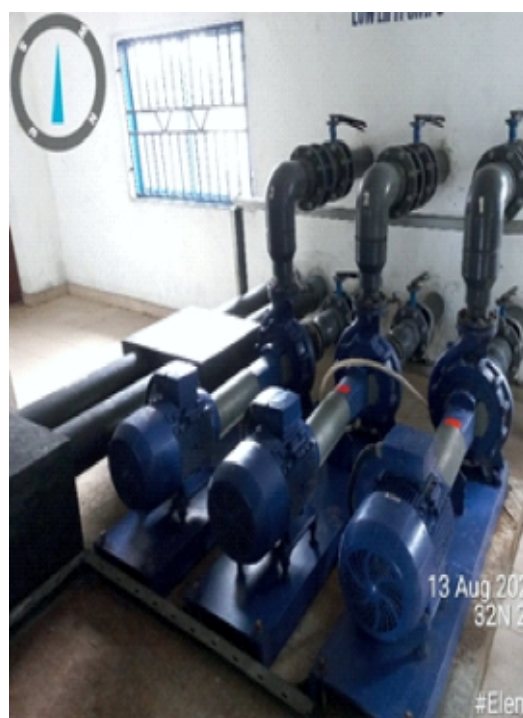
Low-lift pumps at Alesa Headworks
