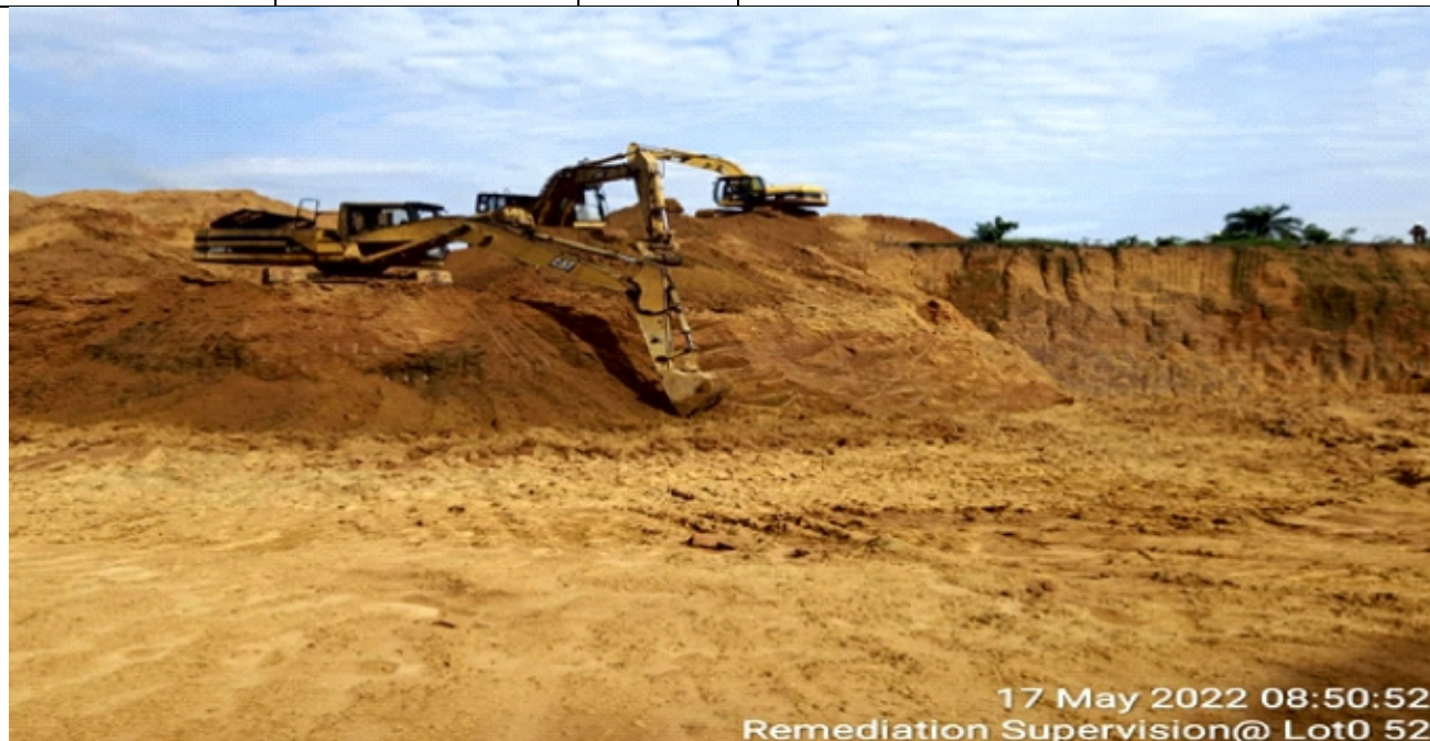
Plate 1.2: Excavation of impacted soil for treatment in progress at Lot 052 Okuluebu Ajeokpori Well 3, Ogale Eleme L.G.A.
