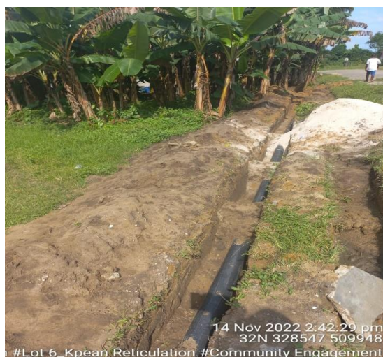
Fig. 4.7a: Ongoing reticulation at Kpean, Khana LGA
