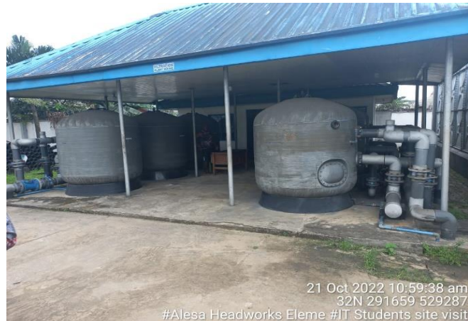
Plate 4.2b: Filtration system at Alesa Headworks
