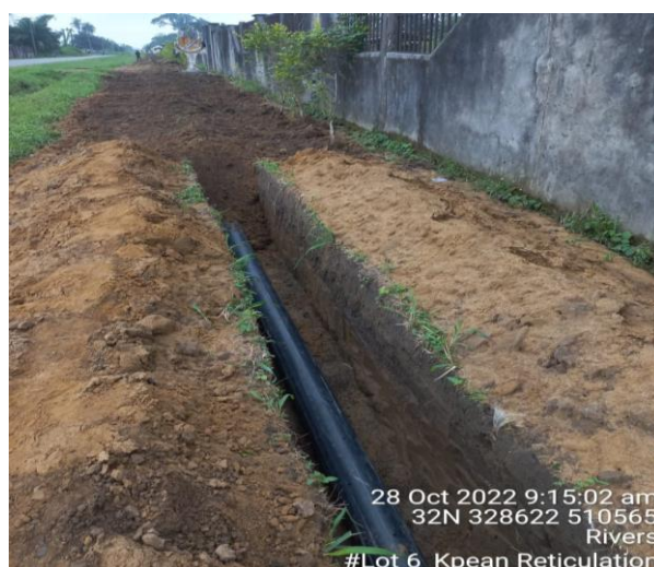
Fig. 4.7b: Ongoing reticulation at Kpean, Khana LGA
