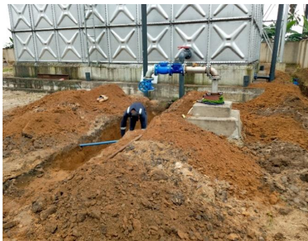
Plate 4.3b: Internal connection ongoing at Ogale, Eleme LGA.
