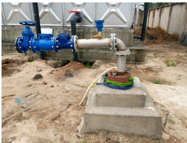
Plate 4.3a: Well head installation at Ogale, Eleme
