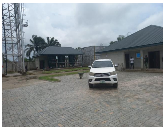
Plate 4.5a: Landscaping completed at Lot 4, Barako Station.
