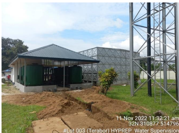
Plate 4.4a: Internal pipe connections ongoing at Terabor Station
