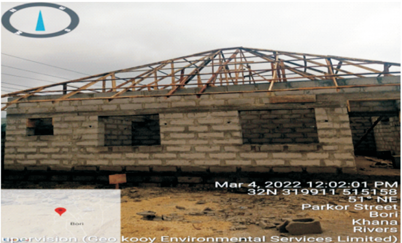
Pump house at Bori Booster Station under construction
