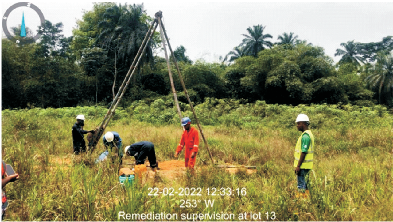
Plate 1.2: Installation of post-remediation groundwater monitoring / defensive boreholes in progress at Lot 013, Nweekol Zorbuke, K.Dere, Gokana L.G.A.
