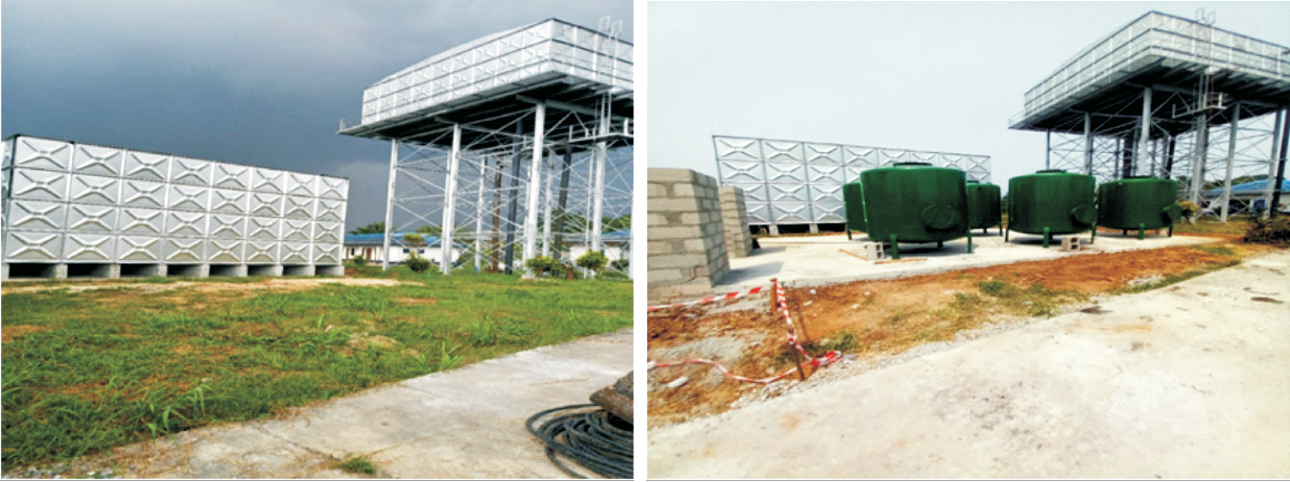
Ground tanks, Elevated tanks and Pressure filter at Terabo
