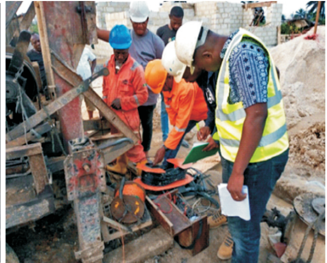
Borehole logging at Ogale
