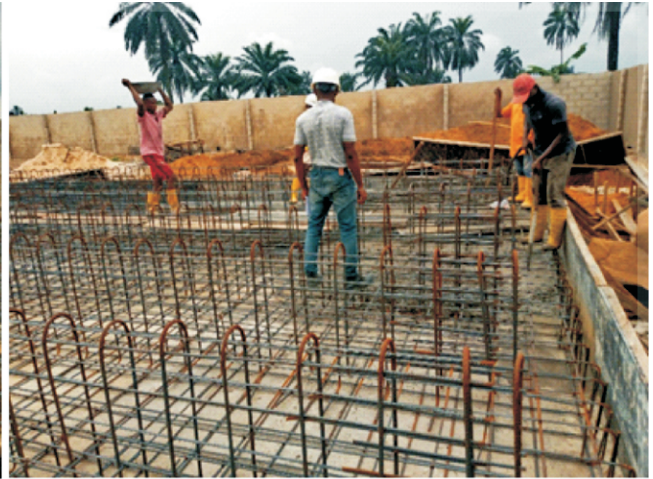
Construction ground tank foundation At Ogale
