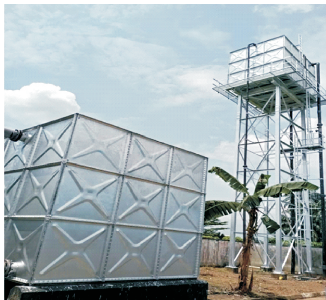
Installed Overhead and Surface tanks at Agbonchia
