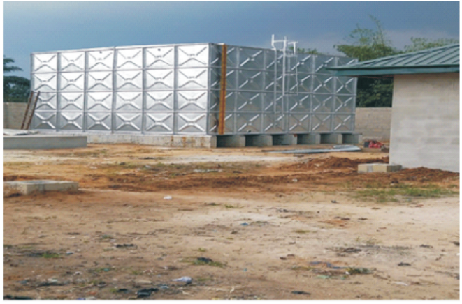
Constructed and installed Overhead and Surface tanks at Barako
