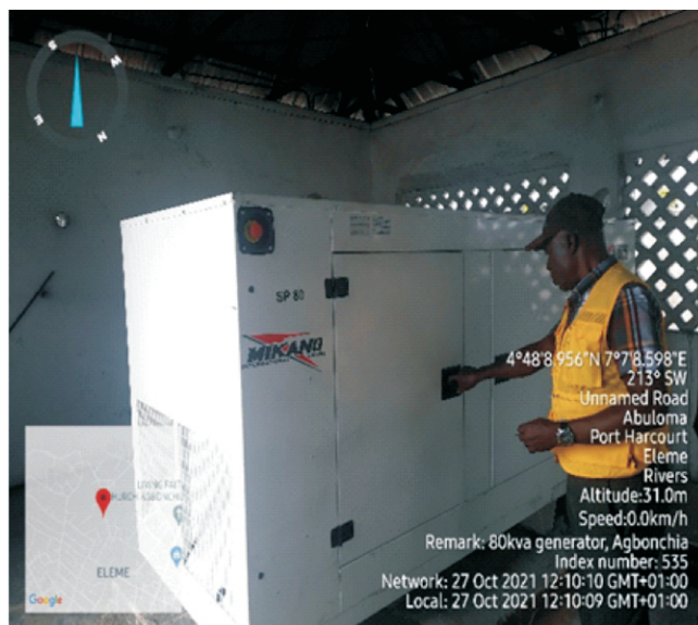
Installed Generator at Alesa Booster Station
