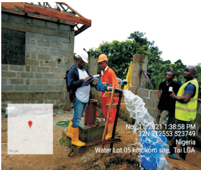
Staff Quarters under construction at Nonwa
