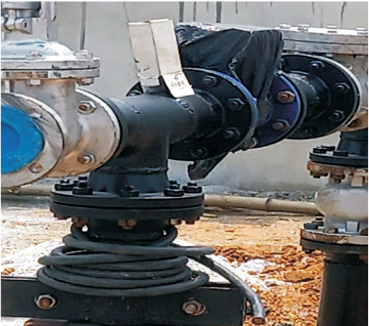
Installed Borehole head at Barako
