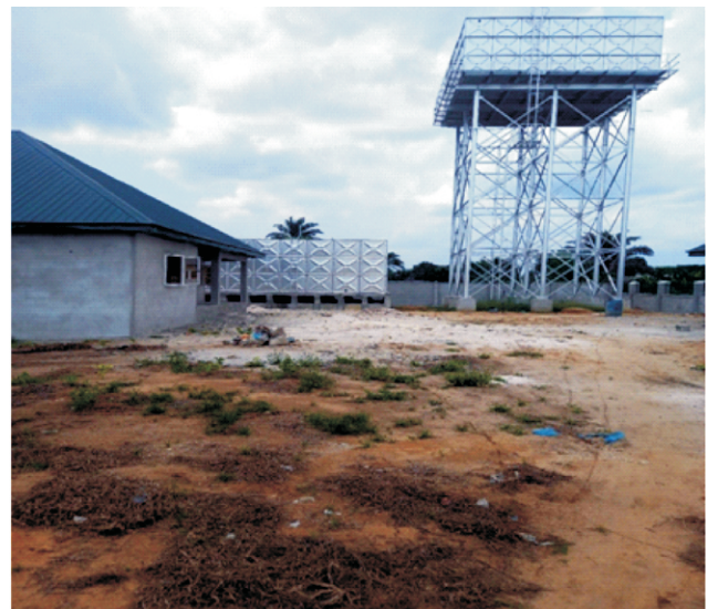
Installed Surface and Overhead tanks at Korokoro
