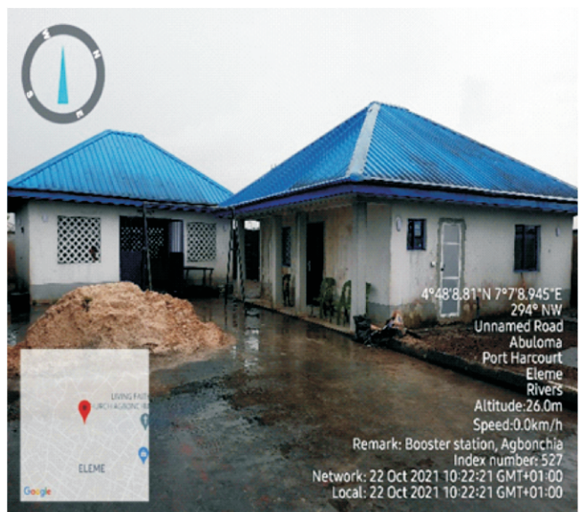
Pumping House at Agbonchia
