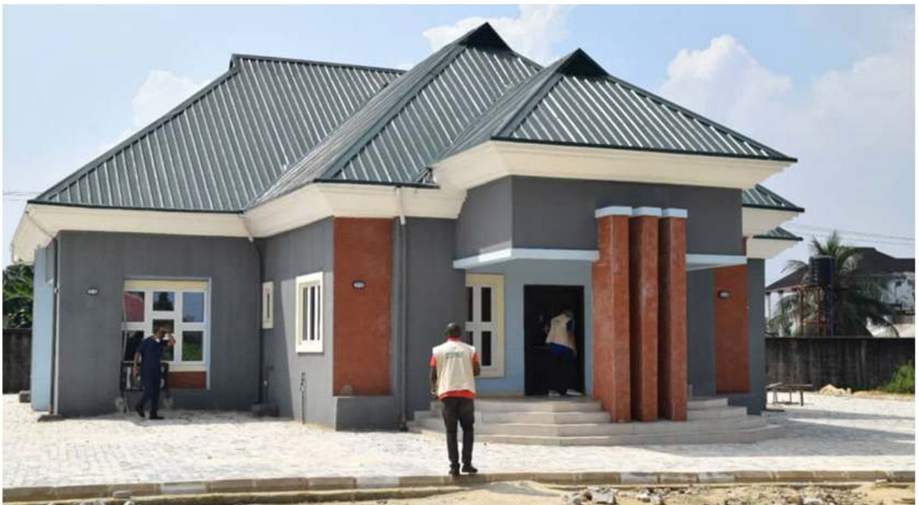
Completed and handed over Area Office at Eleme LGA
