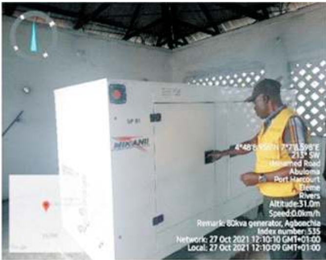
Pump House at Agbonchia
