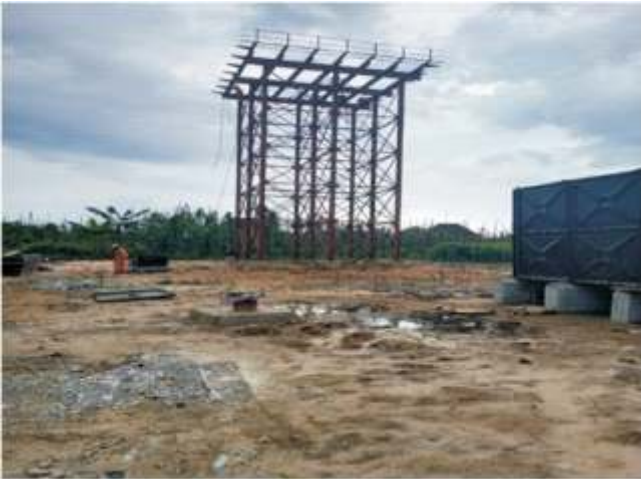
Stanchion installation at Barako
