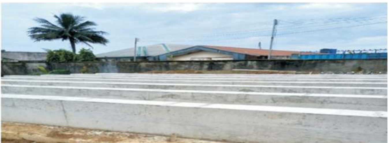
Construction of Foundation for Ground tank at Ebubu water station
