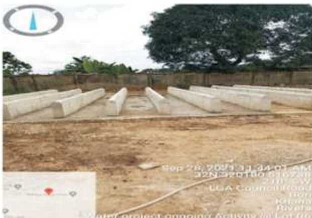
Ground Tank foundation at Bori
