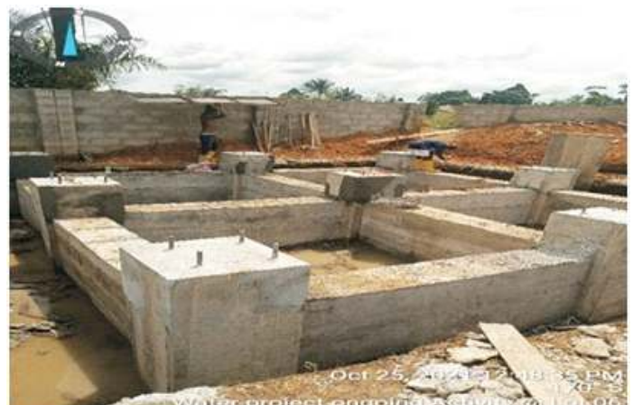
Overhead Tank foundation at Kpean
