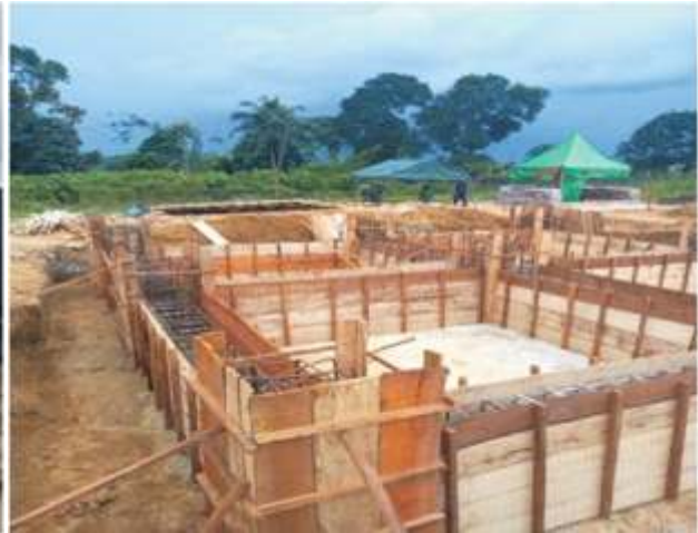
Overhead Tank foundation at B-Dere under
