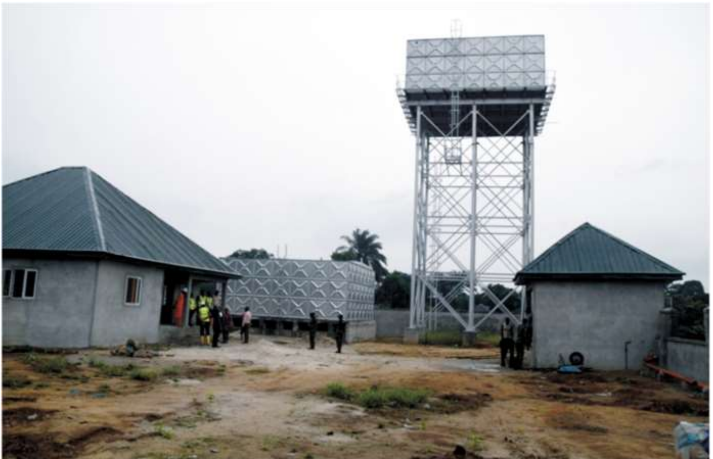
Plate 1.7: Head of Operations visit to HYPREP Potable Water Supply Project under construction at Korokoro, Tai L.G.A during his Supervisory field visit on 3 rd March, 2022.
