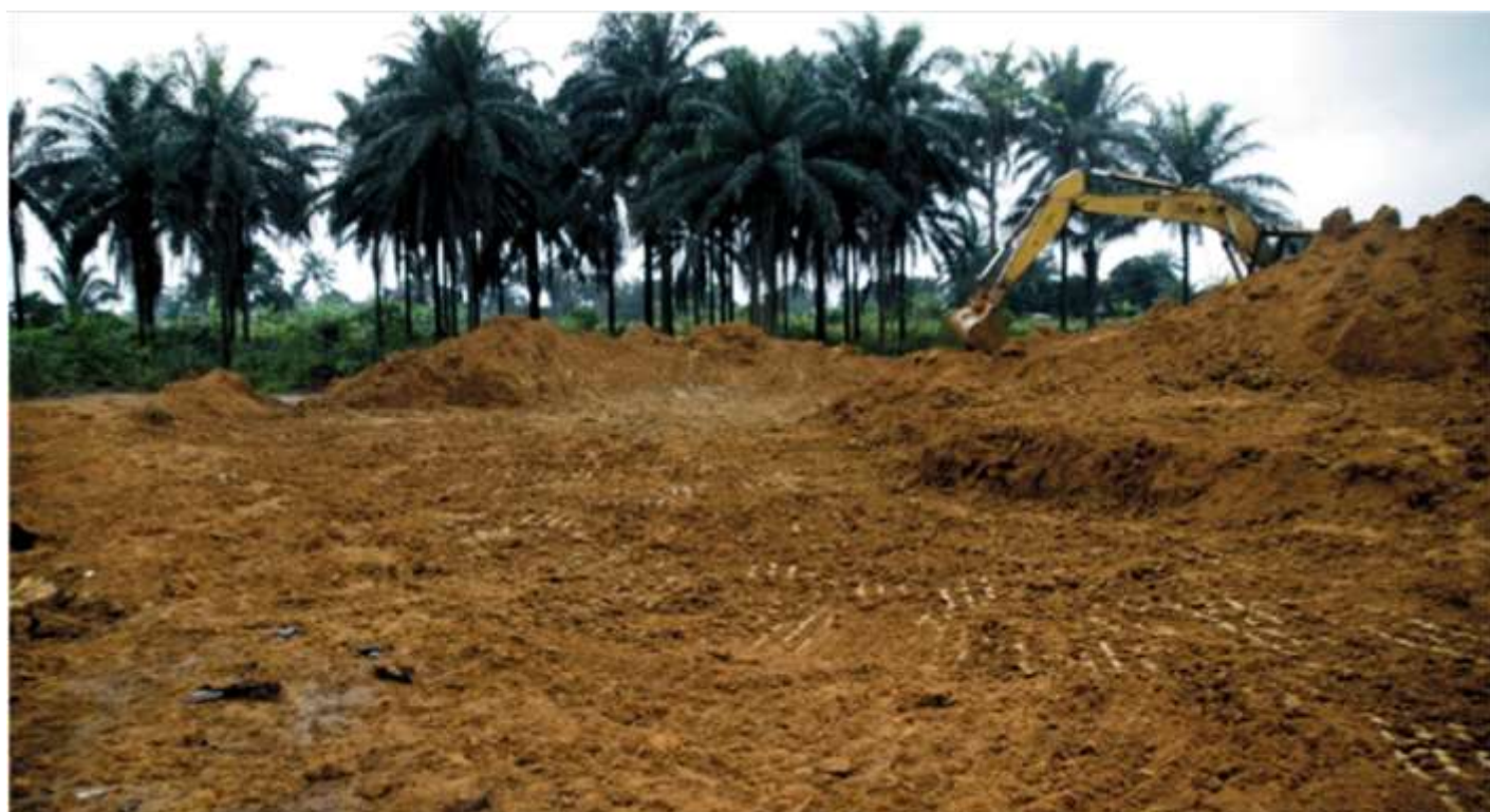
Plate 1.4: Final stage of backfilling, site leveling and landscaping in progress at Lot 029 (Bara Alue, Tai L.G.A) as at 3rd March, 2022. Remediation Contractor -WEAFRI WELLS SERVICES LTD.
