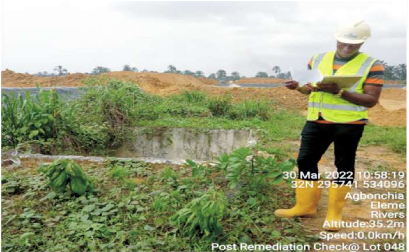
Plate 1.11: Team of Remediation Supervisors undertaking checks on levels of compliance with completion of remediation earthworks and decommissioning of site facilities at Lot 048 (Okuluebu, Ogale, Eleme L.G.A).
