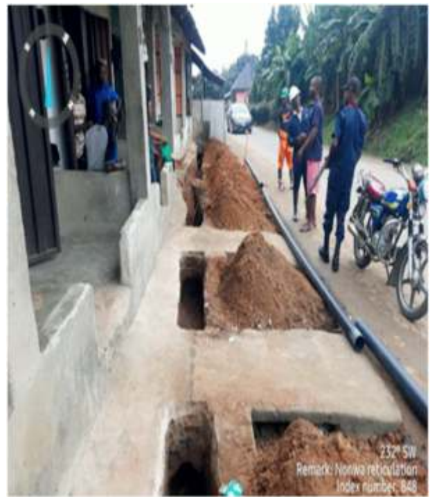
Plate 4.6b: Ongoing reticulation at Nonwa, Tai LGA
