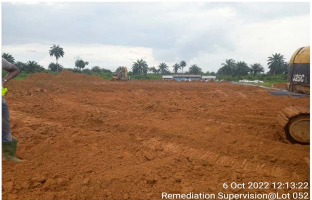
Plate 2.8: Mechanical Transferring of Treated Soils to the Storage Area at Lot 052 Okuluebu -Eleme LGA.
