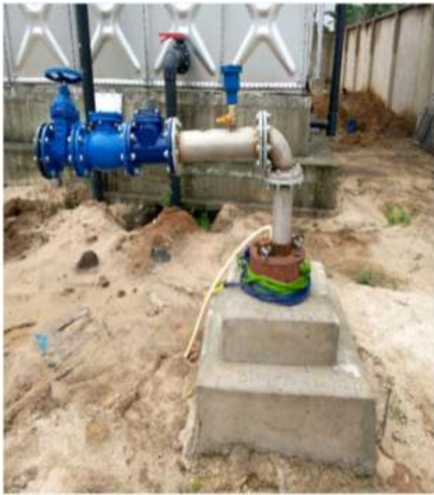
Plate 4.3a: Well head installation at Ogale, Eleme
