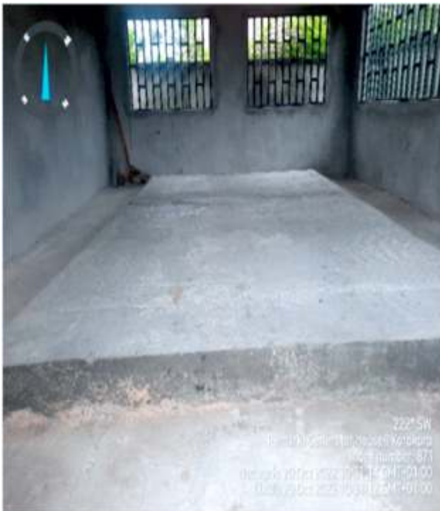
Plate 4.6a: Newly constructed generator base, Korokoro station, Tai LGA.
