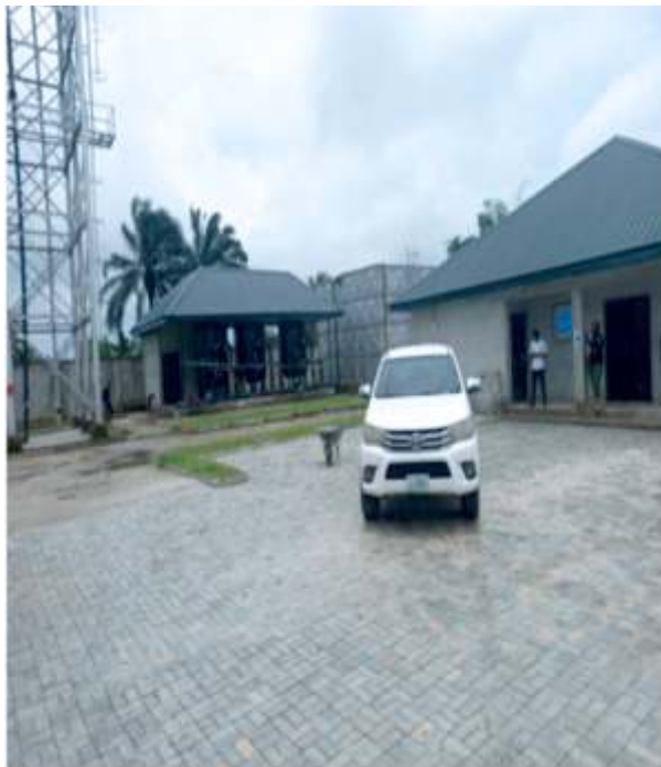
Plate 4.5a: Landscaping completed at Lot 4, Barako Station.
