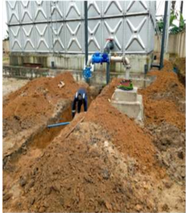
Plate 4.3b: Internal connection ongoing at Ogale, Eleme LGA.
