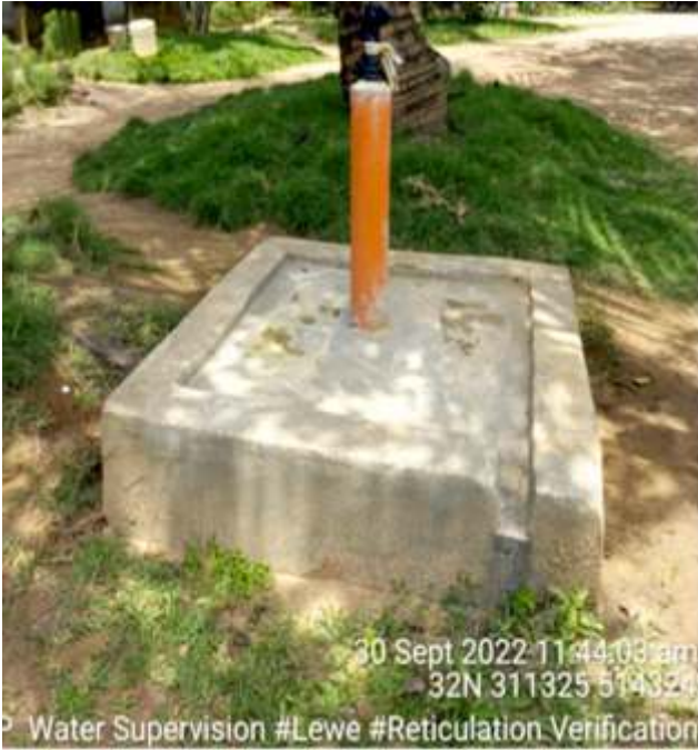
Plate 4.4a: Ongoing construction of fetch point at Lewe, Gokana
