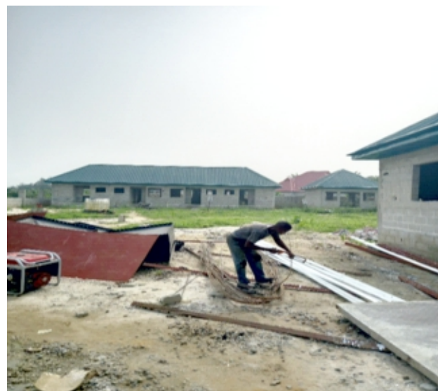
Staff Quarters, Treatment house at Korokoro Lot 6: Bori/Kpean Khana
