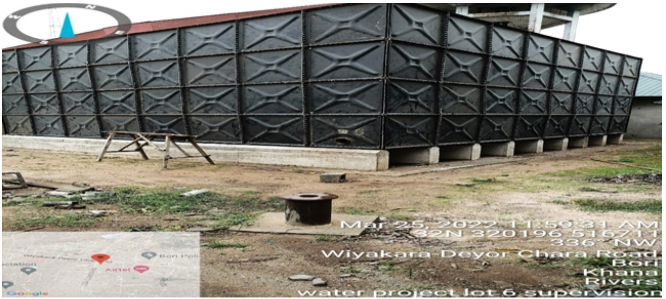
GROUND TANK FOUNDATION AT BORI
