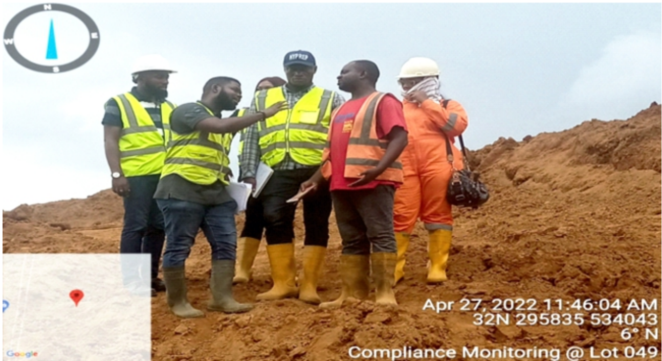
Plate 1.10: Team of Remediation Supervisors undertaking checks on levels of compliance of Contractors in their Remediation Works at Lot 049 (Okuluebu Ajeokpori Well 3, Ogale, Eleme L.G.A).(Lot 049 Contractor: ENVIRON CONSULT AND REMEDIAL SERVICES LTD)
