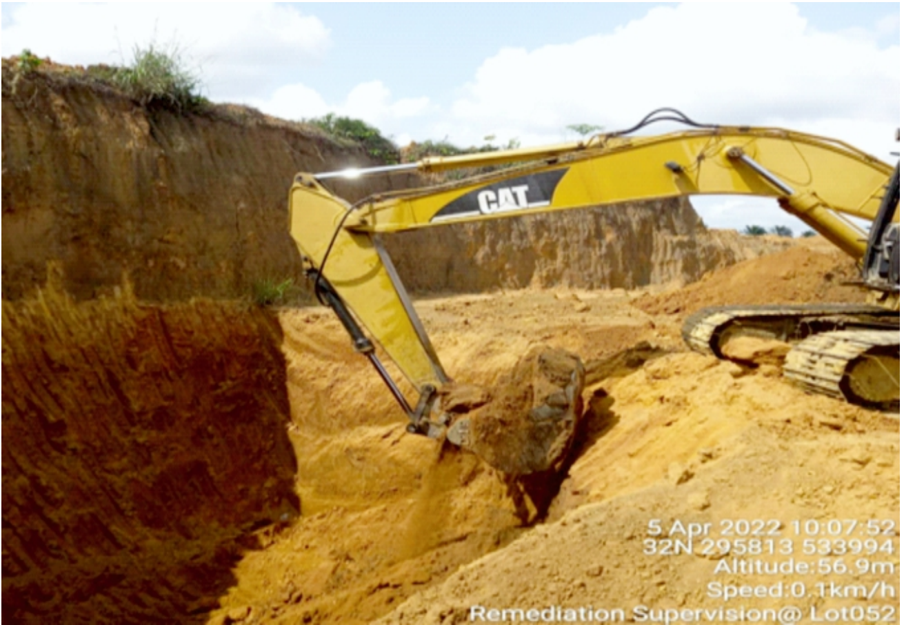
Plate 1.3: Excavation of impacted soil for treatment in progress at Lot 052 Okuluebu Ajeokpori Well 3, Ogale Eleme L.G.A. Remediation Contractor - MONTEGO UPSTREAM SERVICES LTD.
