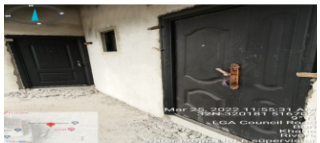
INSTALLATION OF DOORS ON BORI TREATMENT HOUSE.
