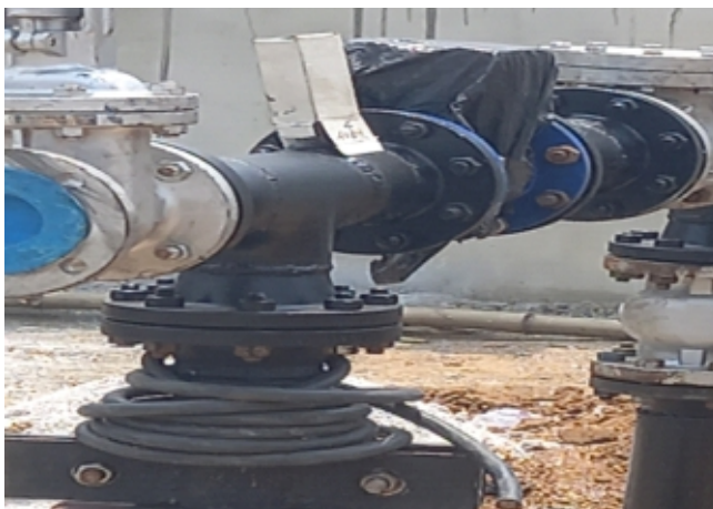
Borehole head installed at Barako.
