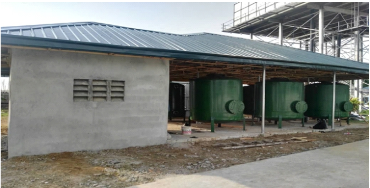
INSTALLATION OF PRESSURE FILTER AT TERABO
