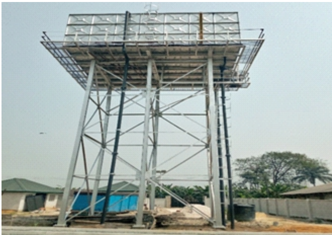
Over head tank construction at Ebubu
