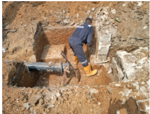
Ground tank construction at Ogale. Pressure filter installation at Ogale.
