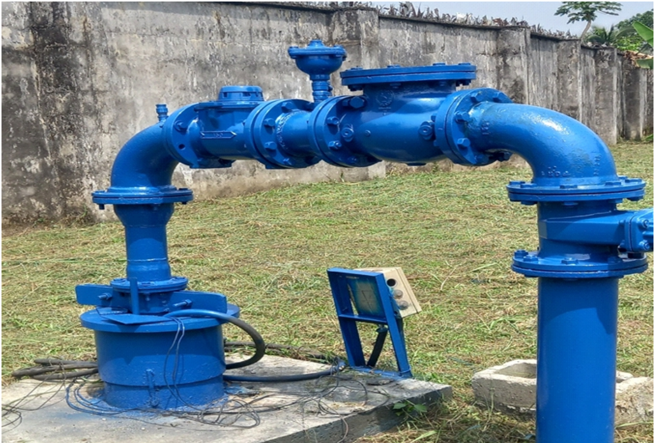
Completed Borehole head at Terabo
