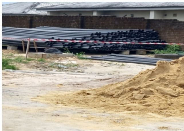
Pipe stack ready for laying
