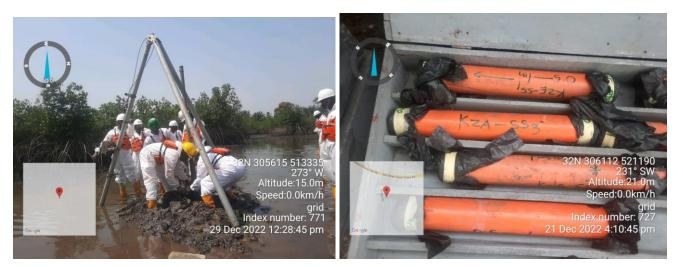
Plate 2.7: Vibro-coring/Boring operation and Characterization. Plate 2.8: Cut Cores labelled, containerized and prepared for sampling.
