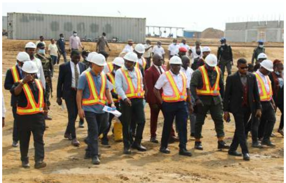
Hon. Minister of State for Environment, Dr. Salako Inspects work on Centre of Excellence for Environmental Restoration, Wiyaakara
