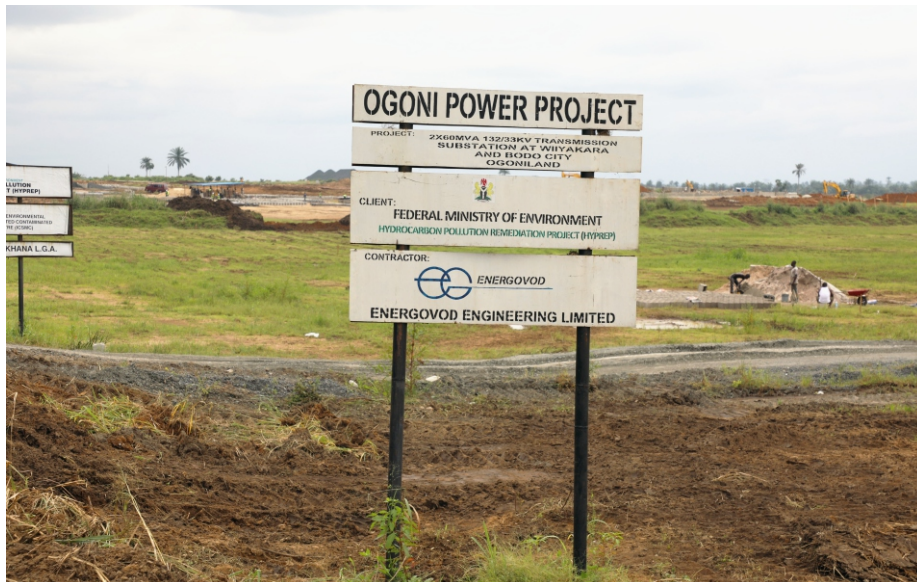
Ogoni Power Project Substation Site, Wiiyaakara
