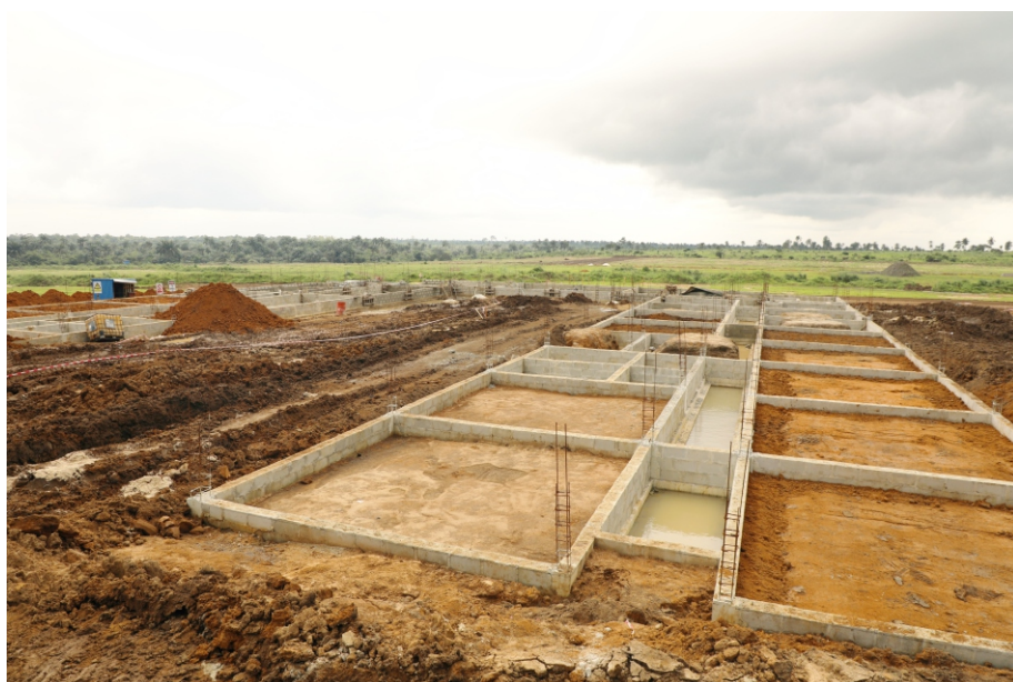
CEER Building under Construction
