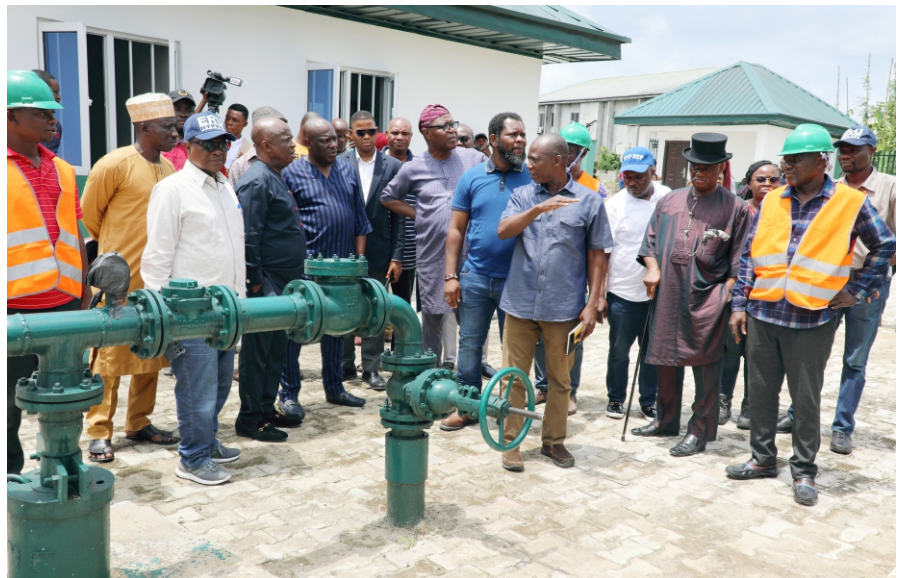
BoT Members on Inspection to HYPREP Water Station
