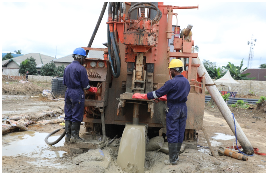
Well Drilling at Onne Water Station
