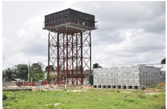
Water station under construction
