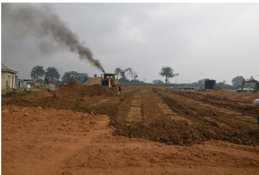
Backfilling of Remediated Soil in Progress
