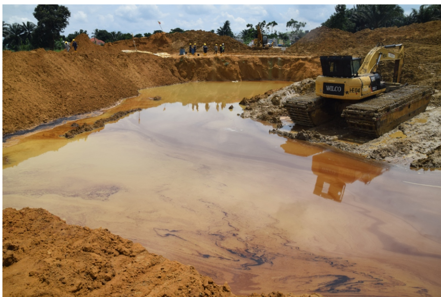
Excavation of Impacted Site in Progress
