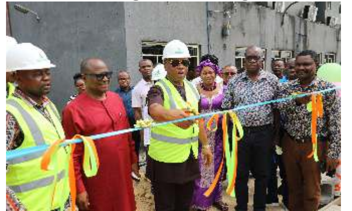
Dr. Giadom Cuts the Tape on New Generating Set to Power Project Office
