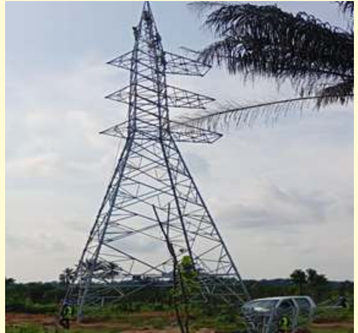
Erection of tower T5A DD90° completed
