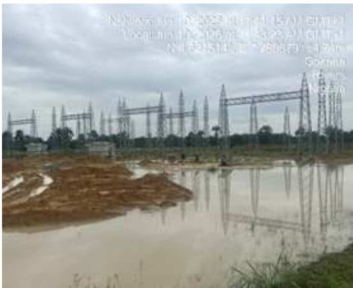
132kv Gantry Erection at Bodo Substation
