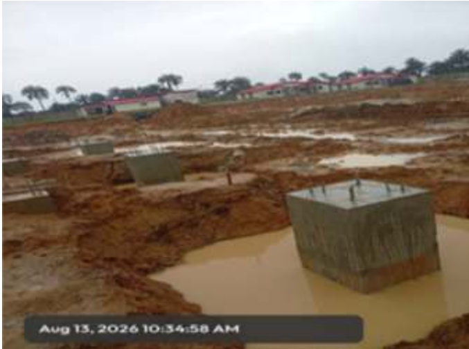
Construction of Disconnecter Switch Foundation at Bodo Substation
