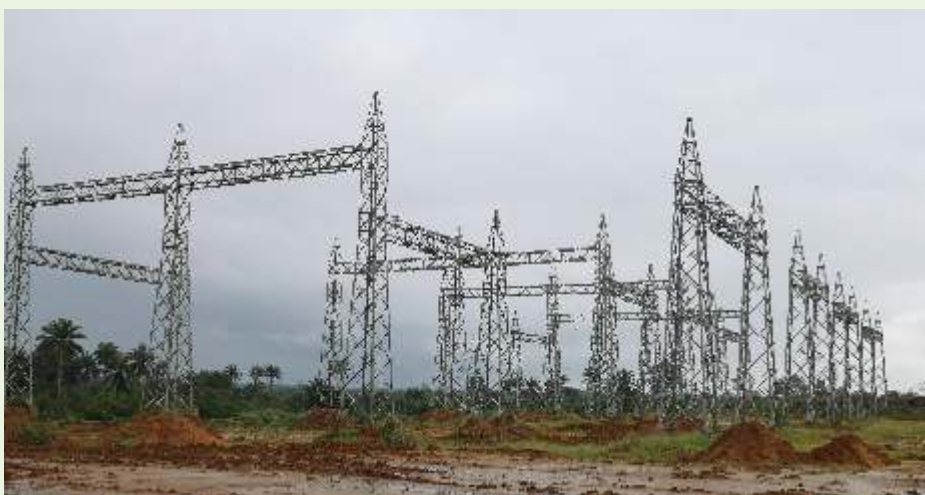
HYPREP Built Ogoni Power Substation Under Construction
