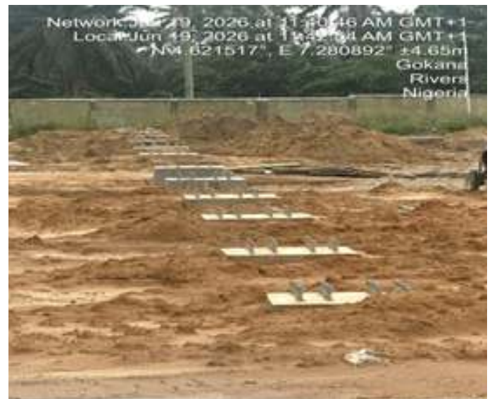
33kV Gantry Foundations at Bodo Substation
