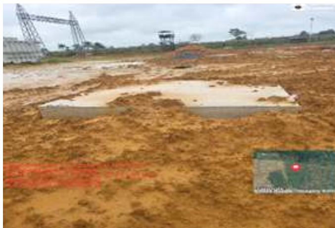
Construction of Earthing transformer completed at Wiiyaakara Substation
