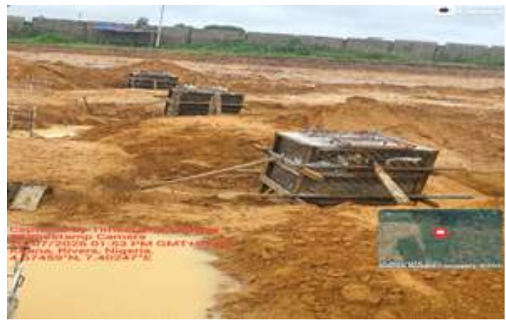
Construction of the Busbar Support Foundation at Wiiyaakara Substation
