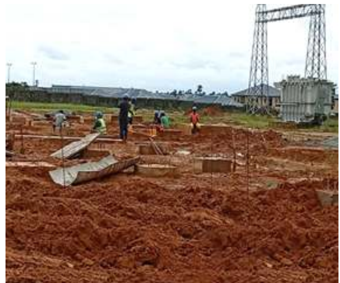
Construction of VT T61, CT T17, and 33 kV Bus DS foundations in progress at Wiiyaakara Substation
