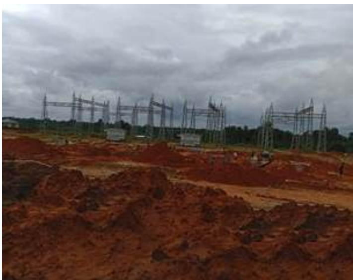
Erection of the 132kV gantry beams completed at Wiiyaakara Substation
