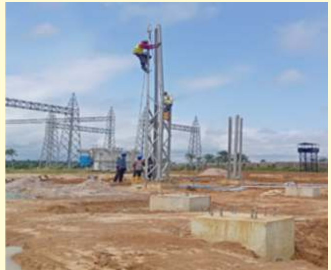
Erection of 33 kV Gantry in Progress at Wiiyaakara Substation
