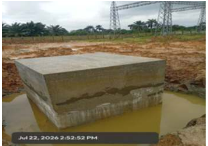
Earthing Transformer Foundation at Bodo Substation
