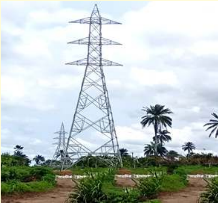
Erection of tower T6A DD2 Completed
