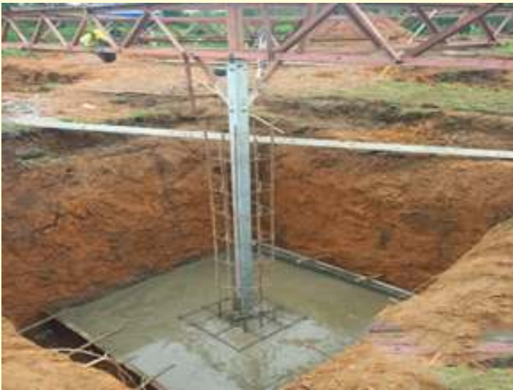
Concreting of Tower Foundation Pads for Tower T10A (DD2)
