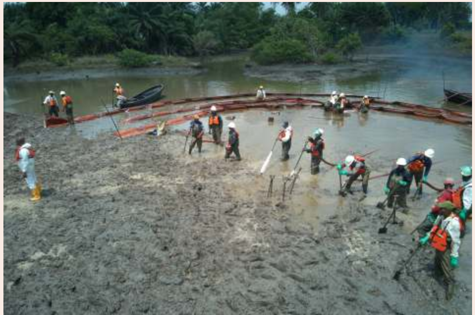
Sediment Flushing, Goi
