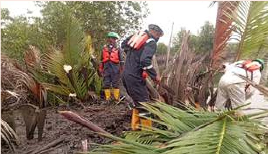
Nipa Palm Removal, Bomu
