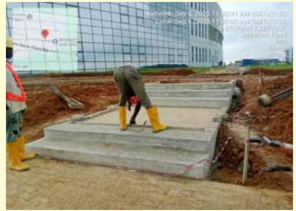
Internal Road Works
