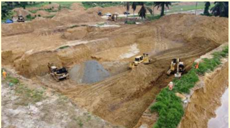
Excavation of Impacted Soil
