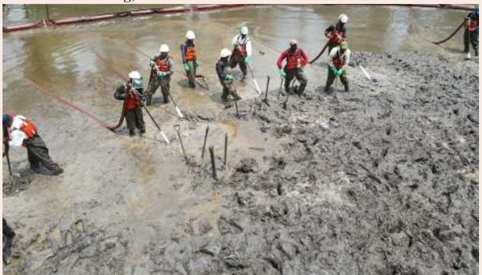
Sediment Flushing, K-Dere
