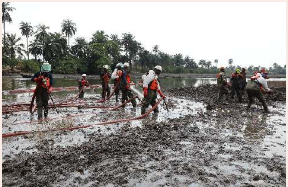
Sediment Flushing, B-Dere
