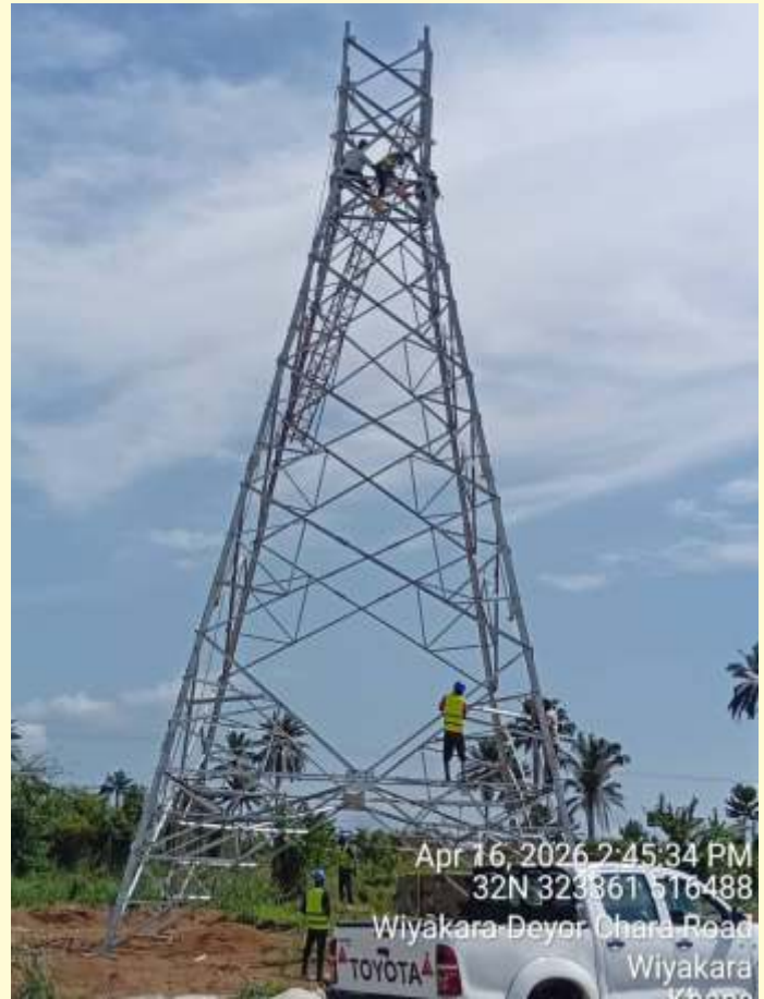
Erection of 1 st Tower T7A
