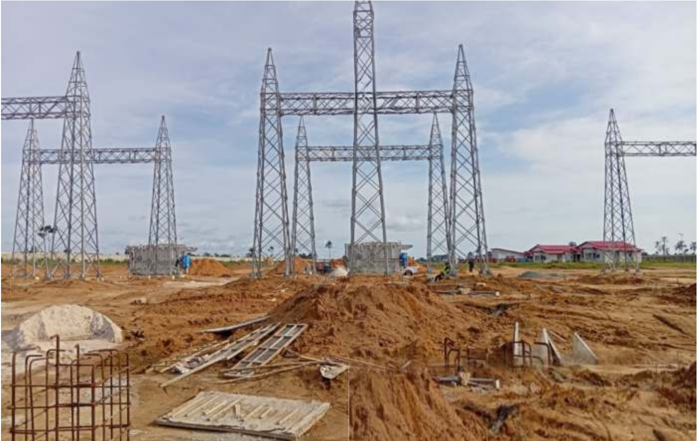
Erection of 17th 132 Gantry at Ogoni Power Substation
