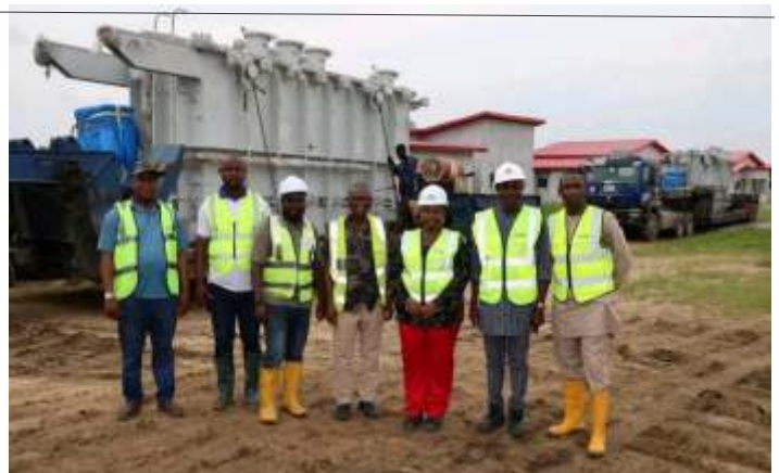
The Power Team Takes Delivery of 4x60MVA Power Transformers at the Wiiyaakara Substation
