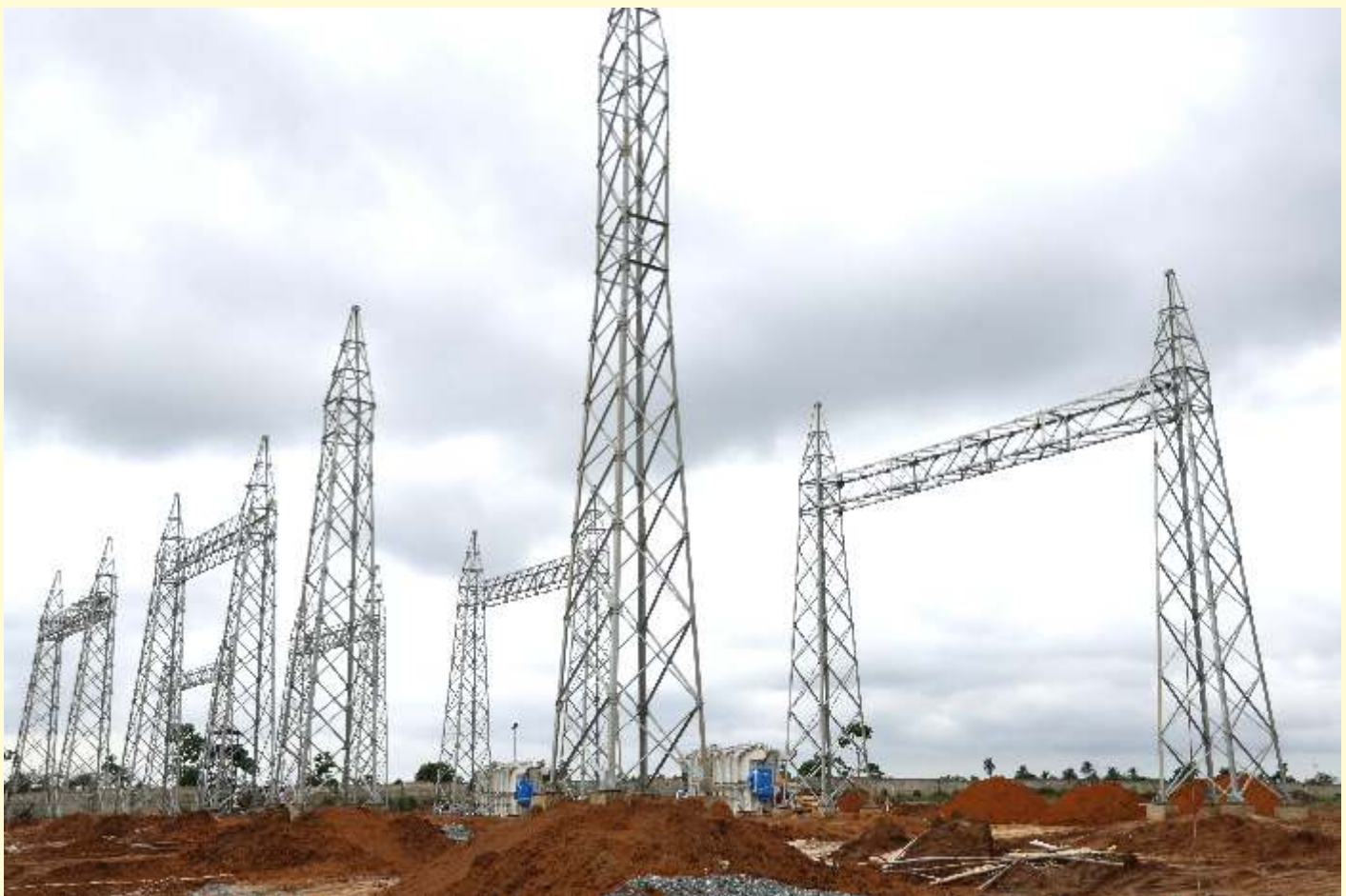
Erection of 17th 132 Gantry at Ogoni Power Substation
