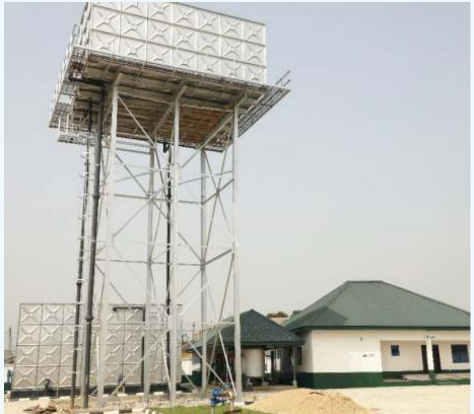
Facilities at HYPREP Water Station
