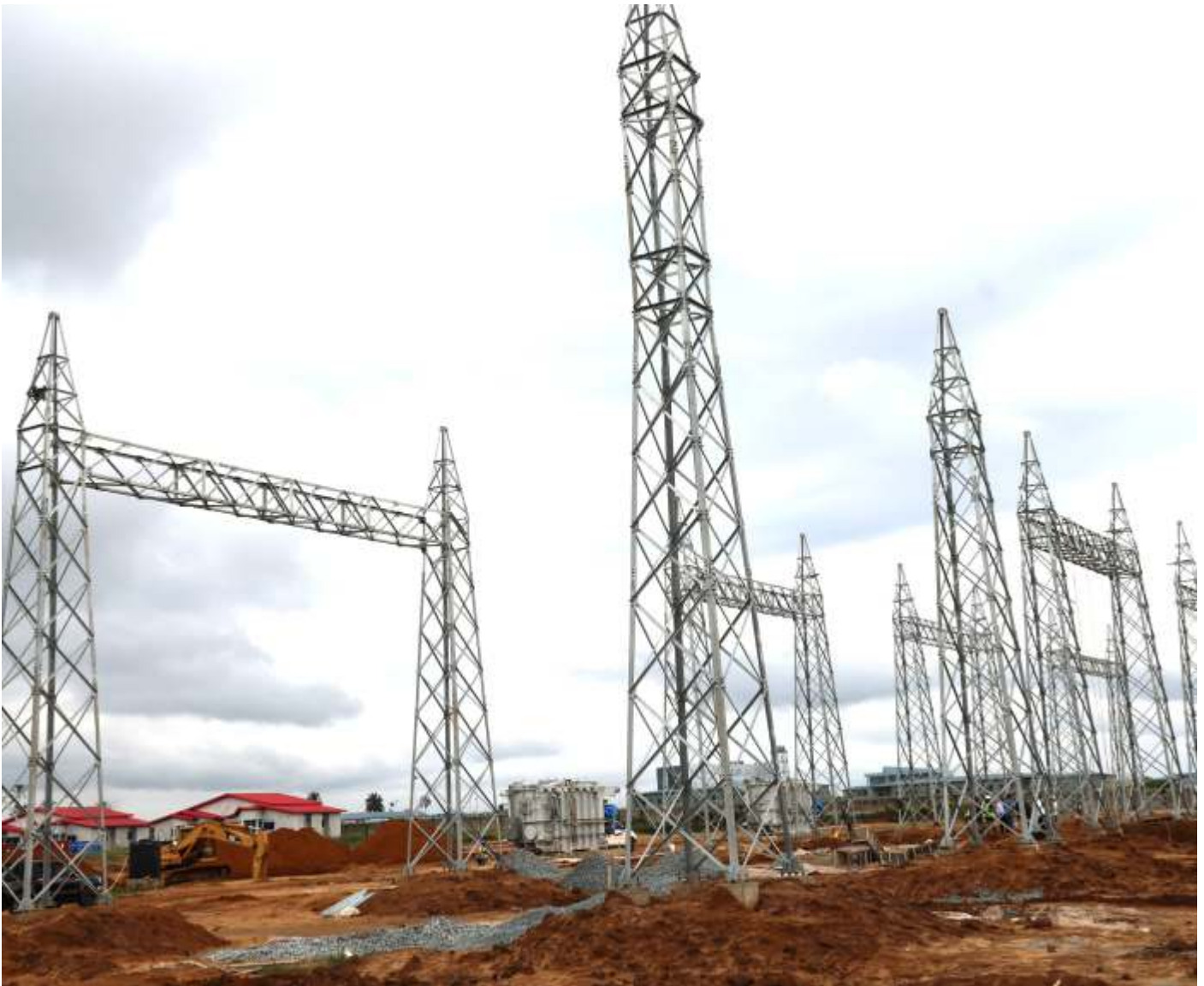
Erection of Gantries at Ogoni Power Substations
