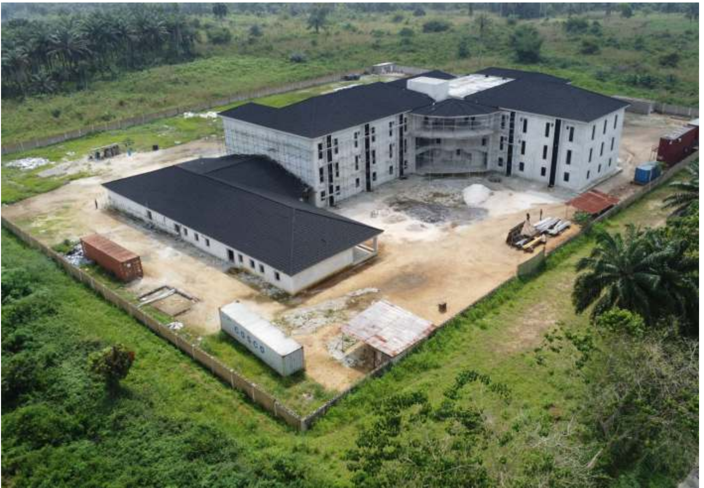
Ogoni Specialist Hospital (78% Completed)
