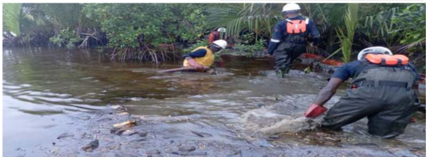
Plate 8: Sediment Flushing -Bomu
