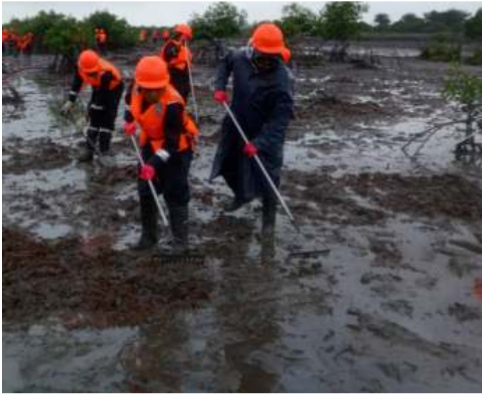
Plate 5: Raking and Agitation – B-Dere
