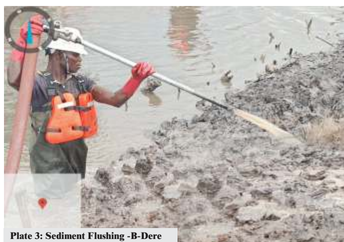
Plate 4: Sediment Flushing -B-Dere
