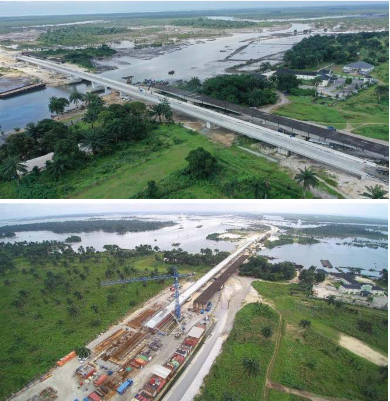
Figure 19: Bodo-Bonny Road under construction and due to link the LGAs of Tai and Khana
