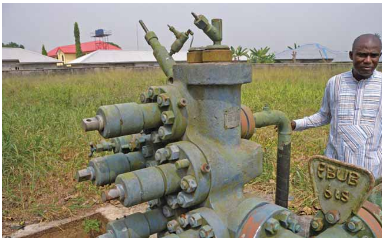
A UNEP project team member at a wellhead at Ebubu Ejama, Eleme LGA, typical of the oil infrastructure progressively installed in Ogoniland since the late 1950s
