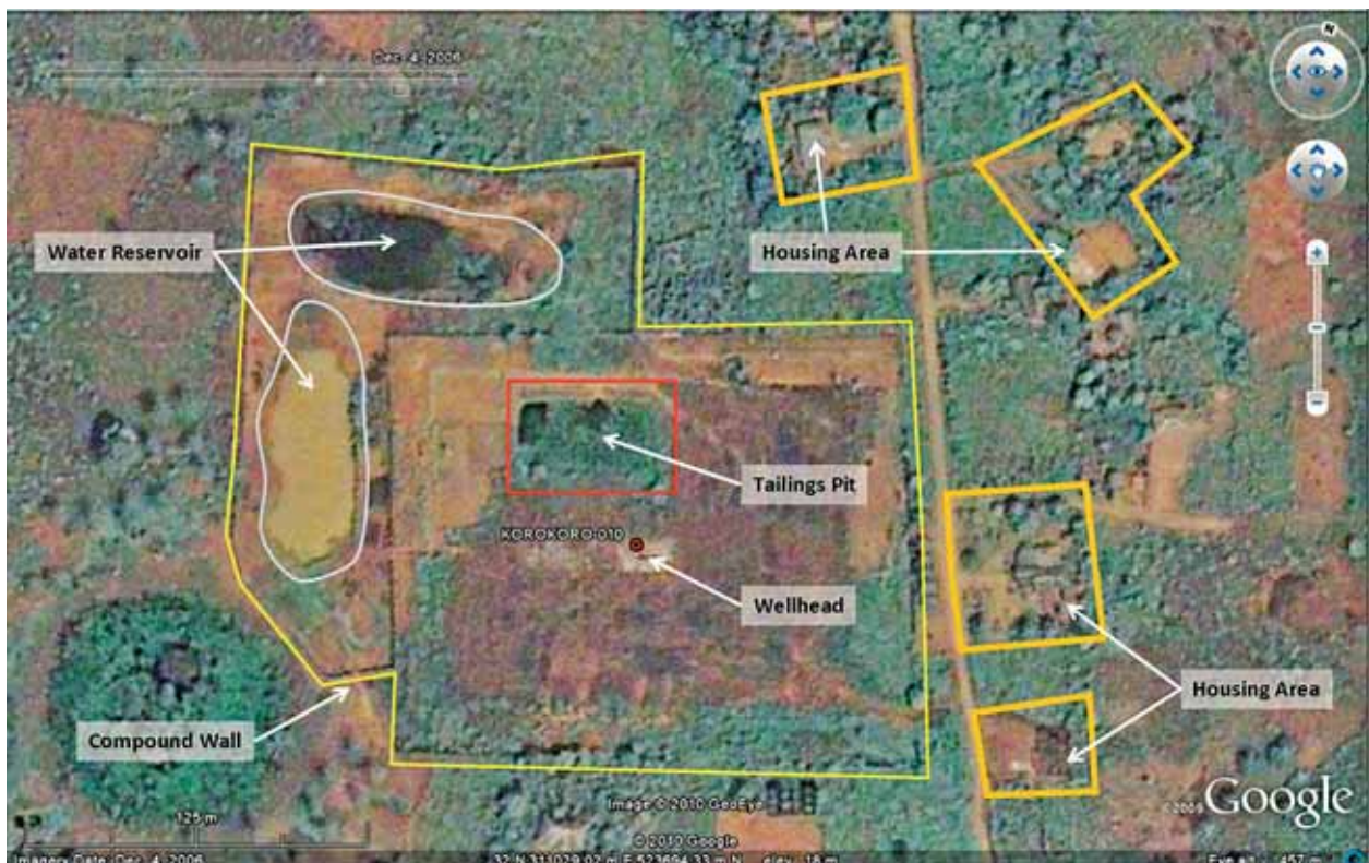
Typical well Infrastructure (009-002 Well Korokoro 10, Tai LGA)
