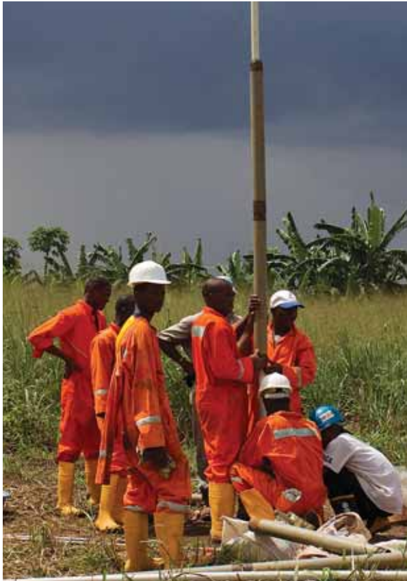
Fugro staff installing a groundwater monitoring well, April 2010
