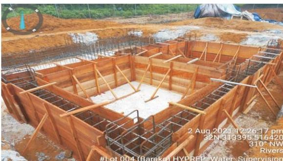
**Construction of Foundation for Overhead Tank at Barako Lot 4**
