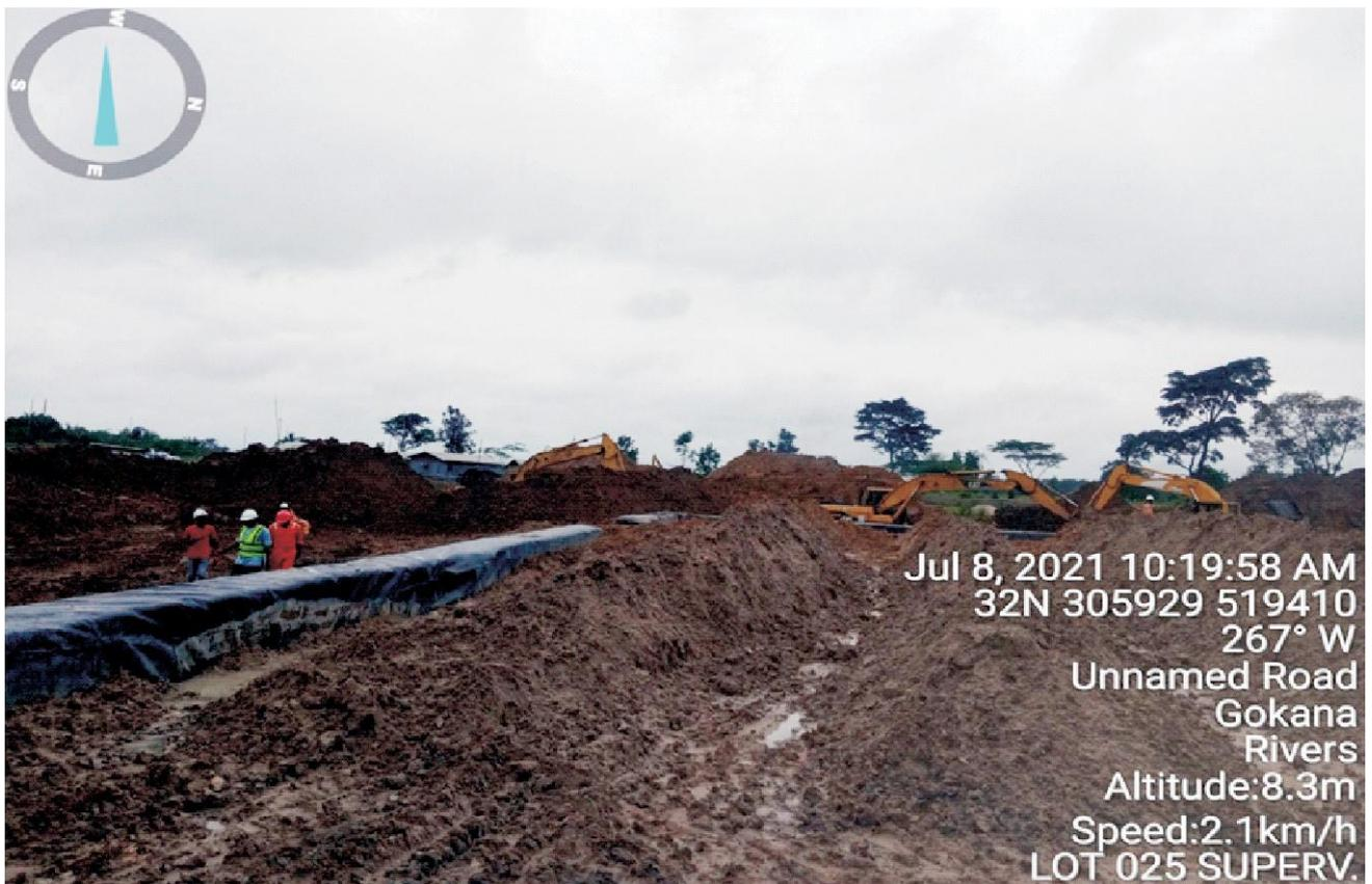
Plate 1.3: Excavation contaminated soil undergoing treatment in the Biocell (solid phase bioreactor cell) at Lot 025 (B. Dere / Gio, Gokana / Tai L.G.A). Remediation Contractor = *SUBADOM GLOBAL RESOURCES LTD*.
