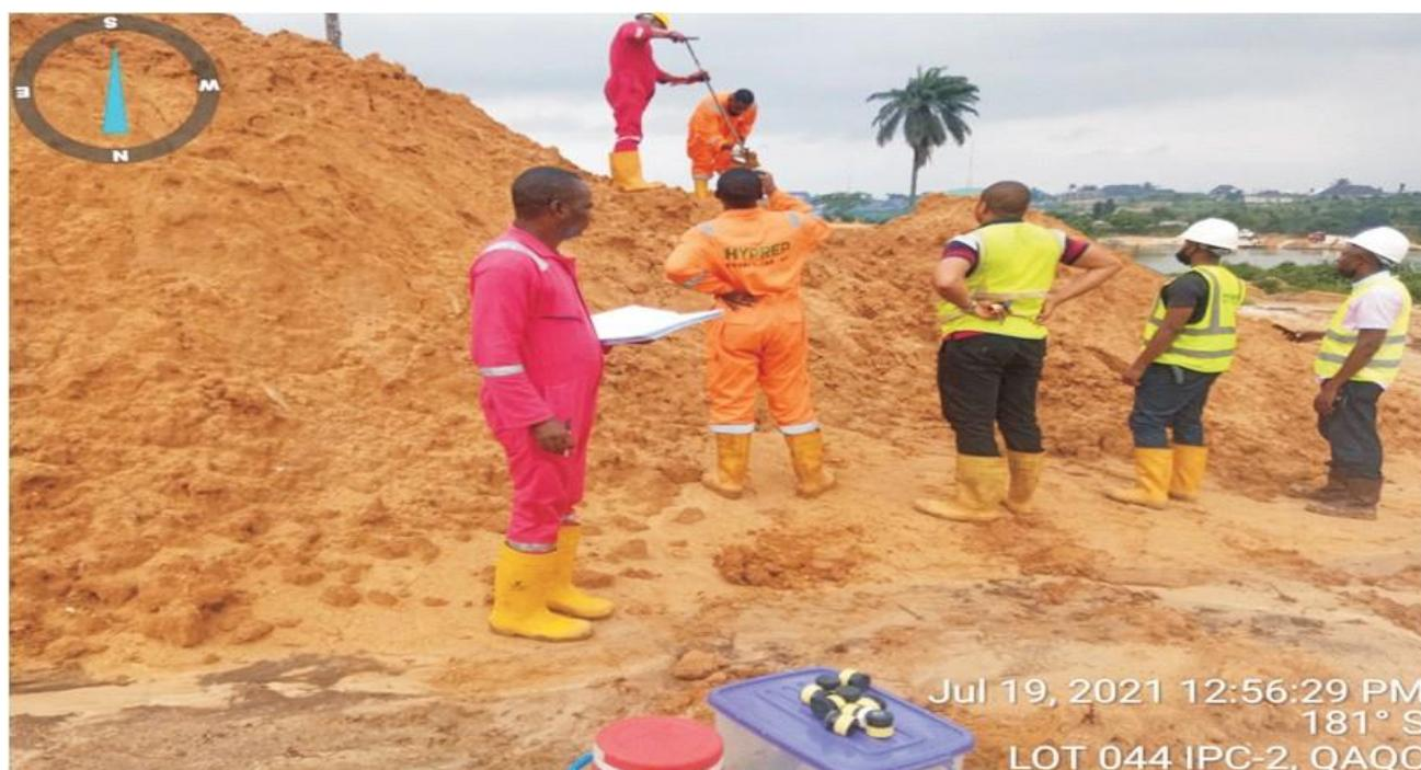
**Plate 1.3: Quality Assurance / Quality Control (QA/QC) and Remediation Execution Officers from the Operations Unit of HYPREP collecting QAQC Monitoring Samples from treated soil volumes with the Contractor representatives at Lot 044 (Aieto (Ngofa), Eleme L.G.A).
