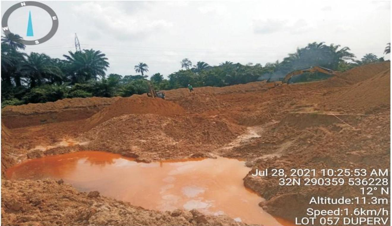
Plate 1.2: Excavation and serial transferring of impacted soil in progress at Lot 057 (New Elemenwa Manifold, Akpajo, Eleme L.G.A). (Remediation Contractor= *INTEGRATED CHEMICAL WORKS LTD*).
