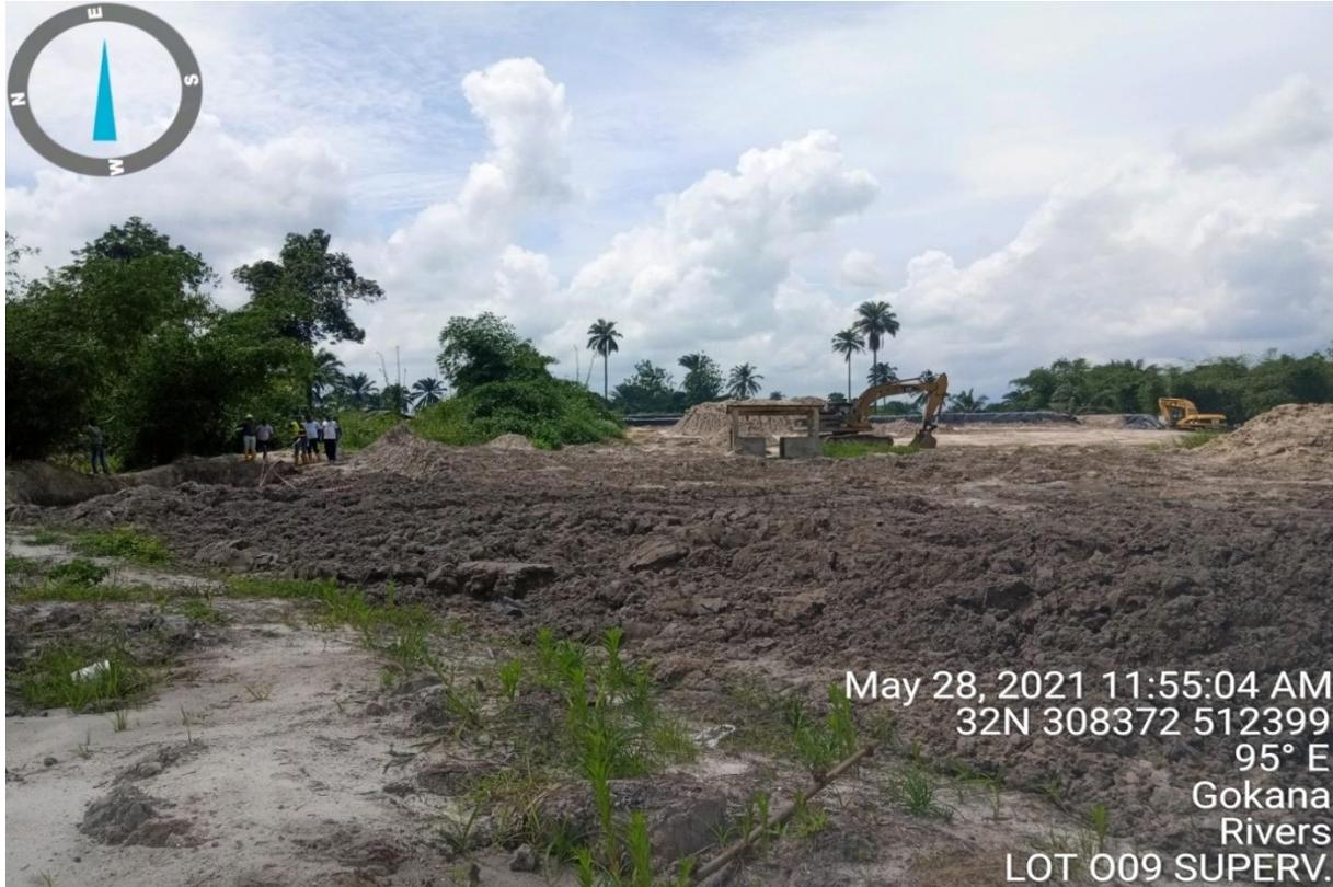
**Plate 1: Final stage of backfilling of excavated pit with treated soil at Lot 009 (Saanako) in Mogho, Gokana L.G.A. (Contractor: Odun Environmental Ltd).**
