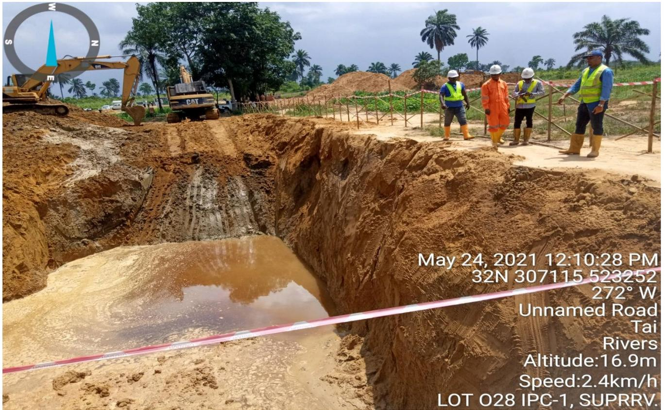
**Plate 3: Commencement of excavation of impacted soil from delineated impacted area for treatment at Lot 028 (Bara Alue in Tai L.G.A). (Remediation Contractor = Emamed Nig. Ltd).**
