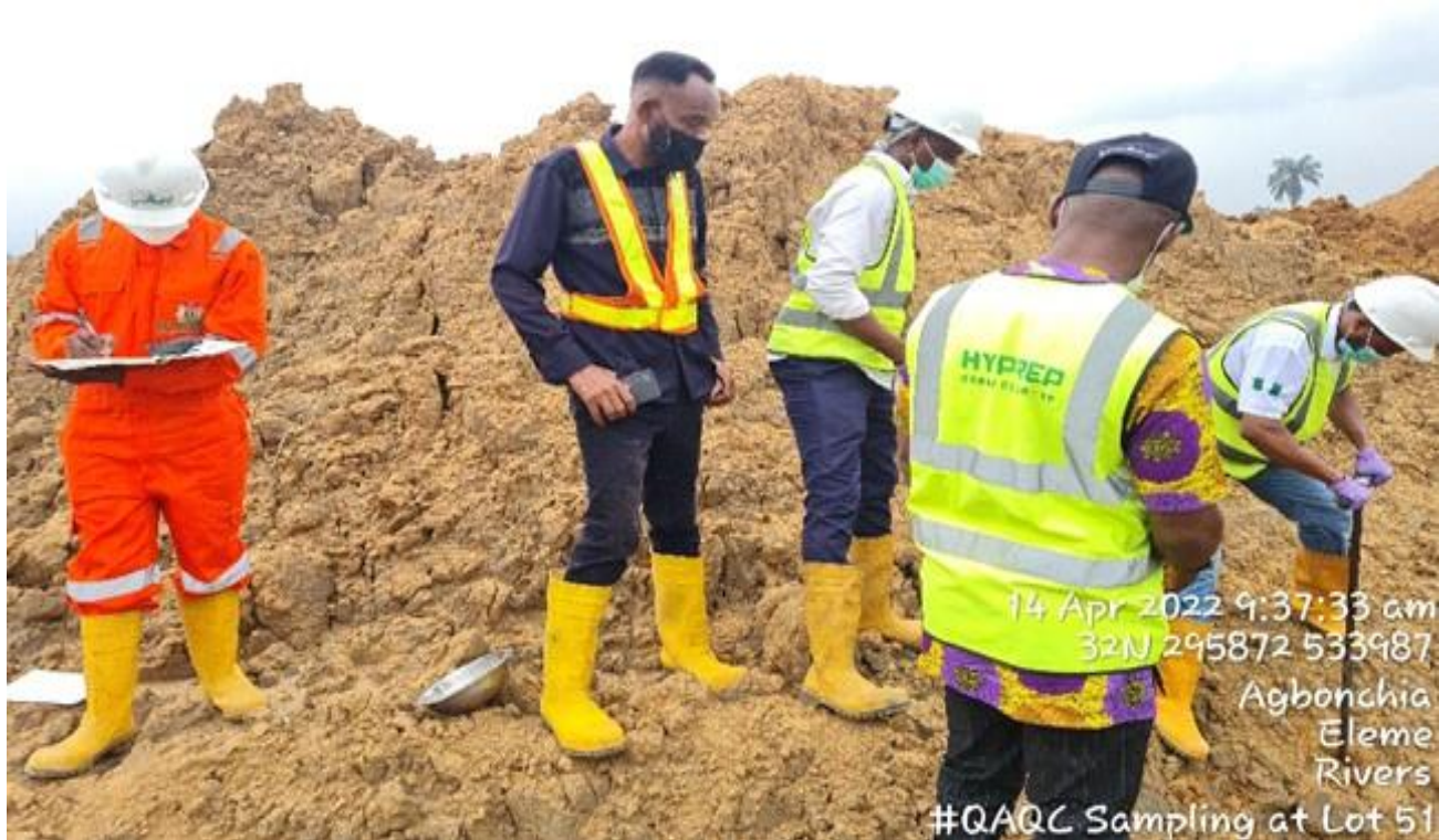
Personnel from the Operations Unit of HYPREP collecting QAQC Mid-Term Monitoring Samples from the base of an excavated pit at Lot 051: Okuluebu Ogale, Eleme L.G.A. Remediation Contractor - EROTINA NIGERIA LTD
