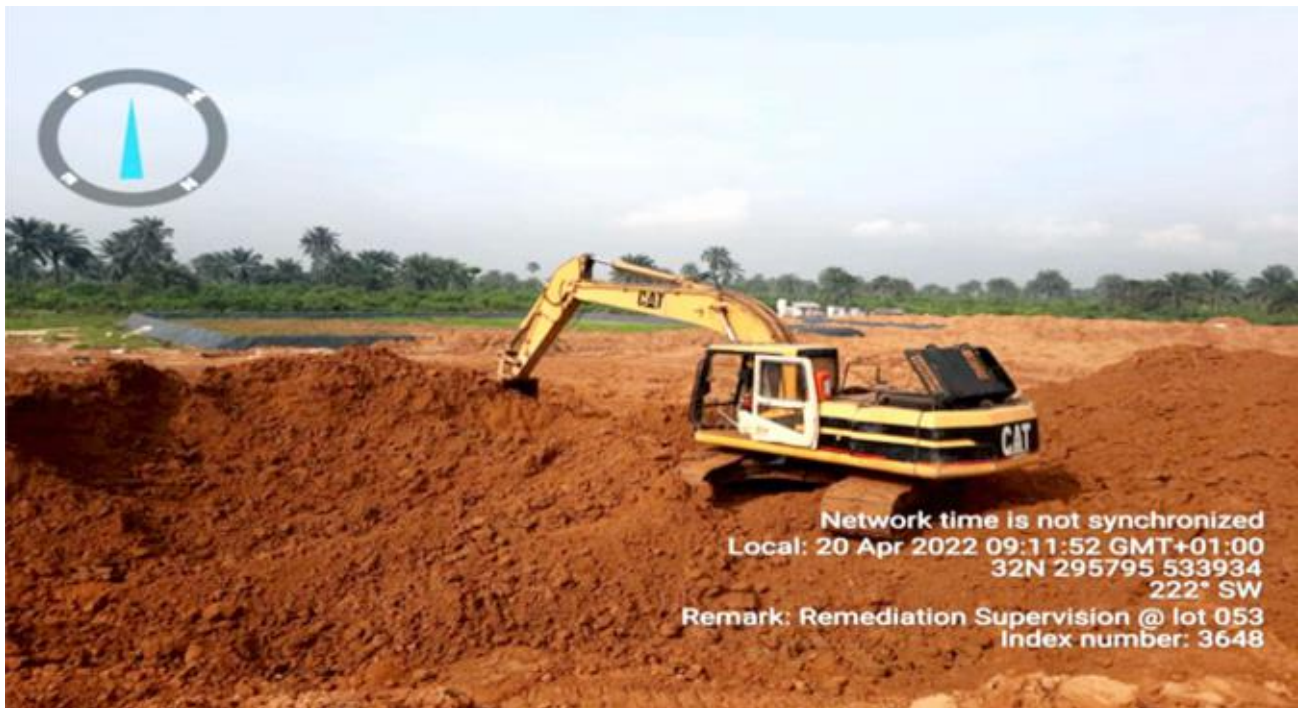
Plate 1.4: Transfer of Treated Soil from Storage Area to Excavated Pit for Backfilling at Lot 053 (Okuluebu Ajeokpori Well 3, Ogale, Eleme L.G.A) Remediation Contractor - ATLAS RAY AND SONS COY LTD.
