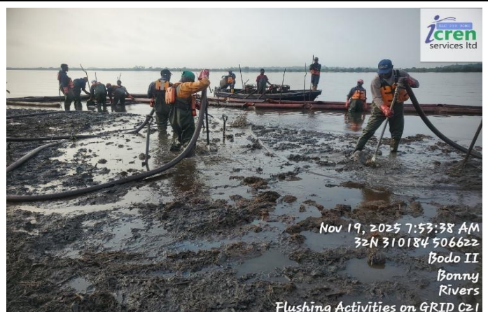
Plate 10: Sediment Flushing, K-Dere
