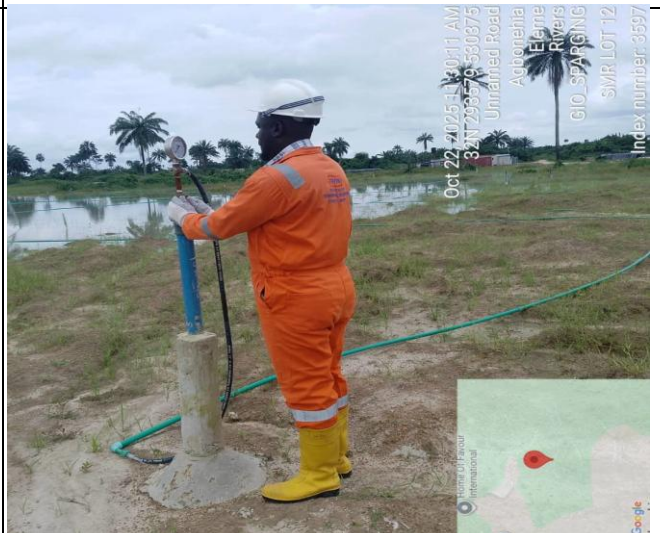
Plate 5: Biosparging Setup at SMR Lot 012
