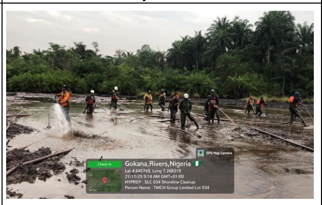
Plate 4: Sediment Flushing, Goi
