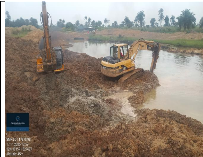
Plate 1: Excavation of impacted soil SMR Lot 017
