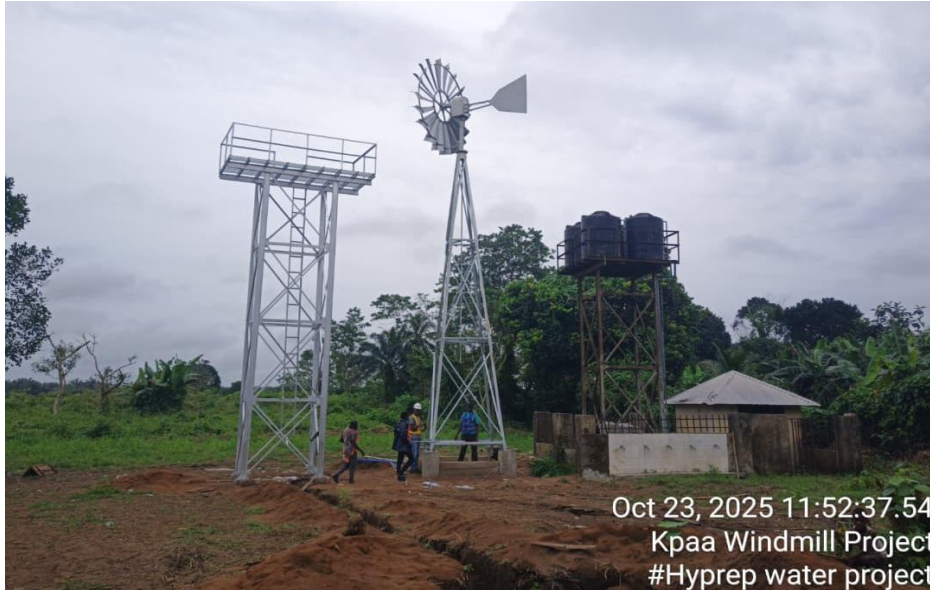
Windmill construction at Kpaa
