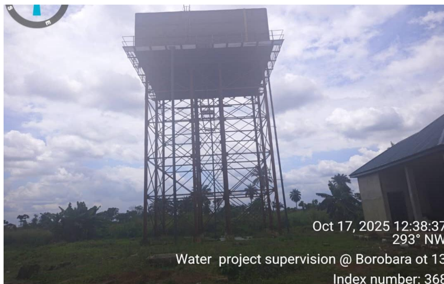
Elevated tank construction at Borobara
