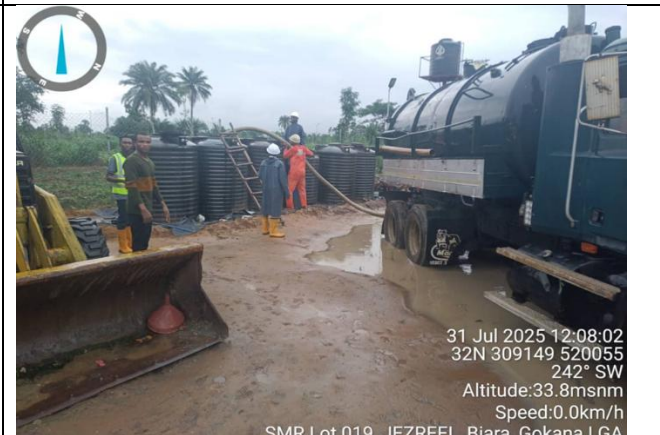
Plate 4: Evacuation of Recovered free-phase oil at SMR Lot 019
