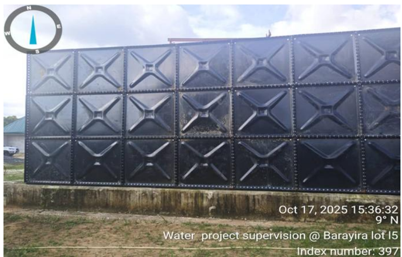
Ground tank construction at Barayira
