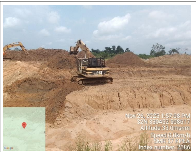
Plate 2: Excavation of Impacted Soil at SMR Lot 037
