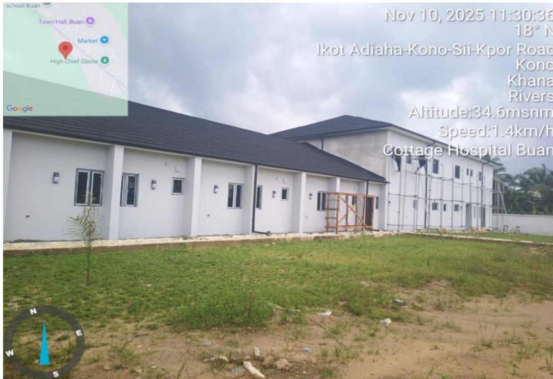
Painting Of Main Building External Walls/Scaffolding
