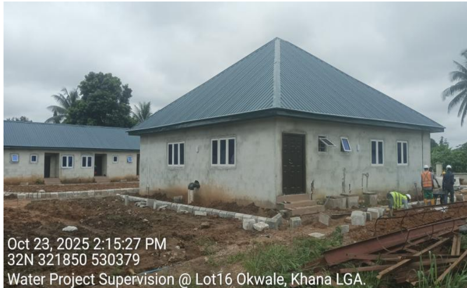
Laying of kerbs and general on-going, Okwale
