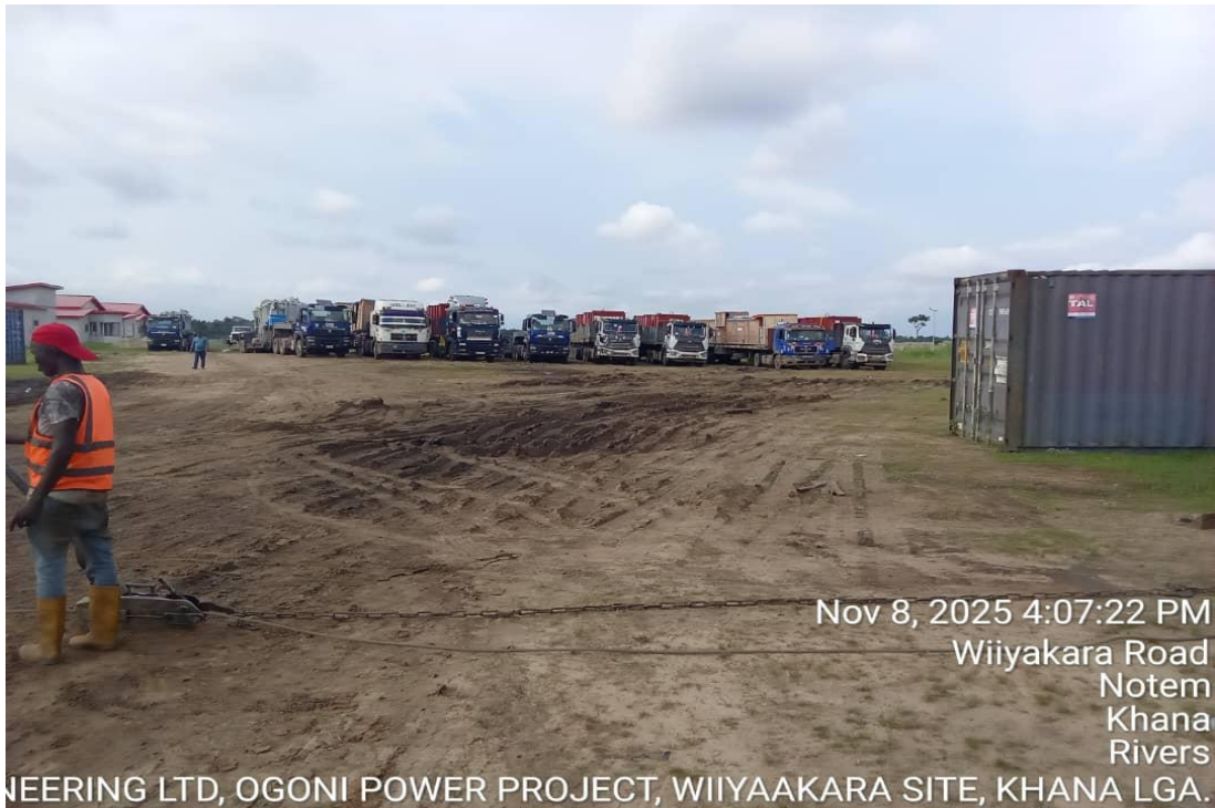
Figure 1: Truckloads of offshore equipment for Transmission Lines, Bodo and Wiyakara Substations.
