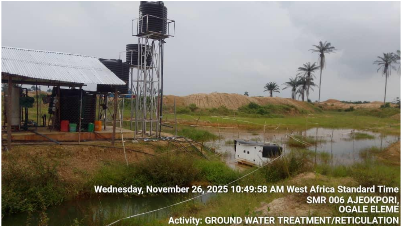
Plate 6: Pump and Treat Setup at Lot SMR 006
