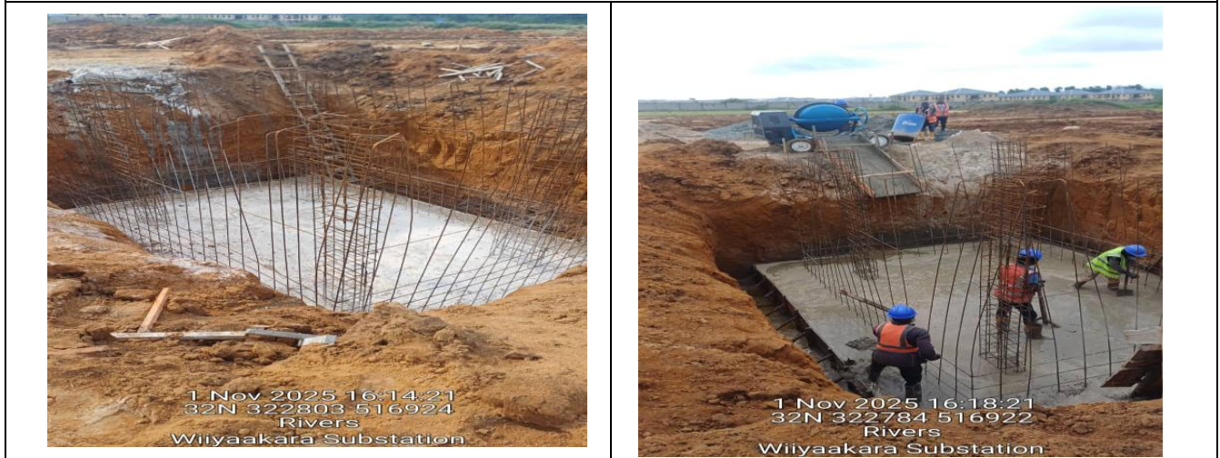
Fig. 2: Preparation of 132kv gantry bases at Wiyakara substations
