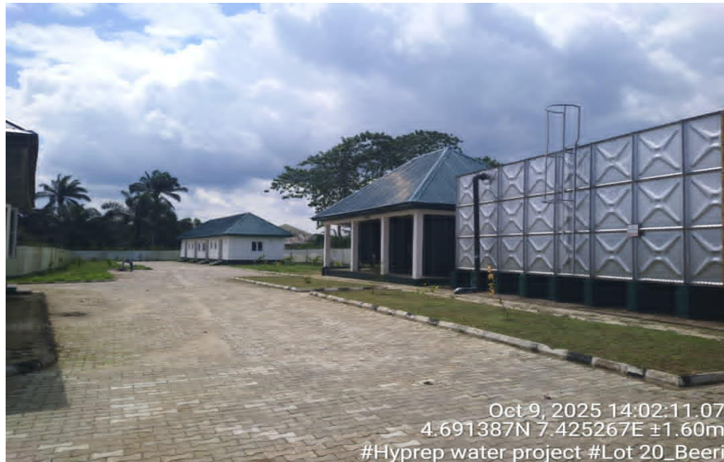
Operational maintenance at Beeri station
