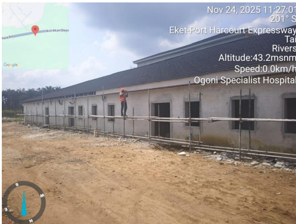
Roofing Annex Building and Scaffolding on Main Building
