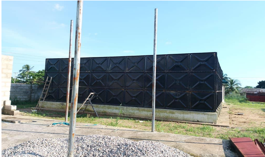
Ground tank construction at Botem, Tai LGA.
