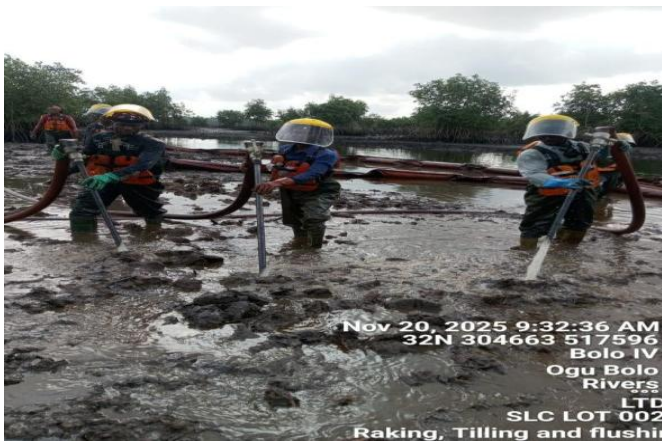
Plate 7: Sediment Flushing, B-Dere
