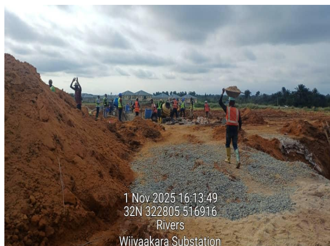
Fig. 3: Construction activities in Wiyakara substations
