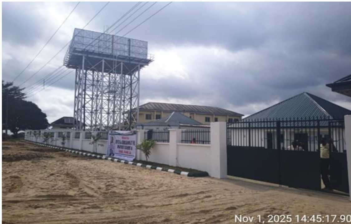
Bane Station getting set for commissioning
