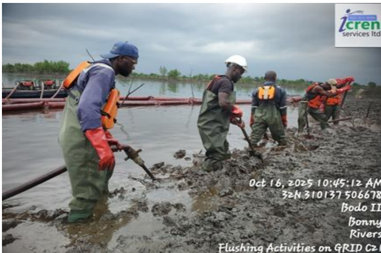
Plate 11: Sediment Flushing, Bomu
