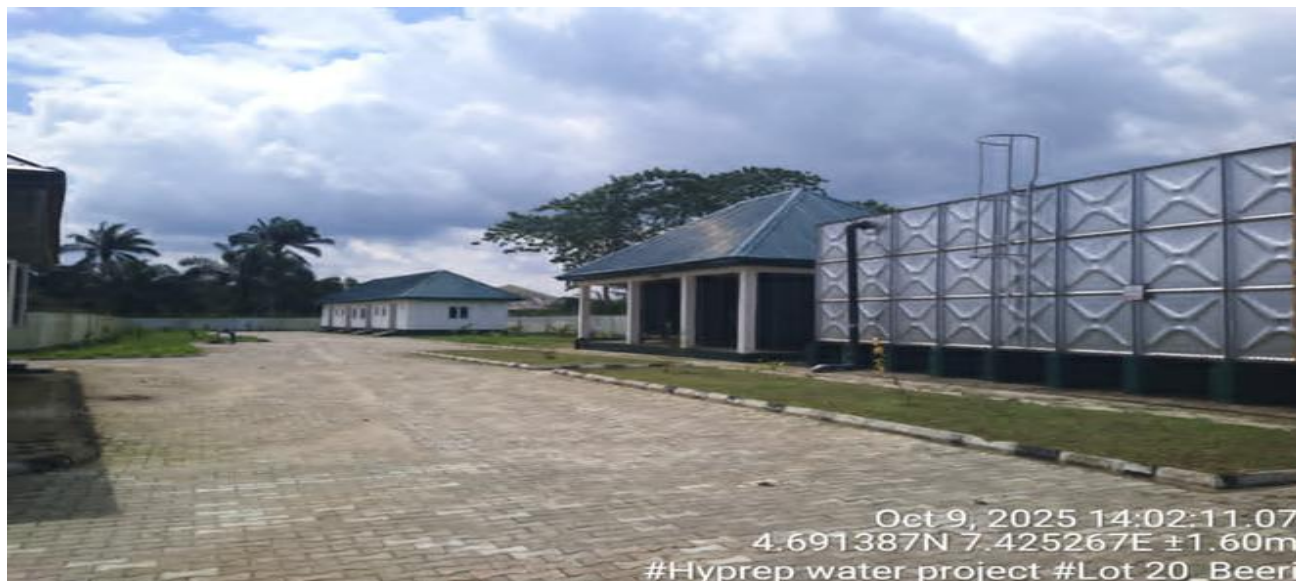
Operational maintenance at Beeri station.
