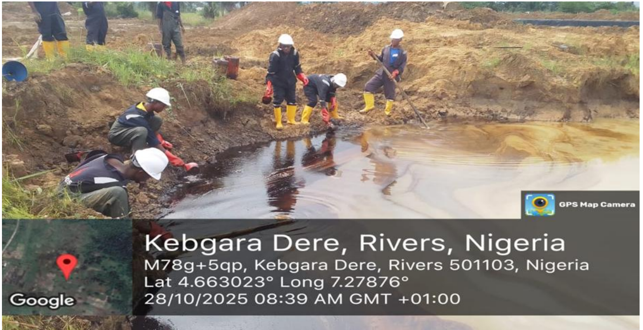
Plate 3: Recovery of Free-Phase Products at SMR Lot 016B
