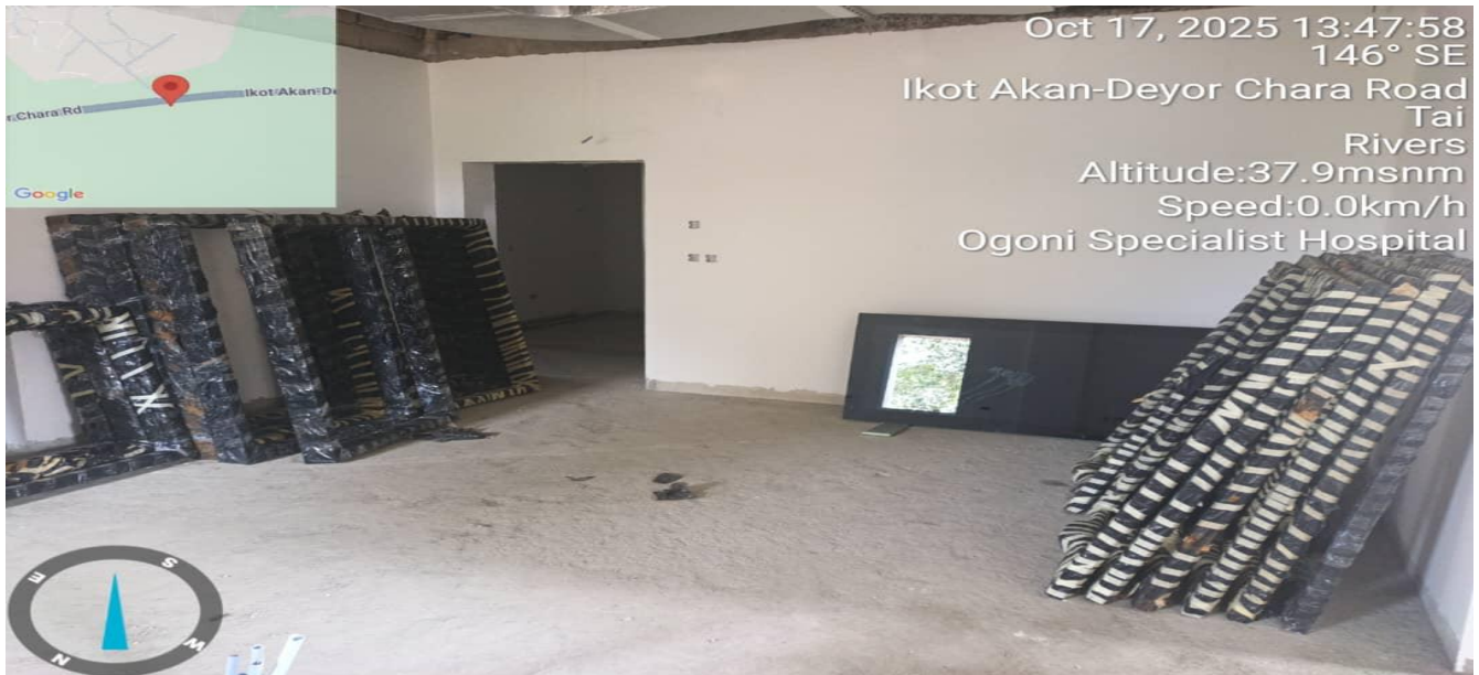
WINDOW FRAMES AND GLASS BEFORE INSTALLATION
