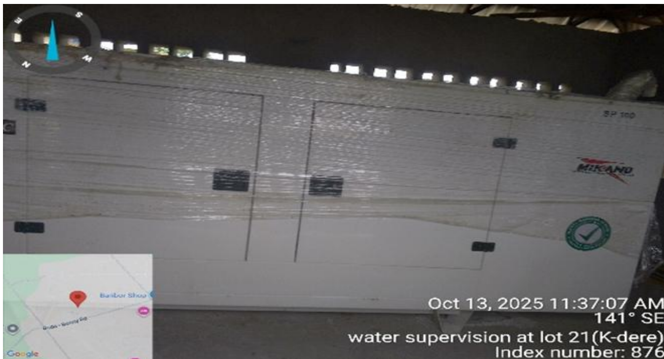
100KVA generator installation at K-Dere site
