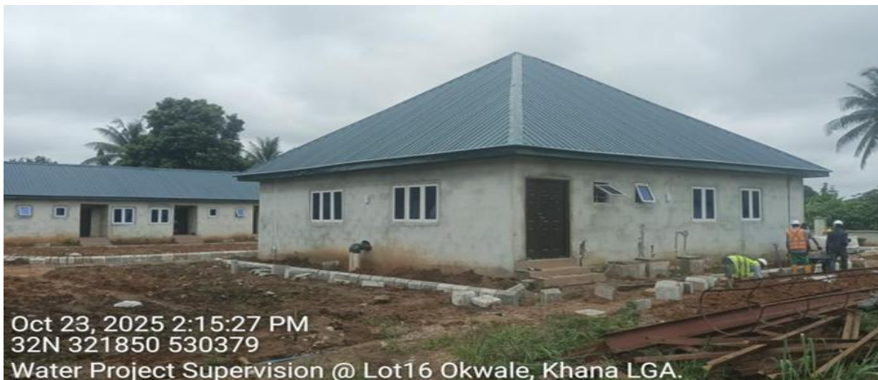
Laying of kerbs and general on-going, Okwale.
