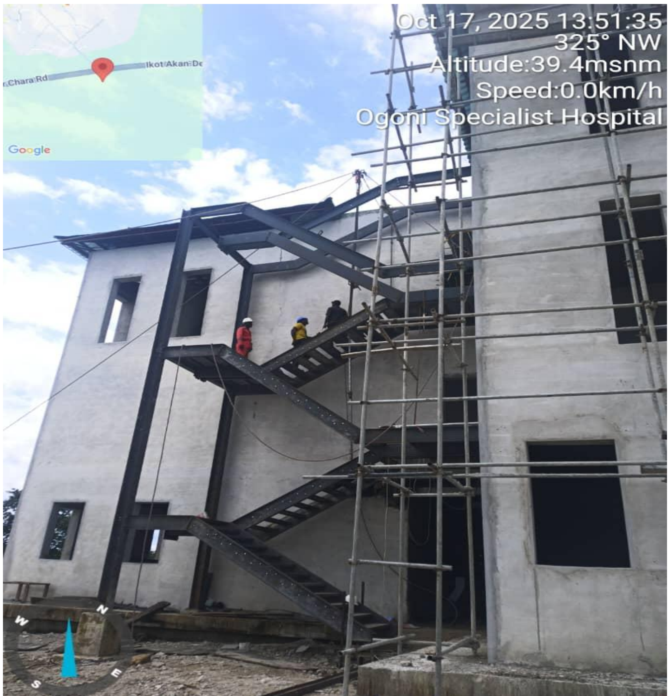
Figure 4.1: Construction of Ogoni Specialist Hospital: Fabrication and Installation of Staircase
