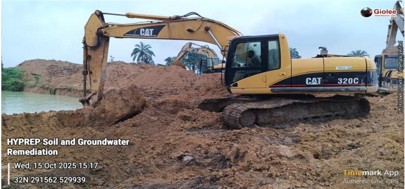
Plate 2: Excavation of Impacted Soil at SMR Lot 010
