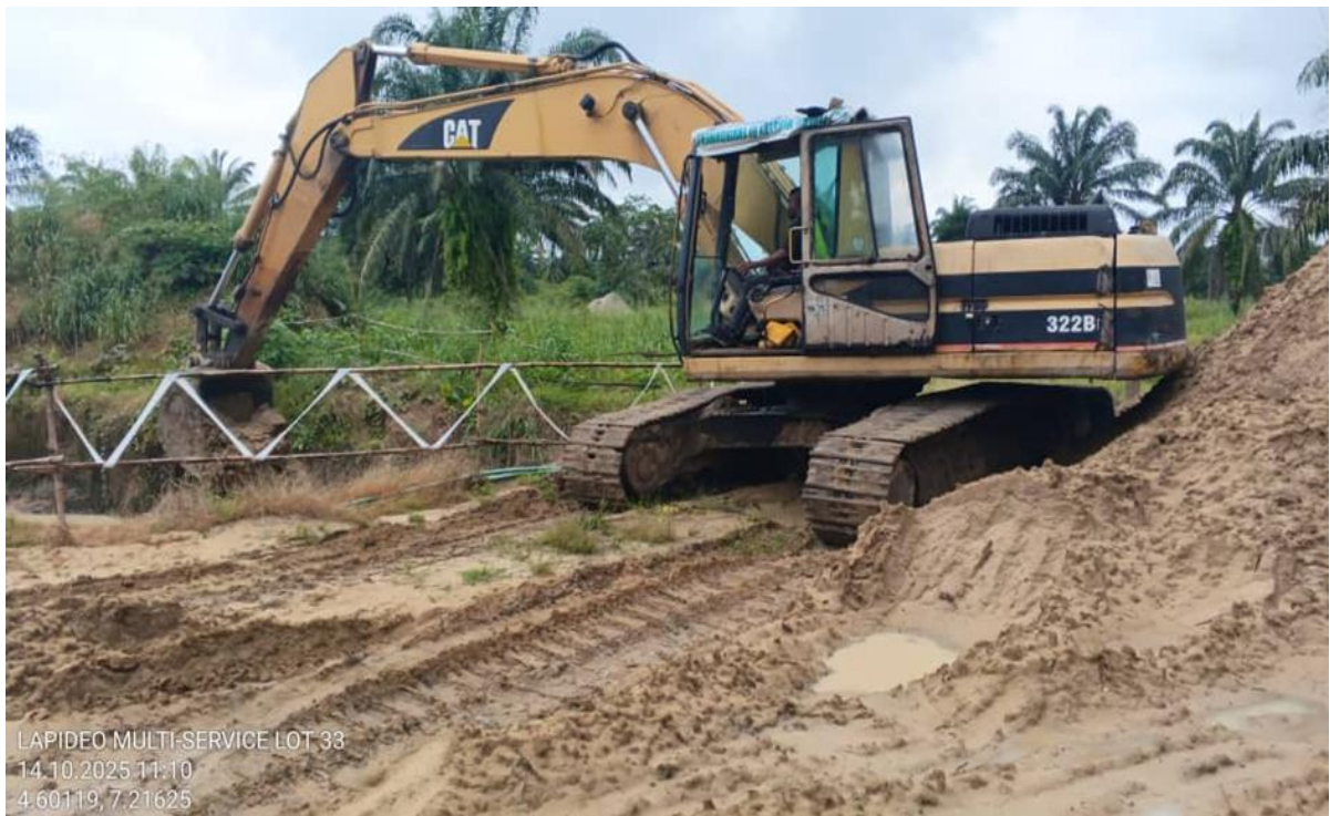
Plate 6: Backfilling of Treated Soil at SMR Lot 033
