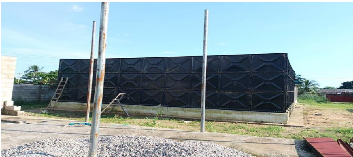
Ground tank construction at Botem, Tai LGA.
