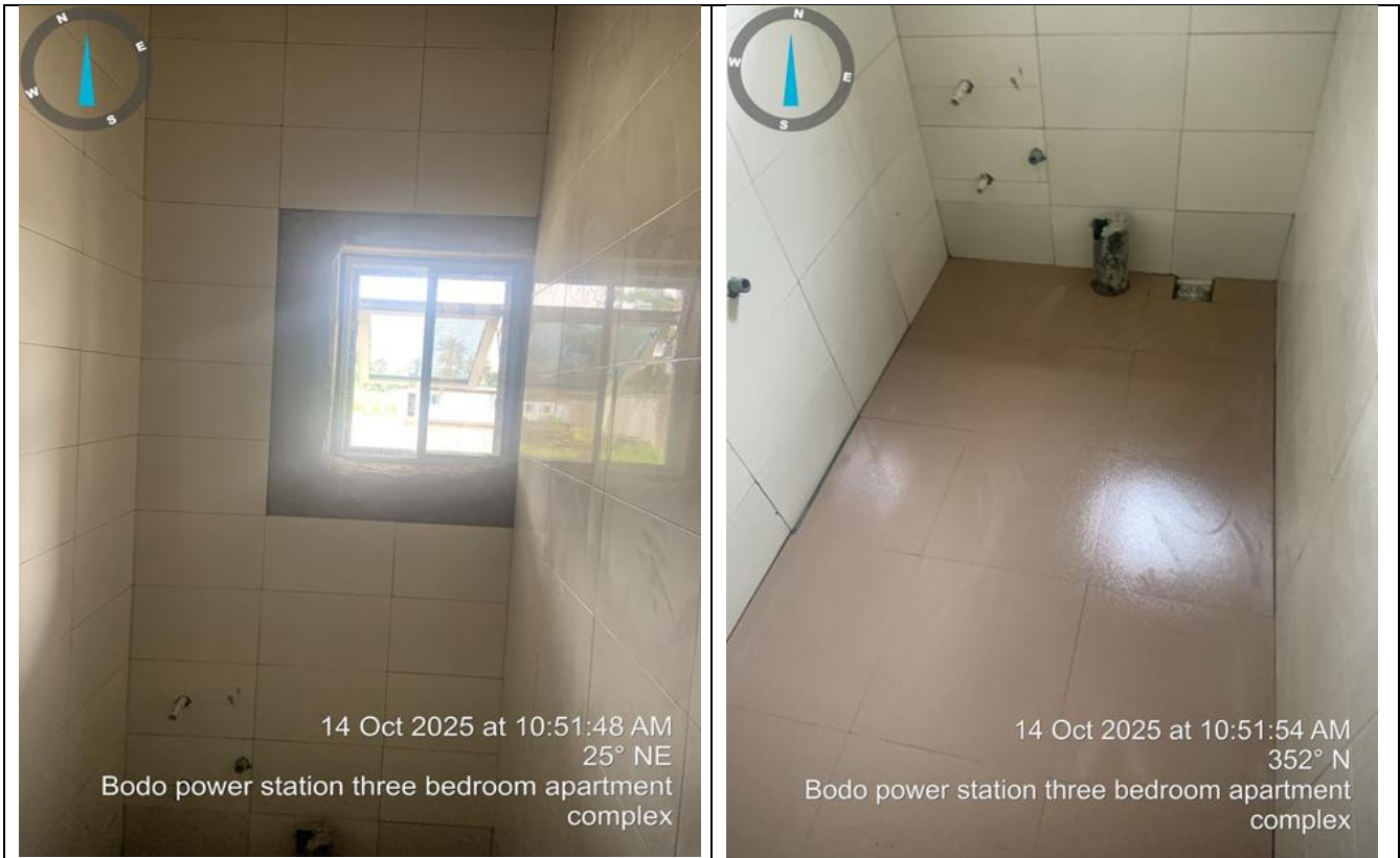
Figure 1: Bodo (Gokana LGA) Substation Staff Quarters Toilet Tiling
