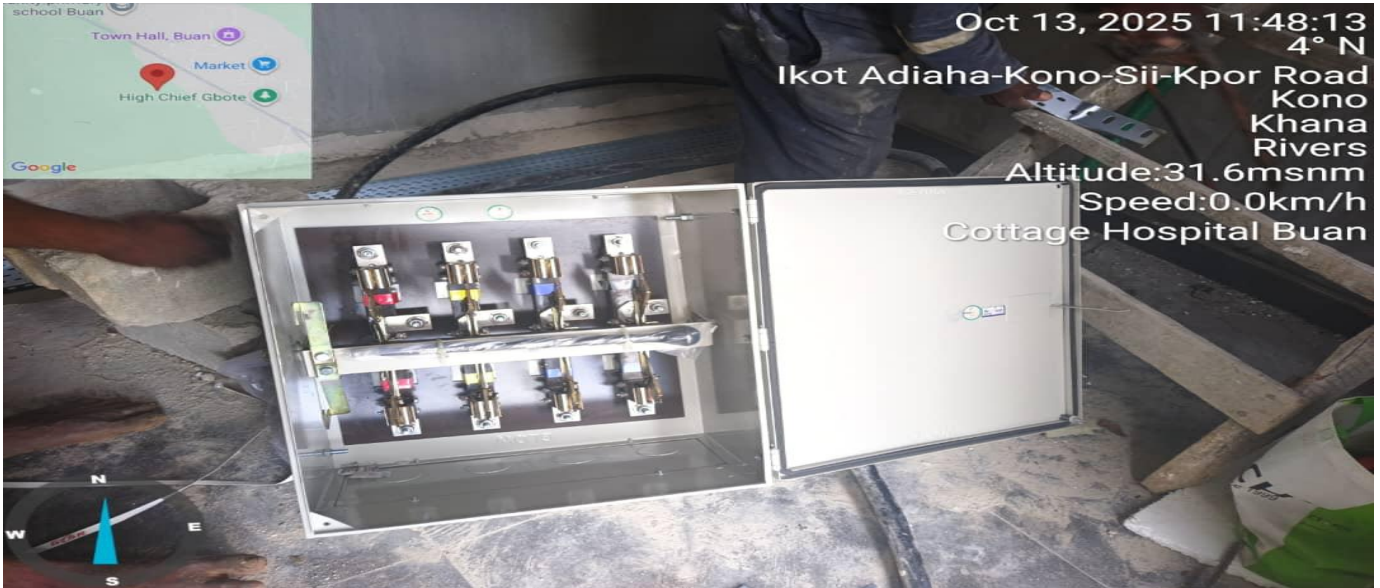
CHANGE OVER SWITCH INSTALLATION
