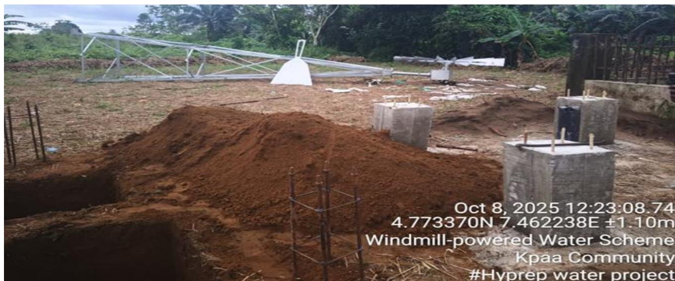
Windmill construction at Kpaa
