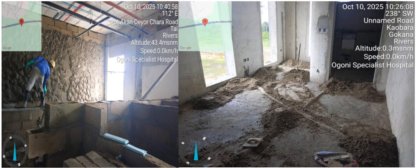
BLOCKWORK FOR REST ROOM ON GROUND FLOOR
