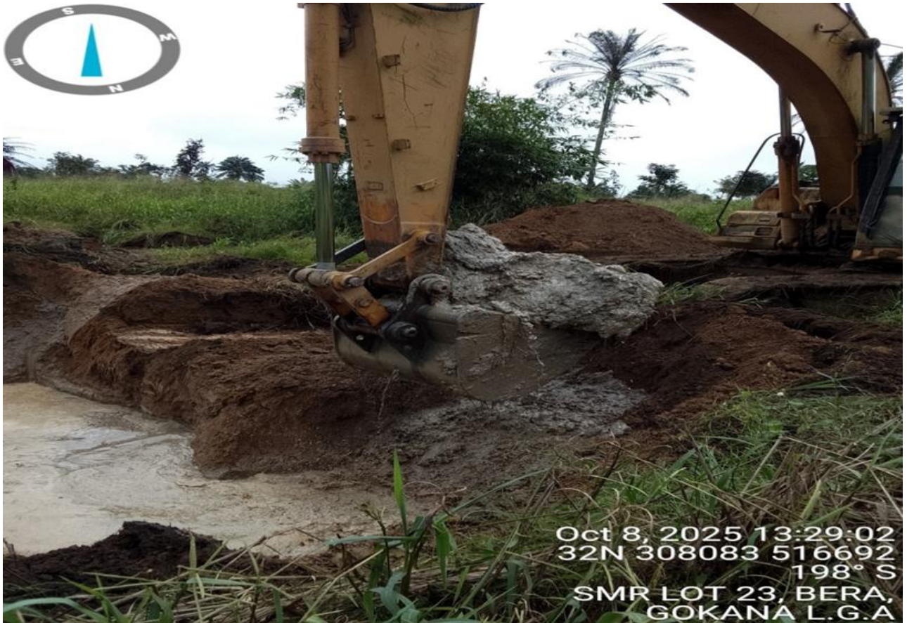
Plate 1: Excavation of impacted soil @ SMR Lot 033
