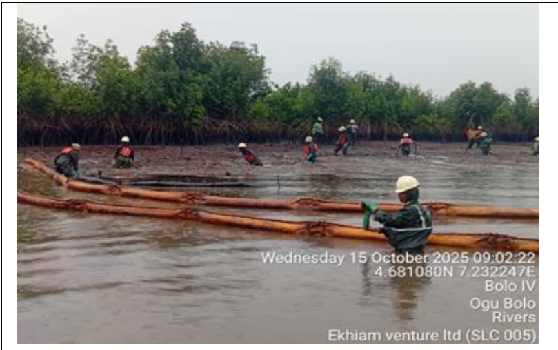
Plate 1: Sediment Flushing, B-Dere
