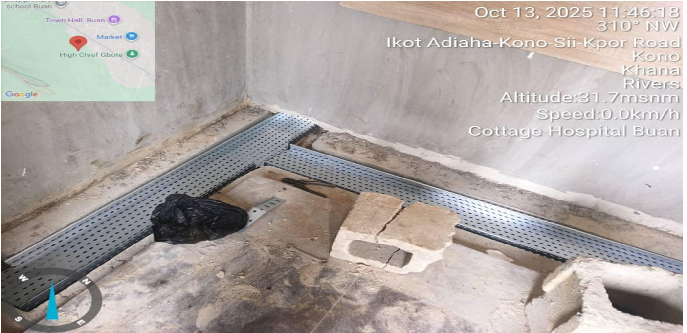
CABLE TRAY AT GENERATOR HOUSE INSTALLATION
