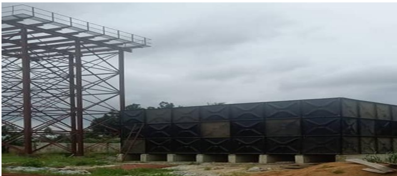
Elevated and ground tank construction at Deeyor
