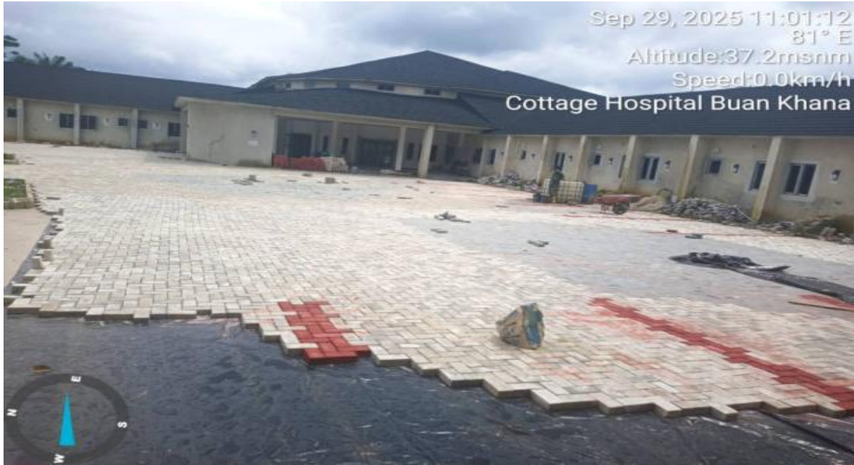
Laying of Interlocking Stone
