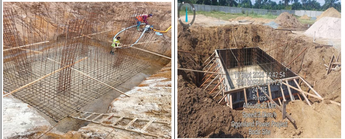
Figure 3: Preparation of gantry base at Bodo substation (Gokana LGA)
