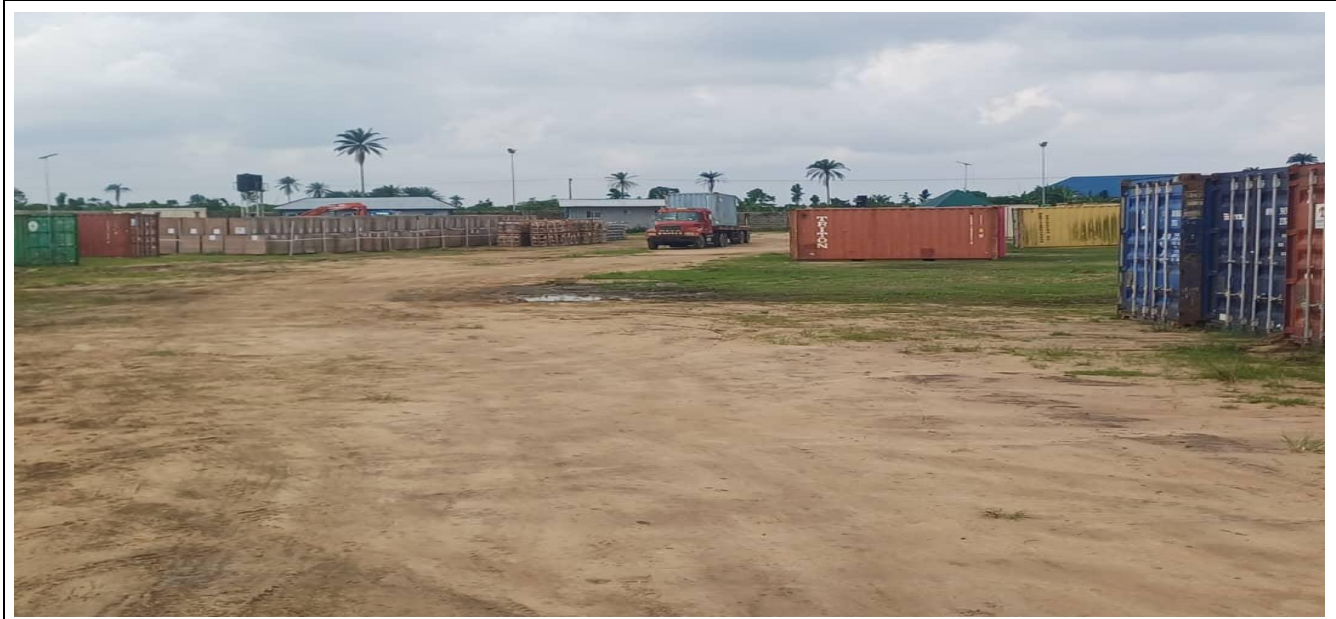
Figure 2: Offshore components of the Power Equipment at Wiiyaakara (Khana LGA) Substation
