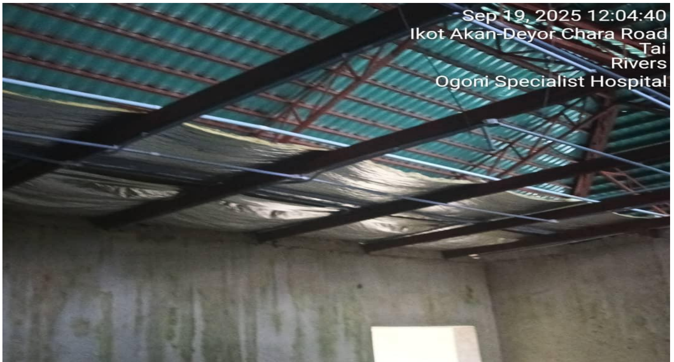
Installation of Rock Wool Installation
