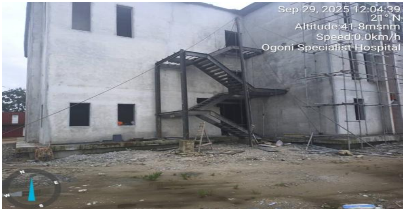
Installation of Staircase
