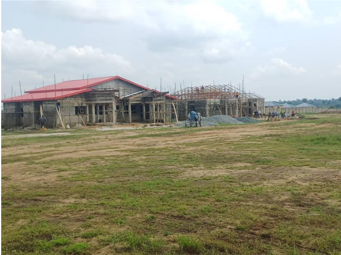
Fig. 4: Construction of staff quarters at Wiyakara substation
