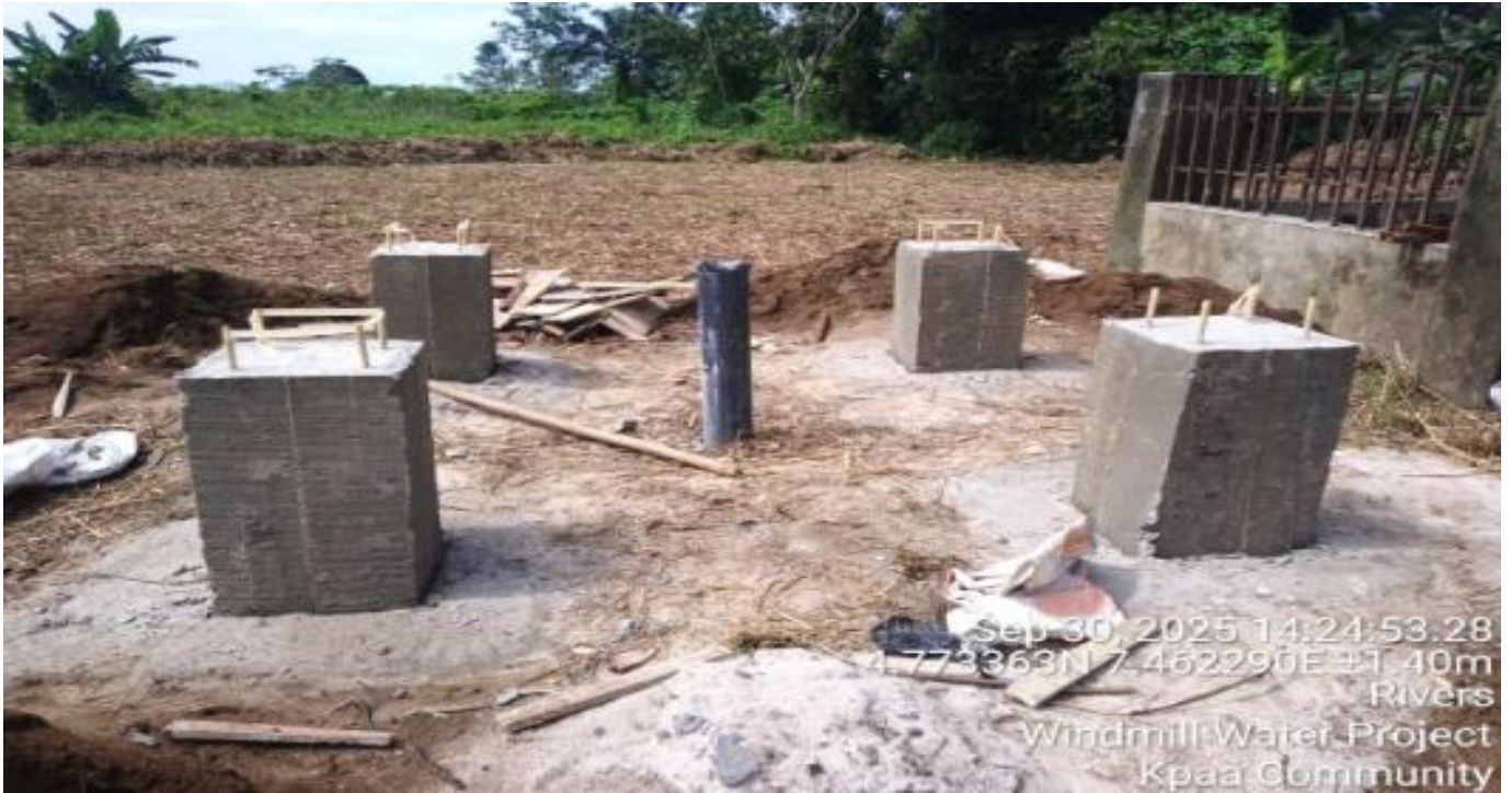
Foundation base construction at Kpaá
