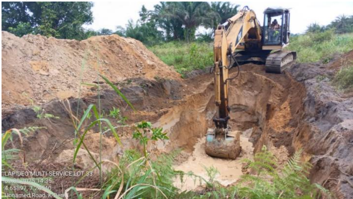
Plate 1: Excavation of impacted soil @ SMR Lot 033
