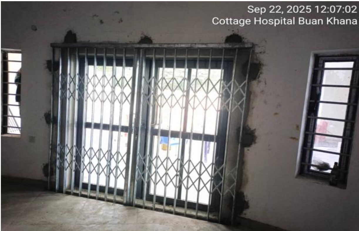
Installation of Burglary Proof at The Entrance Door
