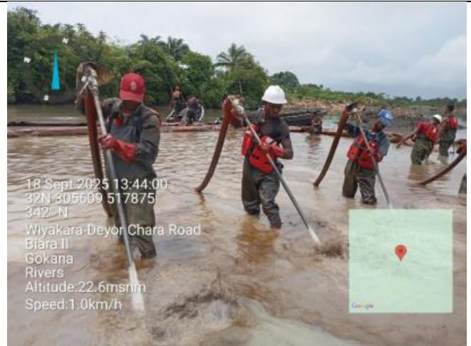
Plate 2: Sediment Flushing, B-Dere
