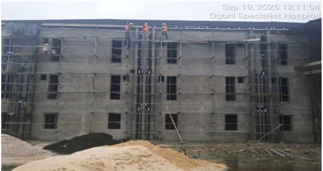
Installation of Fascia Soffit
