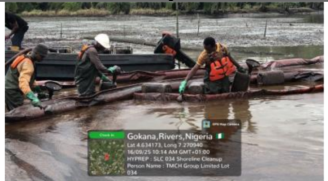
Plate 2: Sediment Flushing, B-Dere
