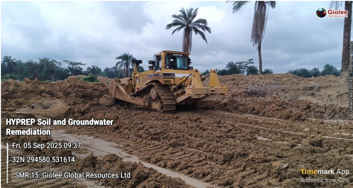
Plate 3: Backfilling of Treated Soil at SMR Lot 015
