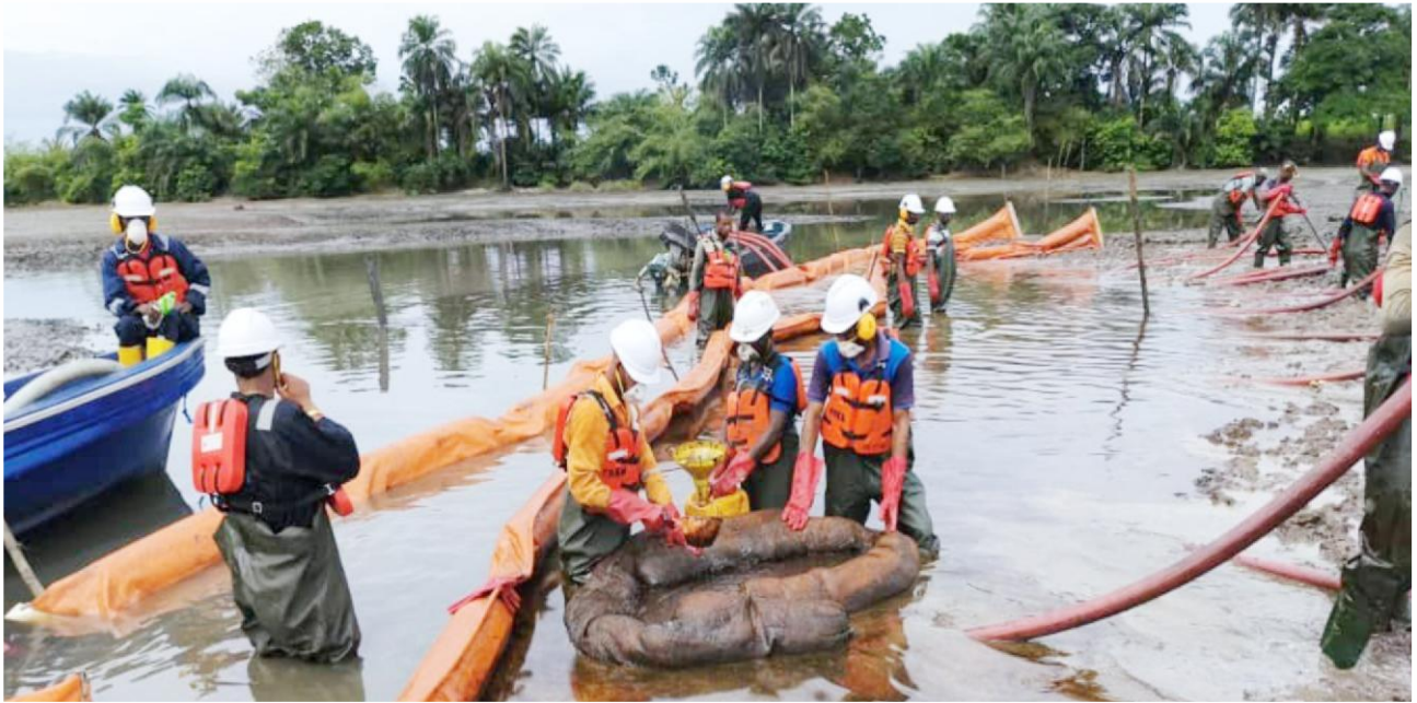
Sediment flushing, Booming and Oil Recovery
