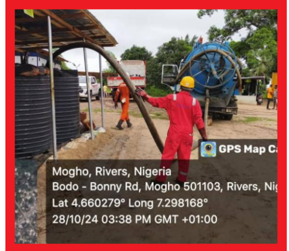
Evacuation of Recovered Oily Sludge for Treatment
