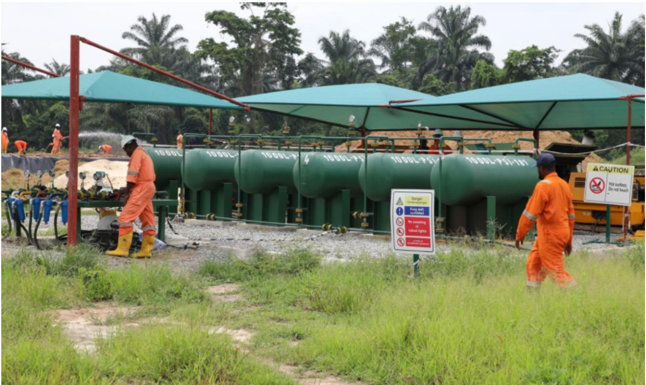
Land Remediation of Medium-Risk, Complex Site Using Biosparging Technology
