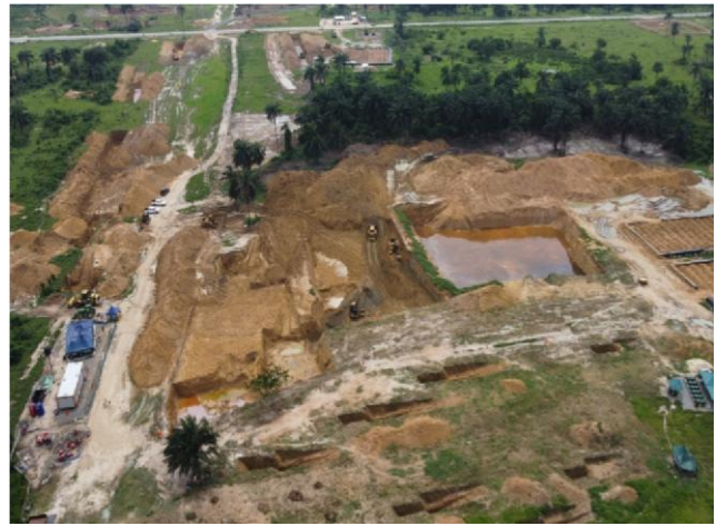
Aerial view of an active remediation site at Ogale, Eleme
