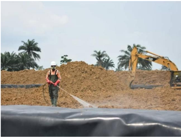
Soil treatment process in an engineered biocell
