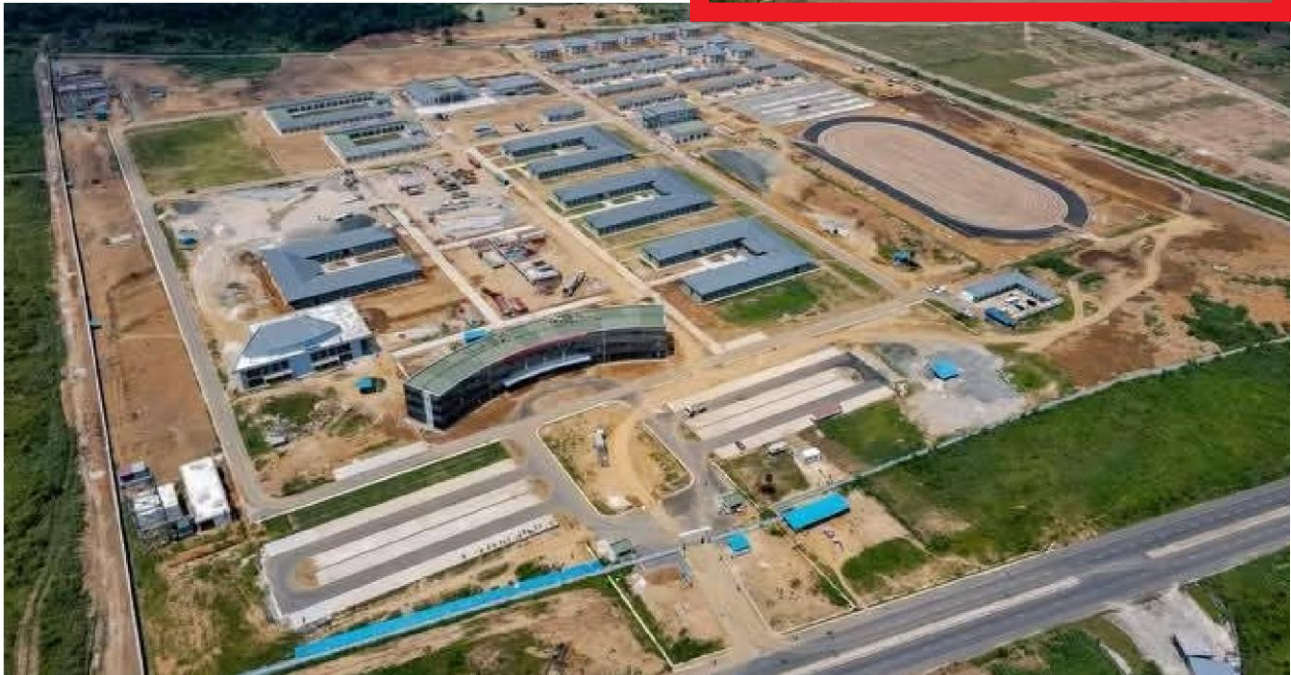
Aerial View of Centre of Excellence for Environmental Restoration under Construction
