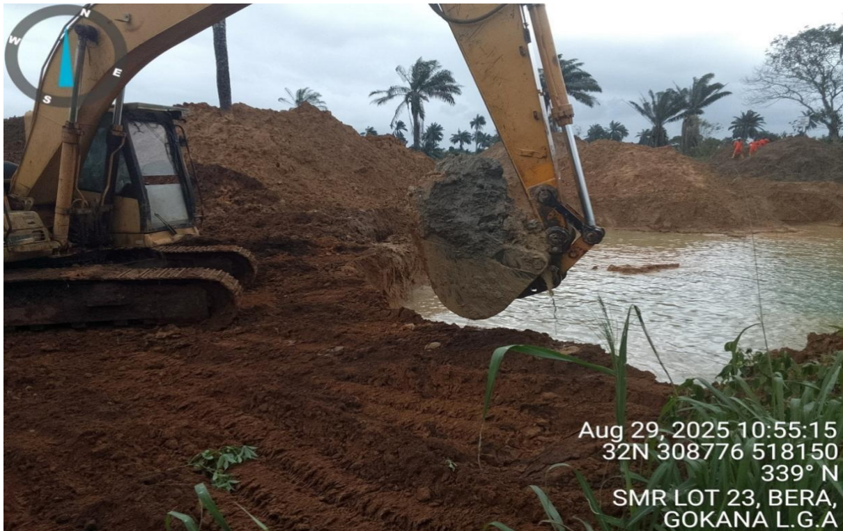
Plate 1: Excavation of impacted soil @ SMR Lot 023
