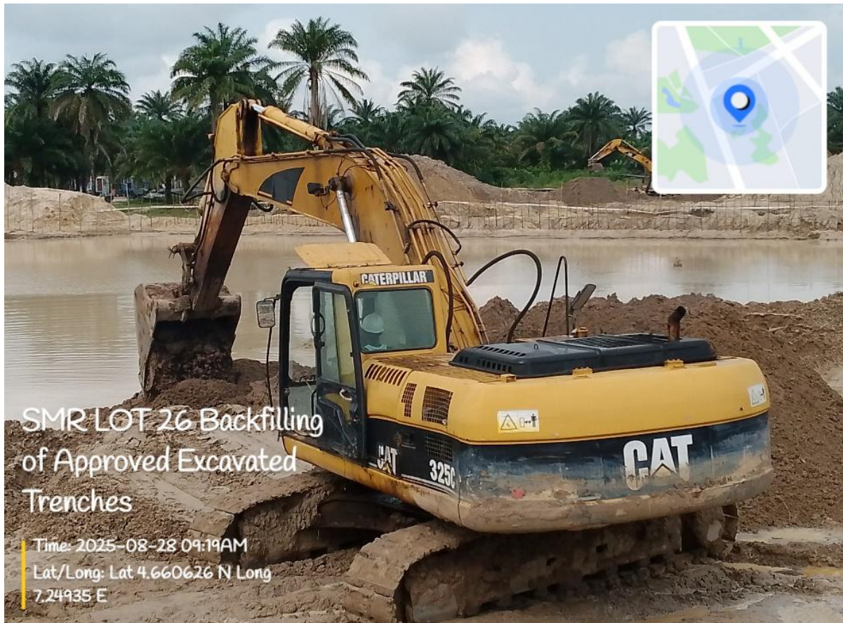
Plate 3: Backfilling of Treated Soil at SMR Lot 026
