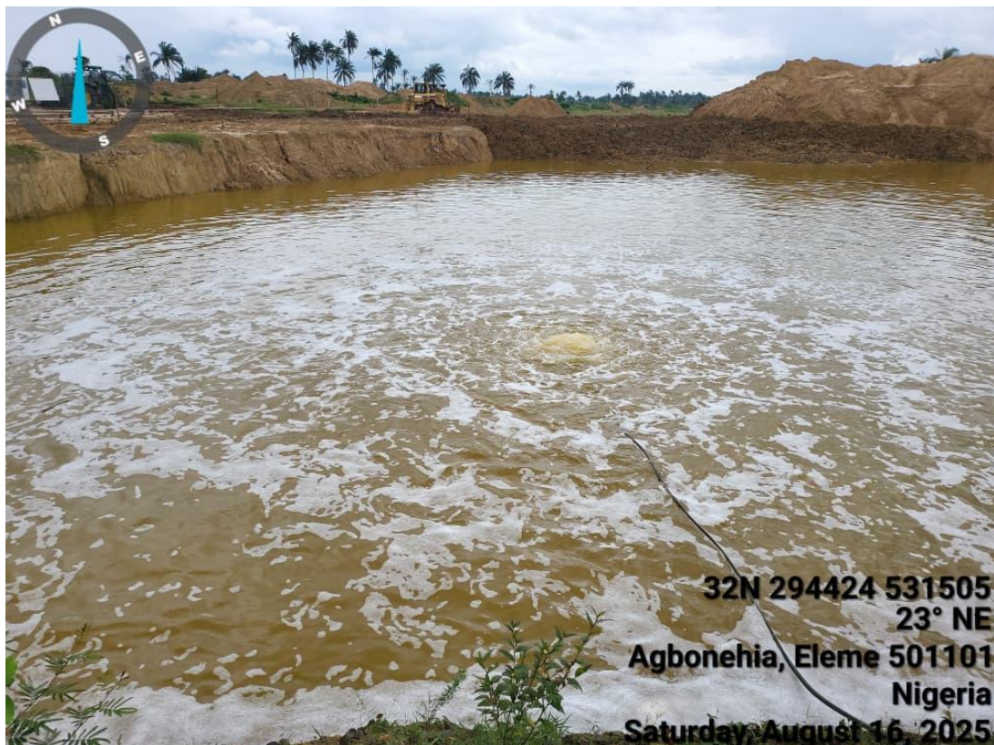
Plate 6: Biosparging of accumulated water in the Excavated Pit at Lot SMR 015
