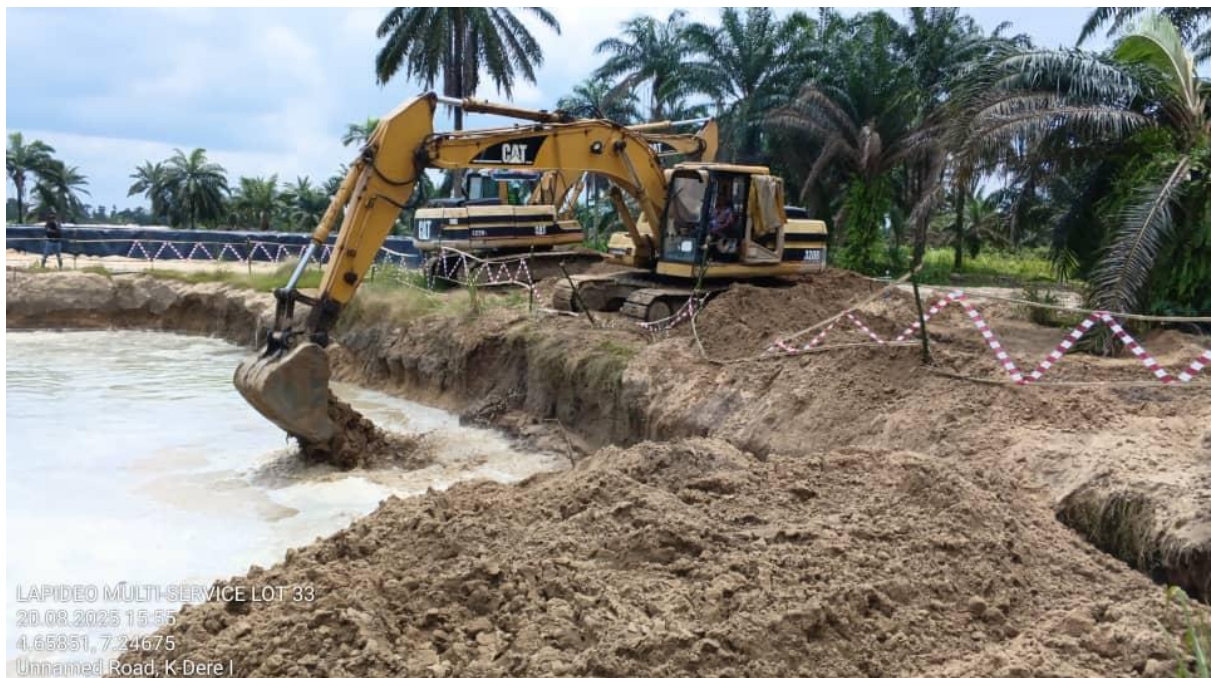
Plate 2: Excavation of Impacted Soil at SMR Lot 033
