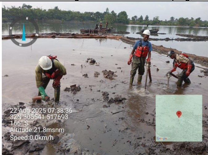
Plate 5: Booming and Manual oil Scooping, K-Dere
