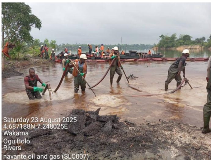
Plate 11: Sediment Flushing, B-Dere
