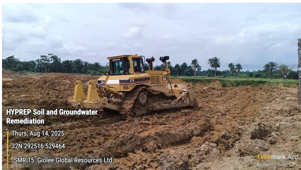
Plate 4: Backfilling of operations of Treated soil at SMR Lot 015
